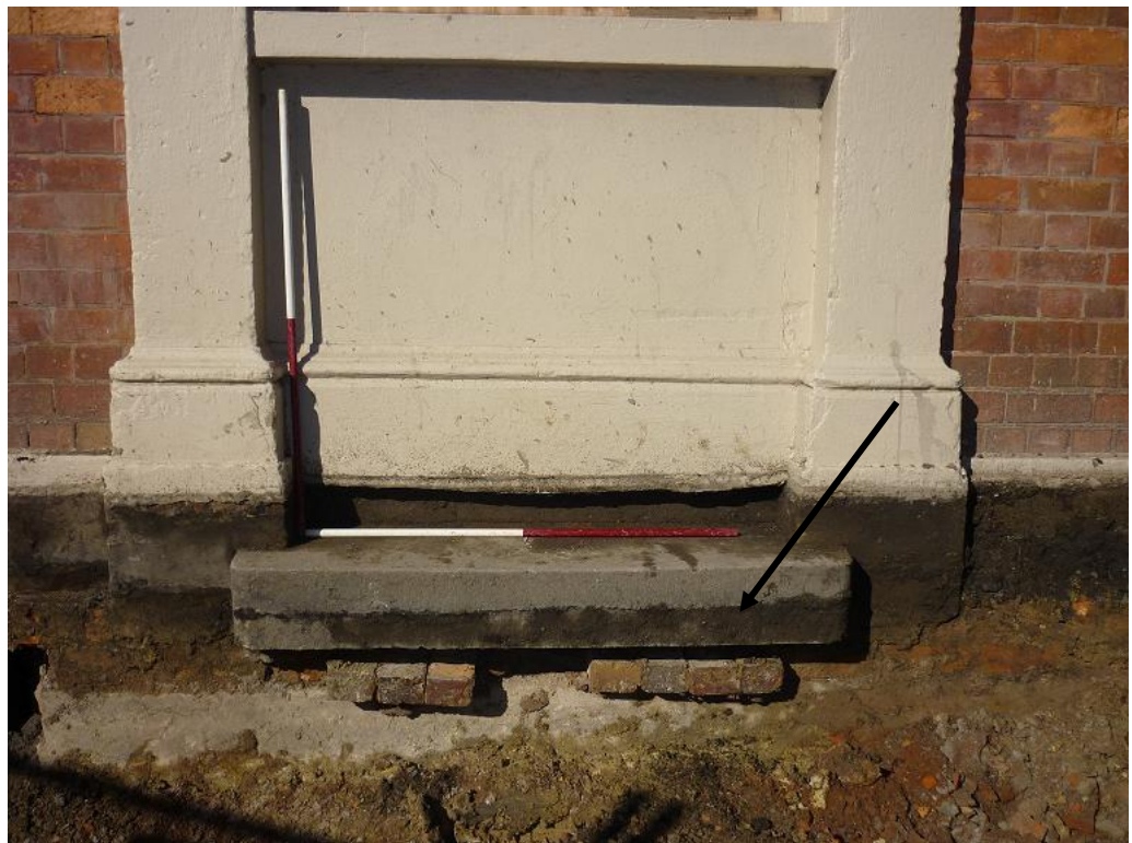
Figure 52. The original ground surface was at the base of the step. This is the original step of the west door that was later converted to a window. Facing east (1m scale)
