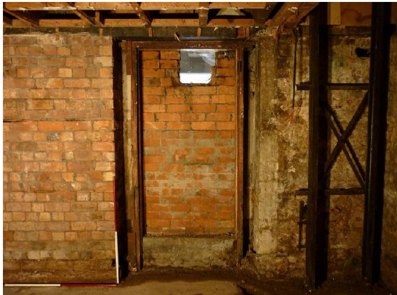
Figure 32. Doorway from the storeroom (here blocked off) which would have accessed the yard. The steel frame to the right is the modern hydraulic lift. Facing east. (1m scales shown)
