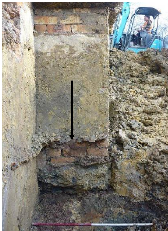
Figure 49. Window Box F, illustrating the rendered bricks, and one bluestone block at the base (arrow). Facing south (1m scale)
