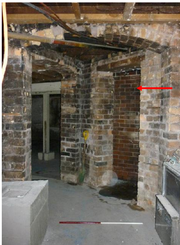
Figure 35. Arched doorway in the hall and in the scullery/store room on the left. The bricked in doorway (arrow) is the beer cellar entrance. Facing west. (1m scale shown)
