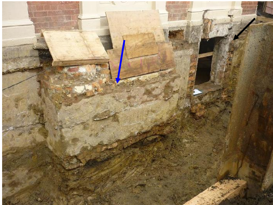
Figure 42. Window Box A after demolition (black arrow); Window Box B and the coal shute (blue arrow). Facing southwest
