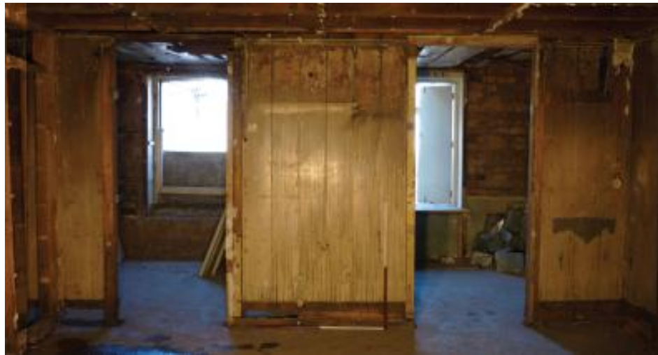
Figure 29. Kauri panelled walls of the pantries. The two windows are also partially visible. Facing south
