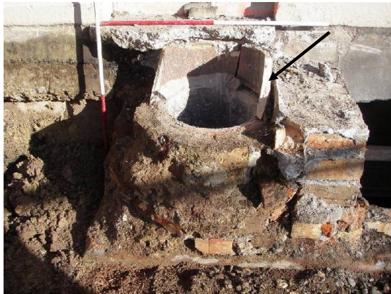
Figure 44. Top of the coal shute, with modern ceramic pipe insert (arrow). Facing south (1m scales)
