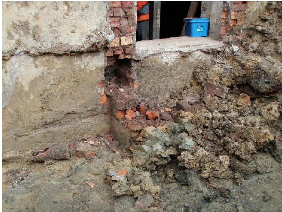
Figure 50. Window Box F during demolition, down to the bluestone block. Facing southeast
