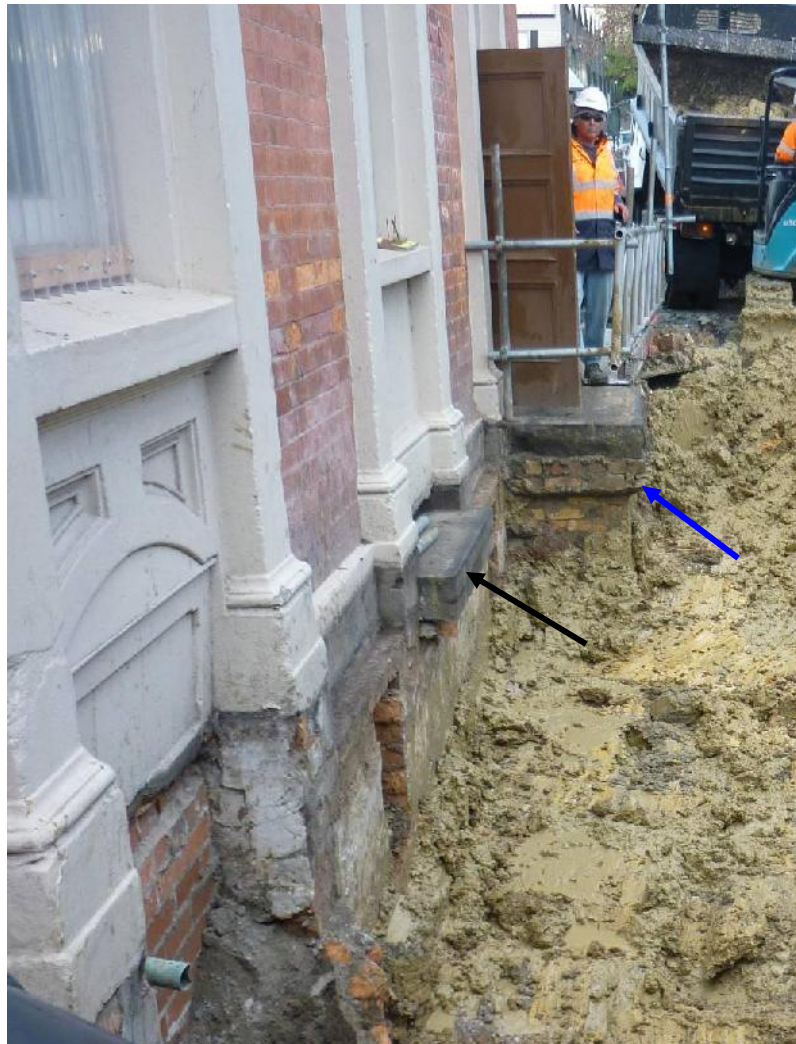
Figure 54. The original west door (centre, arrow) which was later modified into a window, and the new door step above Window Box F exposed during excavation of the trench (blue arrow). Facing south
