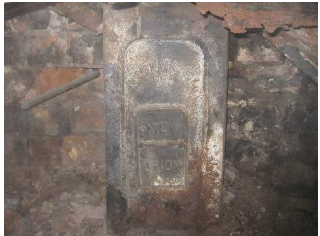
Figure 27. The Shacklock Orion coal range located in the kitchen/scullery, prior to removal. The name on the right hand photo says: Shacklock Ltd. Patent Orion
