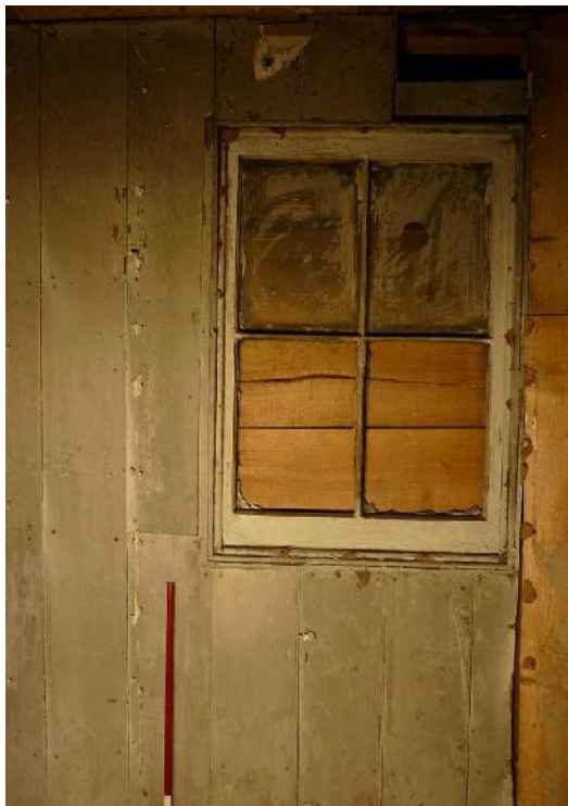
Figure 30. Kauri panelled wall with four pane window separating the coal cellar from the storeroom. The view from the coal cellar (left) and storeroom (right) (red and white scales measure 1m)
