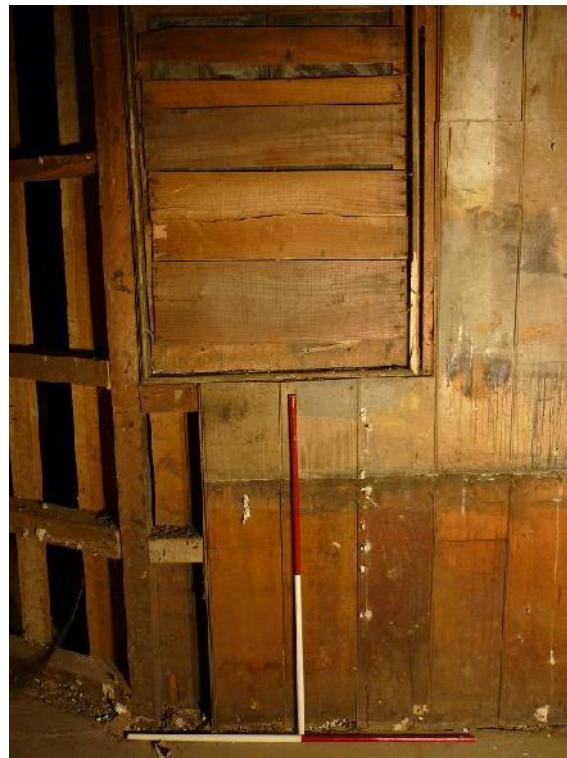
Figure 30. Kauri panelled wall with four pane window separating the coal cellar from the storeroom. The view from the coal cellar (left) and storeroom (right) (red and white scales measure 1m)
