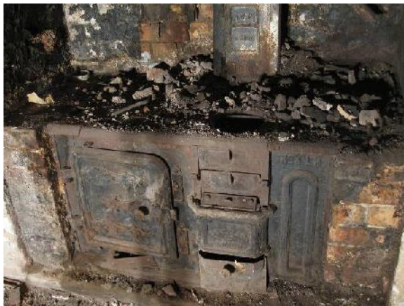
Figure 27. The Shacklock Orion coal range located in the kitchen/scullery, prior to removal. The name on the right hand photo says: Shacklock Ltd. Patent Orion
