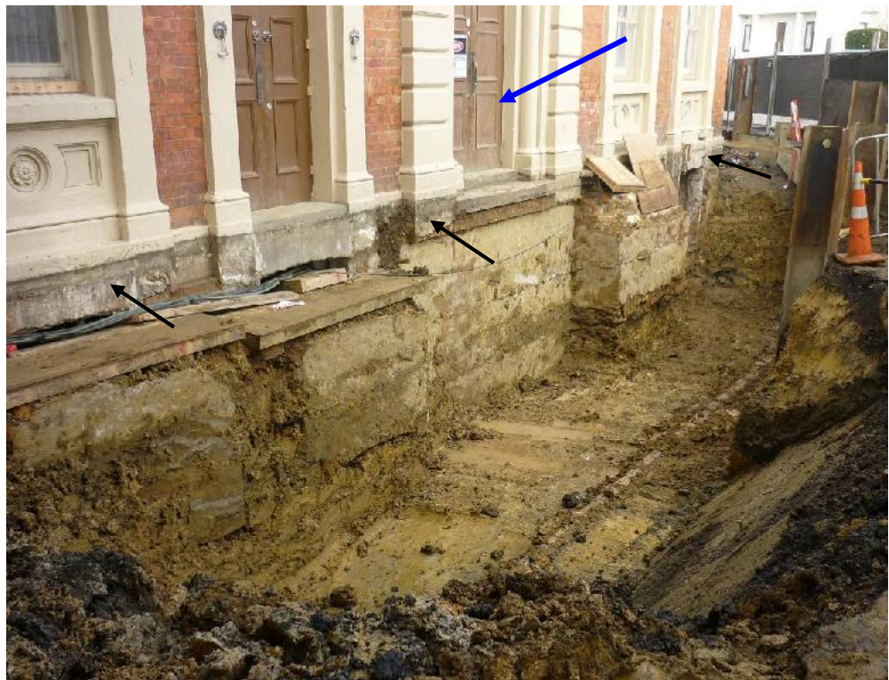
Figure 40. The dark band (arrows) indicates the original ground surface level once the Rob Roy Hotel was completed. The original private entrance is indicated by the blue arrow, with the door to its left being a later alteration of a window to a door. Facing southwest
