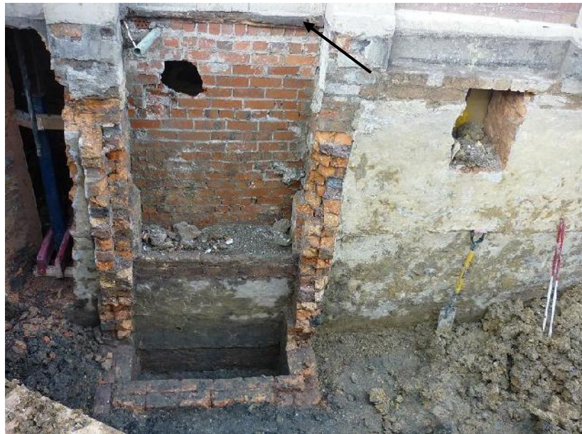
Figure 47. Cellar Door E, which had been bricked over in the late 20 th century from the inside. The arrow points to the base of the wooden cellar door at ground level. Facing east
