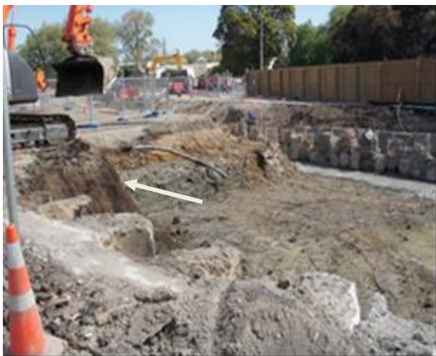
Figure 83. Variation in the upper 2m is seen on the left, with different deposits visible. On the right, the concrete beams are part of the roof extending across the tunnel (east-west). The arrow marks the ground surface level in the background, and the foreground illustrates the level after the 2m had been removed
