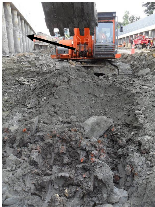
Figure 109. The ground surface level is indicated by the arrow on the concrete piles (left) near Well 1 (the well is located outside of this photo). The grey degraded mudstone layers dominated the stratigraphic profile
