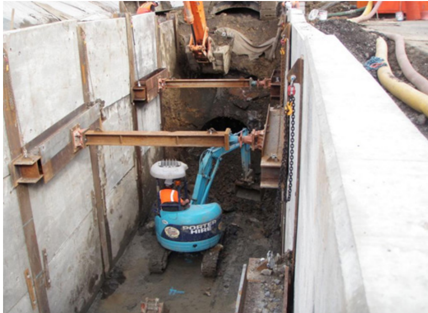
Figure 69. View facing south showing the excavation of the 19th century stormwater culvert in the area behind Franklin Mews (southern section of Area 3)
