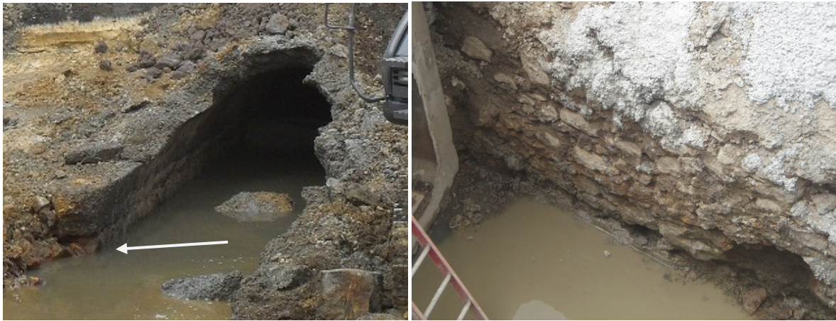
Figure 102. The base of the concrete and start of the faced internal basalt blocks is indicated by the arrow (left), and the unfaced rough blocks on the exterior surface (right)
