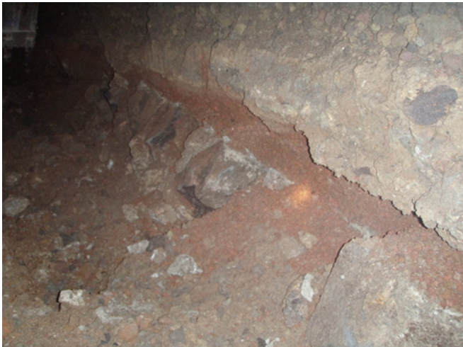
Figure 36. View facing northwest showing the south facing section of the seawall. The seaward slope of the sea wall can be seen descending to the north, into the section. The reddish scoria material is derived from the fill around a concrete pipe just to the north. The concrete steps are shown in the right-hand photo
