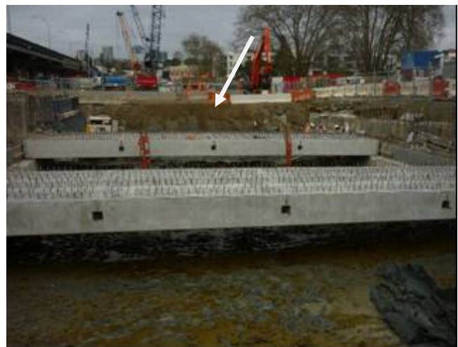
Figure 83. Variation in the upper 2m is seen on the left, with different deposits visible. On the right, the concrete beams are part of the roof extending across the tunnel (east-west). The arrow marks the ground surface level in the background, and the foreground illustrates the level after the 2m had been removed
