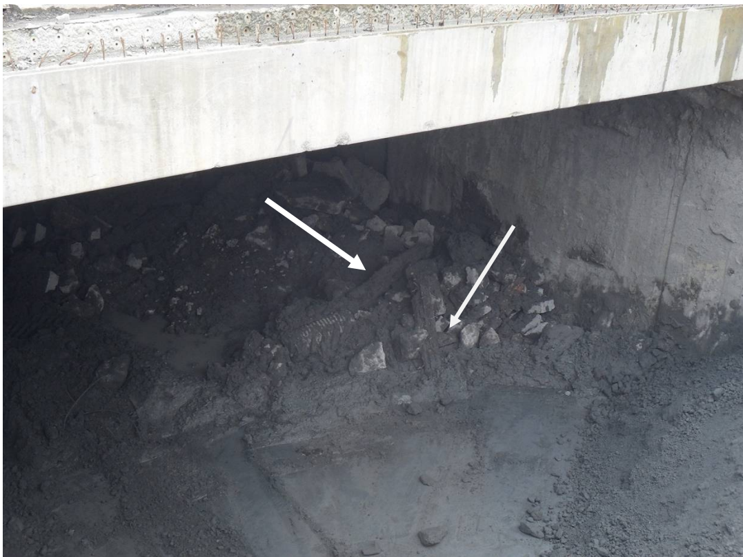
Figure 95. The two timber piles within the tunnel excavation just in front (north) of the original location of the Birdcage Tavern
