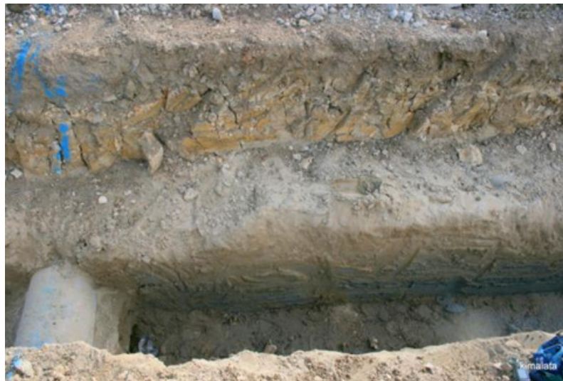
Figure 27. Stormwater pipe located on top of marine sediments and below benched soil and clay layers. Facing south
