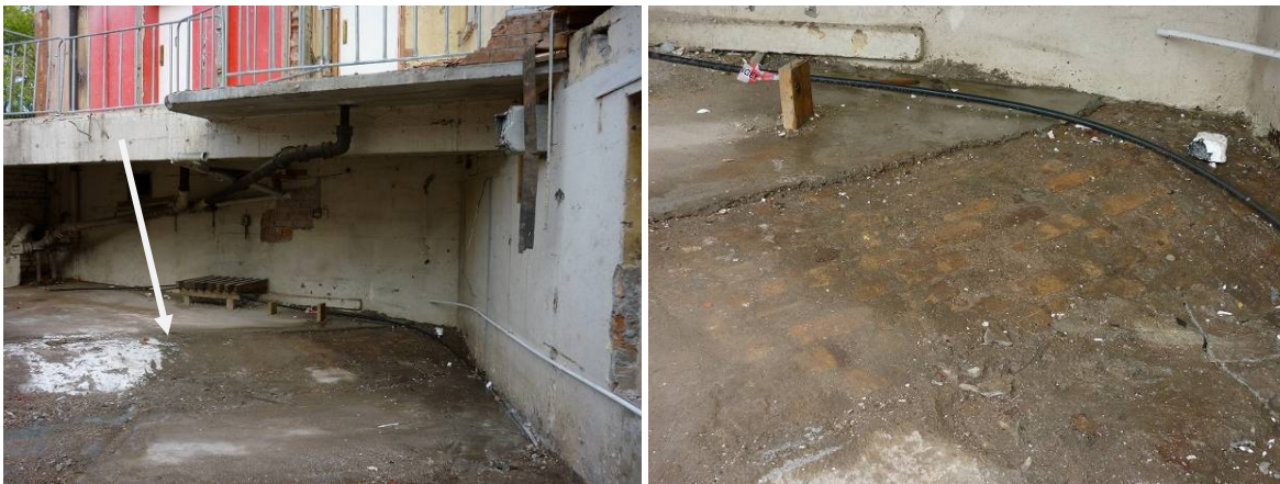
Figure 103. The top of the stormwater as it was exposed in the former yard of the Birdcage Tavern. Note the bricks in the top arch, in contrast to the concrete arch present to the south of this area
