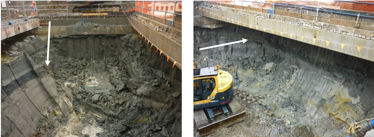
Figure 84. Typical stratigraphy in the central area of the former bay/Victoria Park. The former sea floor (654) is obvious as the dark band (left) and some additional layering around the sea floor is visible on the right
