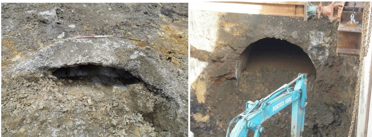
Figure 101. Photos of the top arch of the culvert illustrating the thickness and coarseness of the concrete (50cm scale shown)
