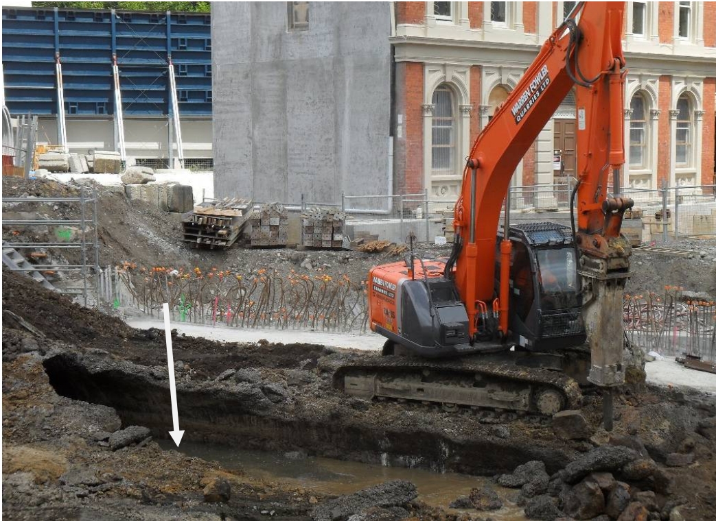
Figure 98. Demolition of the culvert with water visible (arrow), and the Birdcage Tavern in its temporary location in the background
