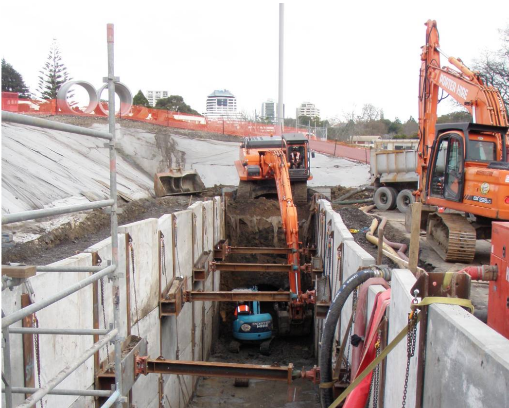
Figure 99. Further south of the Birdcage the culvert was demolished within a shored trench. The mechanical diggers are slowly removing sections of the culvert here
