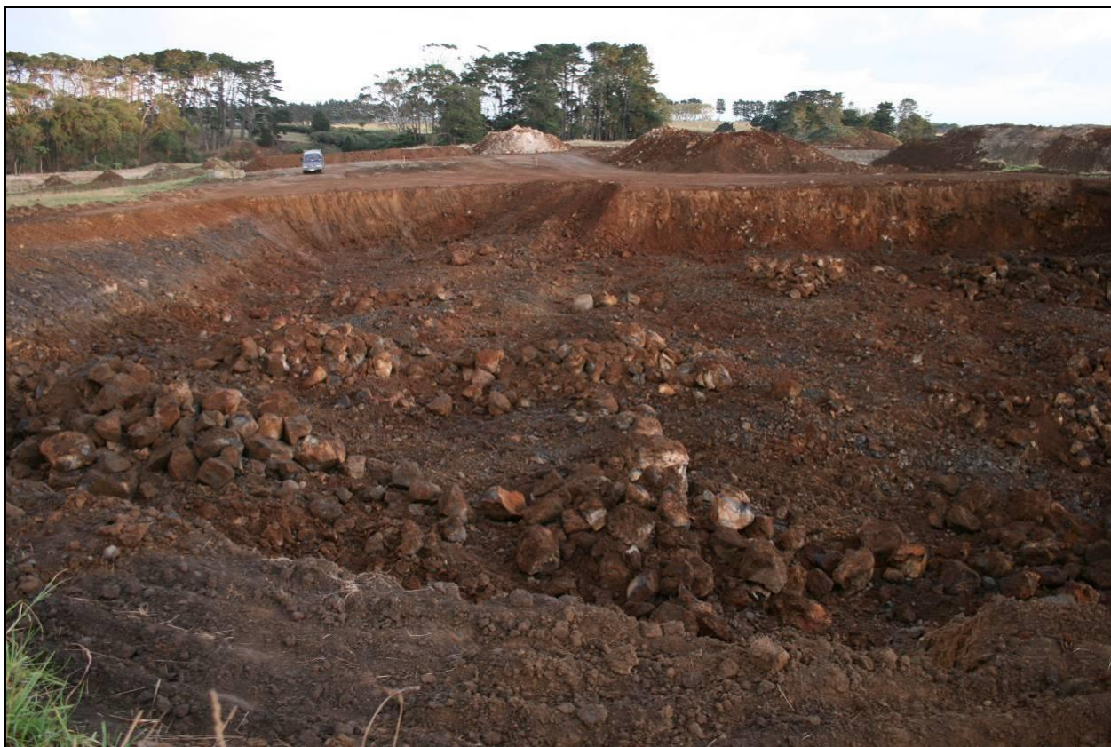
Figure 39. Monitored area mined with topsoil removed, and excavation removing boulders to depth down to 2.5m
