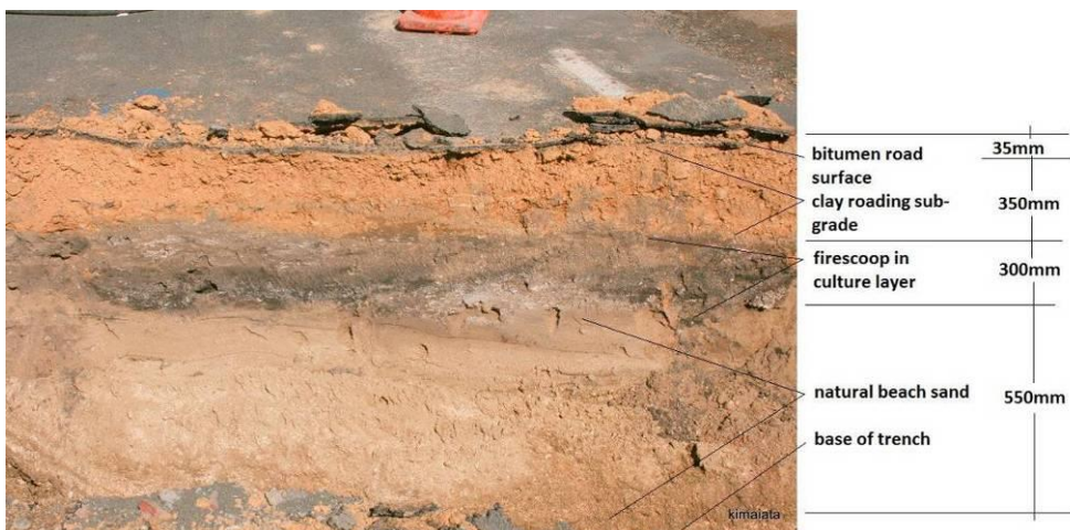
Figure 13. Trench profile across Ferndale Drive showing firescoop (Harlow et al. 2012: Figure 64)
