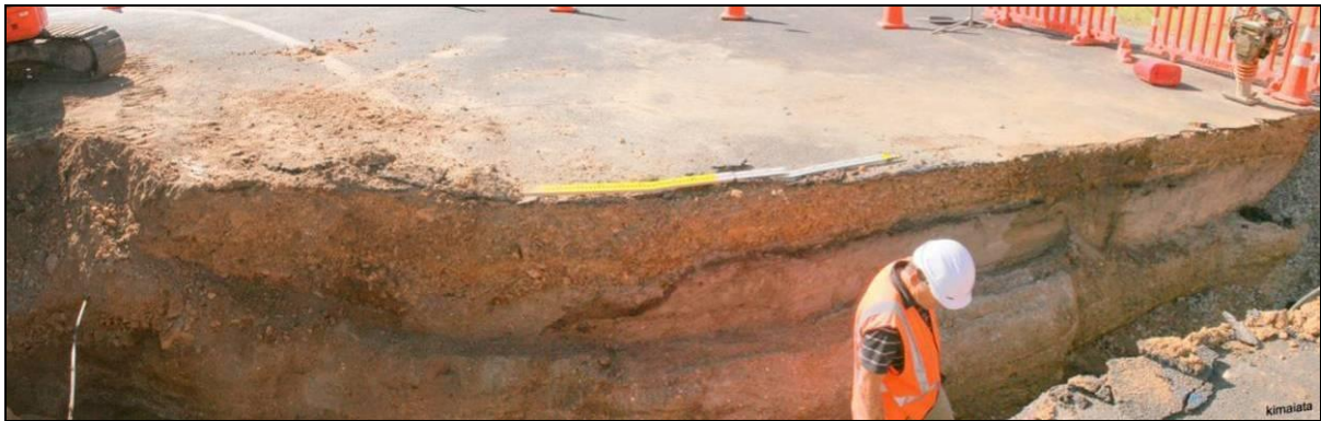
Figure 12. View of wastewater trench (Harlow et al. 2012: Figure 63) across Ferndale Drive showing previous roading other material above natural beach deposit
