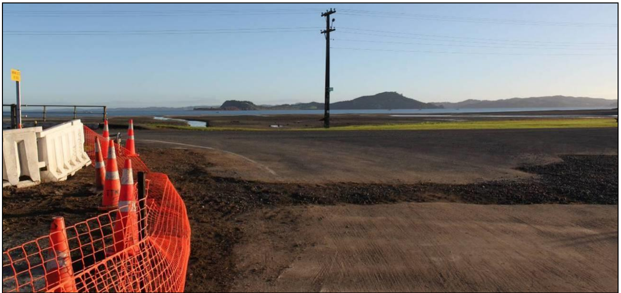
Figure 43. Restoration of pipeline trench across Ferndale Drive
