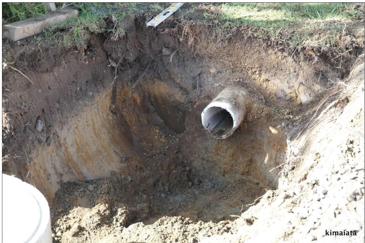
Figure 69. View showing the installation of the stormwater pipe, which had been cut down onto basal yellow marine sand and through a mixed brown topsoil-sand, and fill above the pipe consisting of a mix of stone and sand
