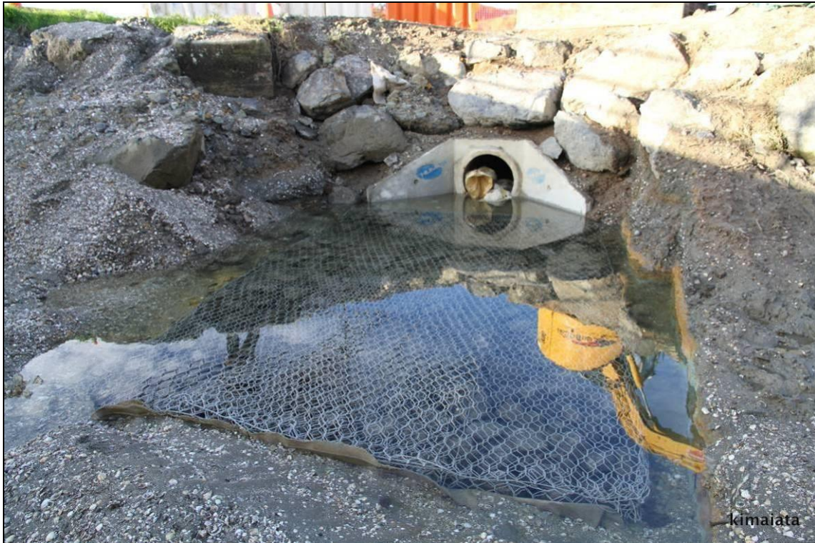
Figure 71. Scour apron installed below stormwater outfall in Rautawa Stream bed
