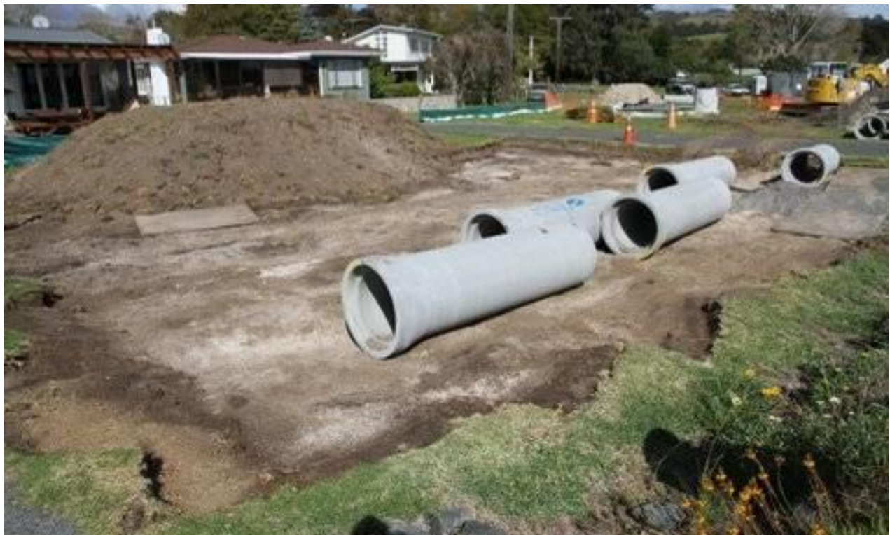
Figure 45. View of pipe laydown along trench alignment
