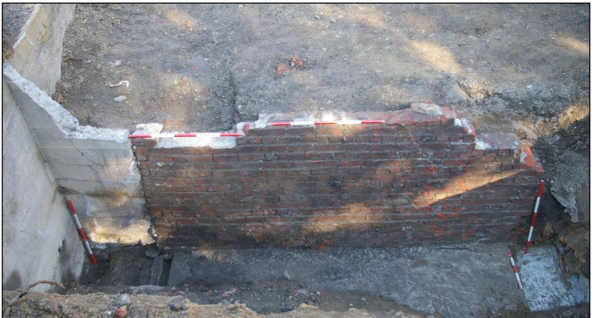
Figure 3.18 The brick wall (context 6016) and concrete floor (context 6021) comprising part of the brick section of Structure 1 situated on the lower terrace, with the buttress of the 1914 concrete retaining wall seen at left. Facing south-southwest. Scale 4 x 1m & 1 x 0.5m
