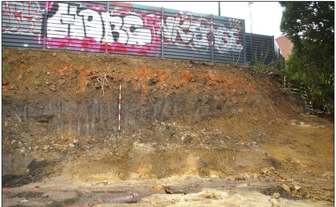
Figure 3.28 Western edge of excavation area at the rear of the crèche illustrating the upper levels of stratigraphy dominated by aggregate basecourse and made ground layers containing construction materials derived from the 1980 demolition of St Patrick’s College
