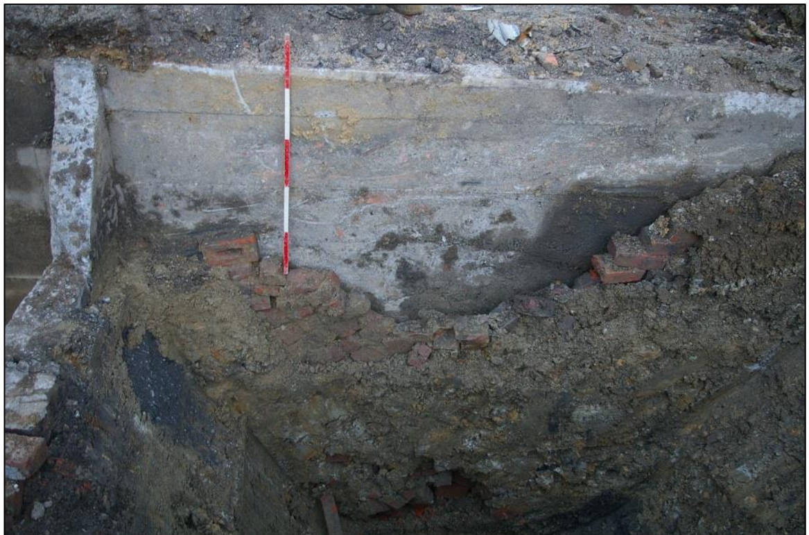
Figure 3.27 The 1914 retaining wall (context 6023) at the rear of the Home of Compassion Crèche seen during the excavations. NB. The bricks derived from the demolition of Structure 2 are clearly visible within the backfill of the construction cut still adhering to the wall. Scale: 1.8m
