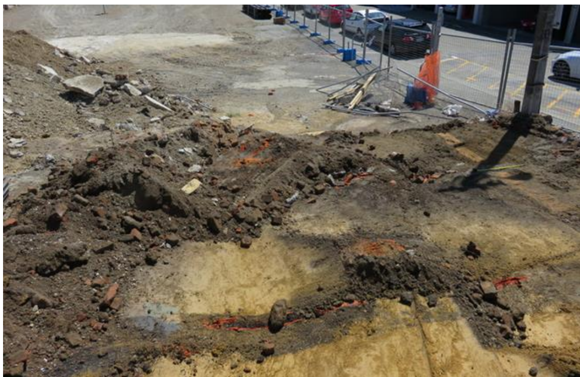
Figure 6.81 Area 2 showing exposed modern and historic drains following removal of brick foundations, facing north-west (10 February 2016)
