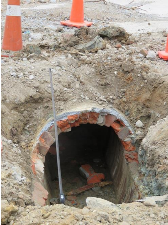
Figure 6.51 Damaged stormwater culvert (1 December 2015; scale 1m
