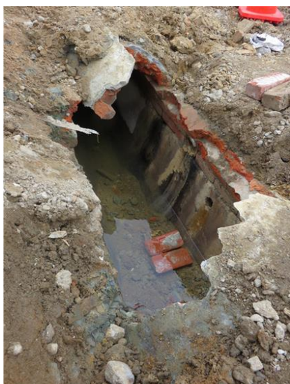
Figure 6.54 Damaged stormwater culvert (1 December 2015)
