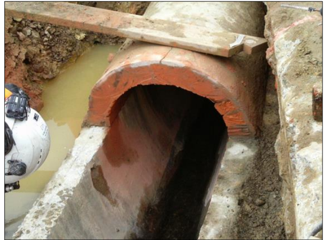
Figure 6.56 Damaged stormwater drain showing interior of stormwater culvert (left); damaged section of stormwater drain cut for repair (4 December 2015; image courtesy Emma Christie)
