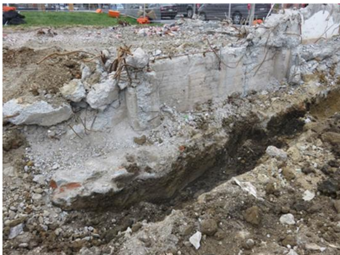
Figure 6.58 Trench A facing south-west showing approximate level of suspended floor foundations (1 December 2015)
