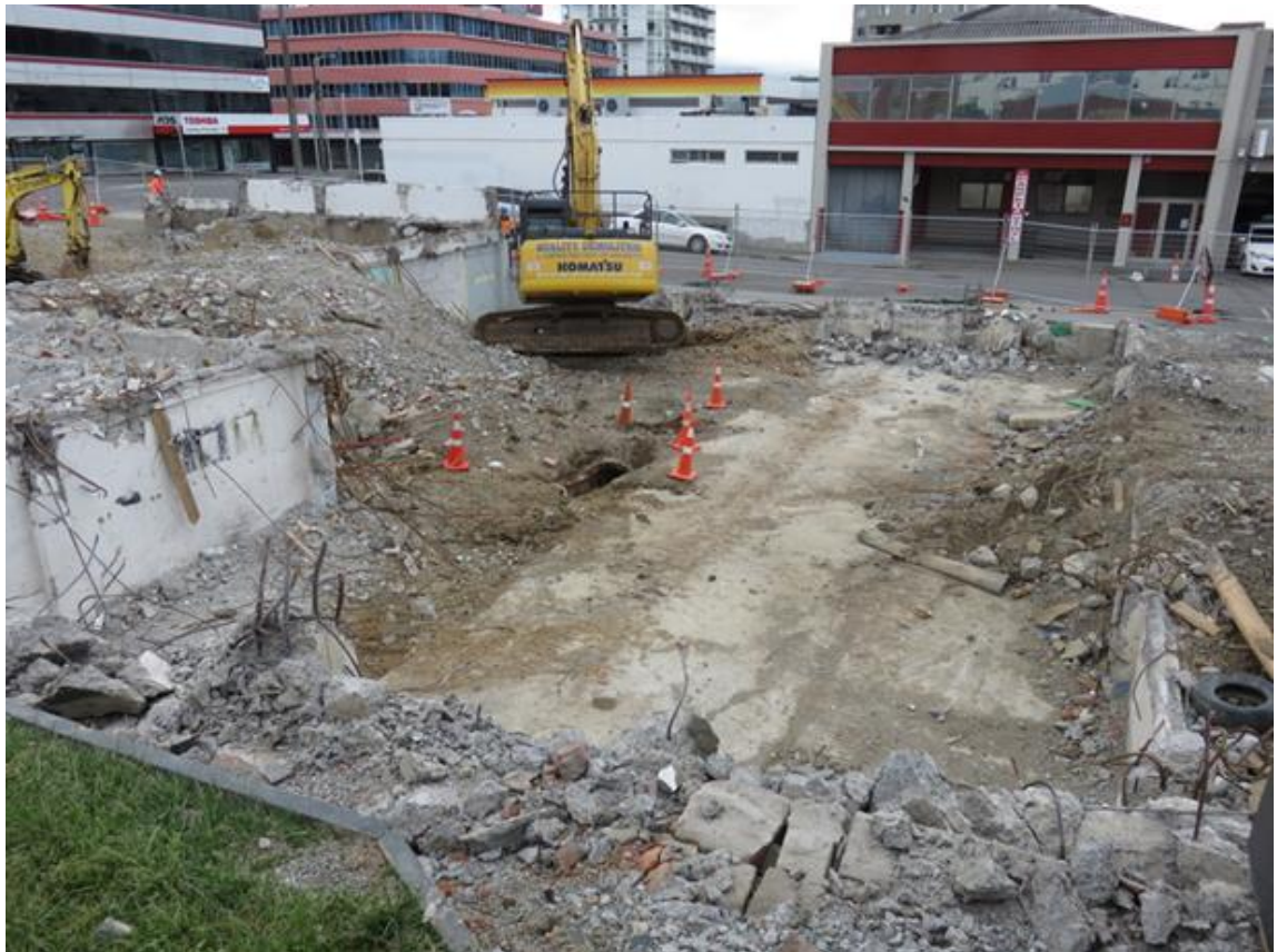
Figure 6.50 Damaged stormwater culvert underneath Bradley's Building rear basement, facing north (2 December 2015)
