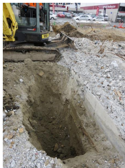
Figure 6.61 Test Trench C showing depth of excavation
