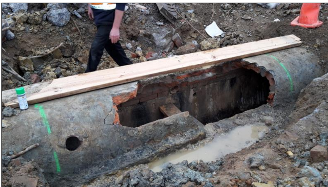
Figure 6.55 Damaged section of stormwater drain exposed (4 December 2015; image courtesy Emma Christie)
