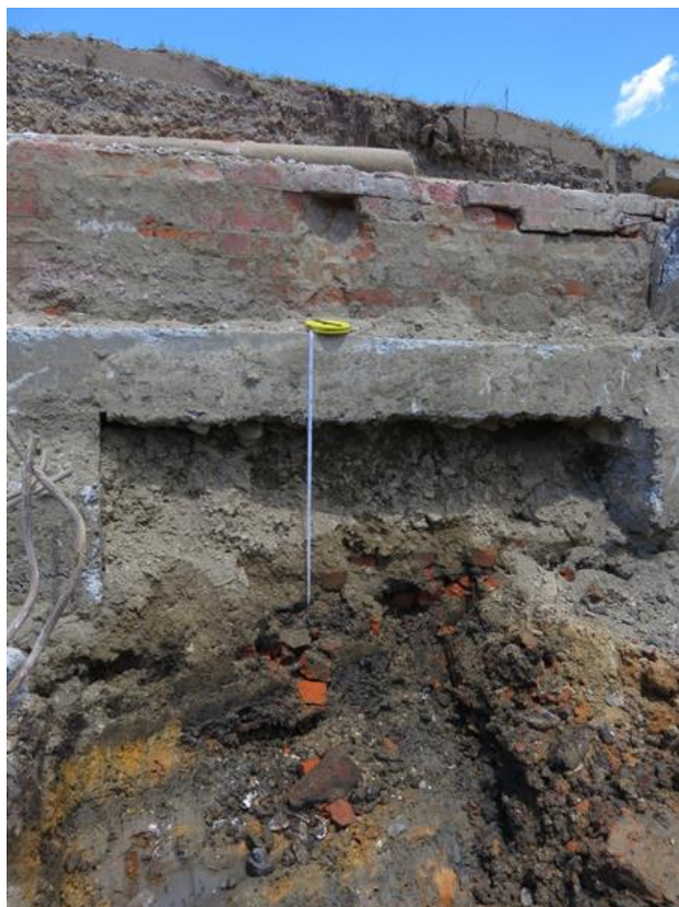
Figure 6.67 South-west boundary wall of 1950s Bradley's Building addition showing stratigraphy within Square A3. Bricks inside concrete footings and rubbish deposit visible at base of scale tape (8 December 2015; scale 1m)
