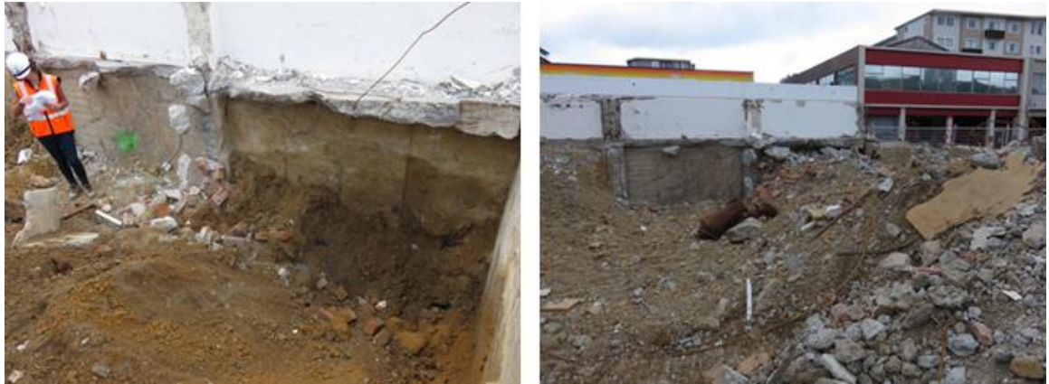
Figure 6.63 Test Trench D following excavation to approximate Martin Square street level (left) and Trench D location prior to excavation (right)
