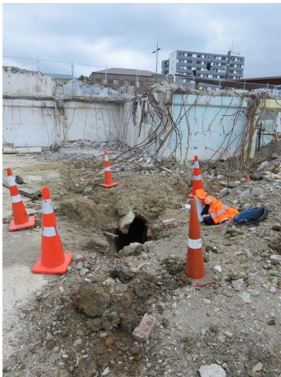
Figure 6.53 Damaged stormwater culvert (1 December 2015)
