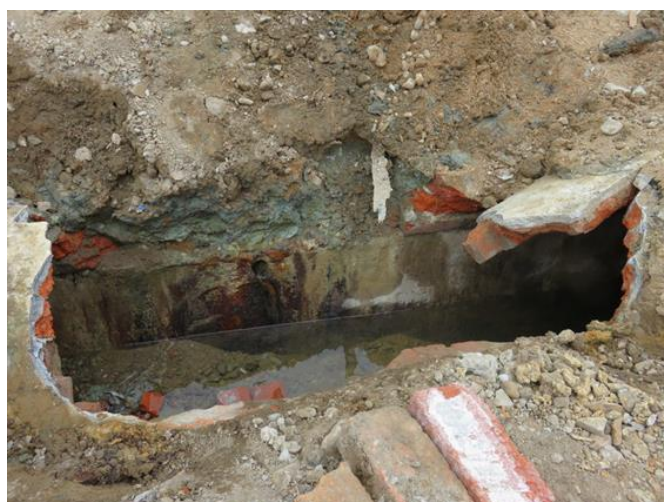
Figure 6.54 Damaged stormwater culvert (1 December 2015)
