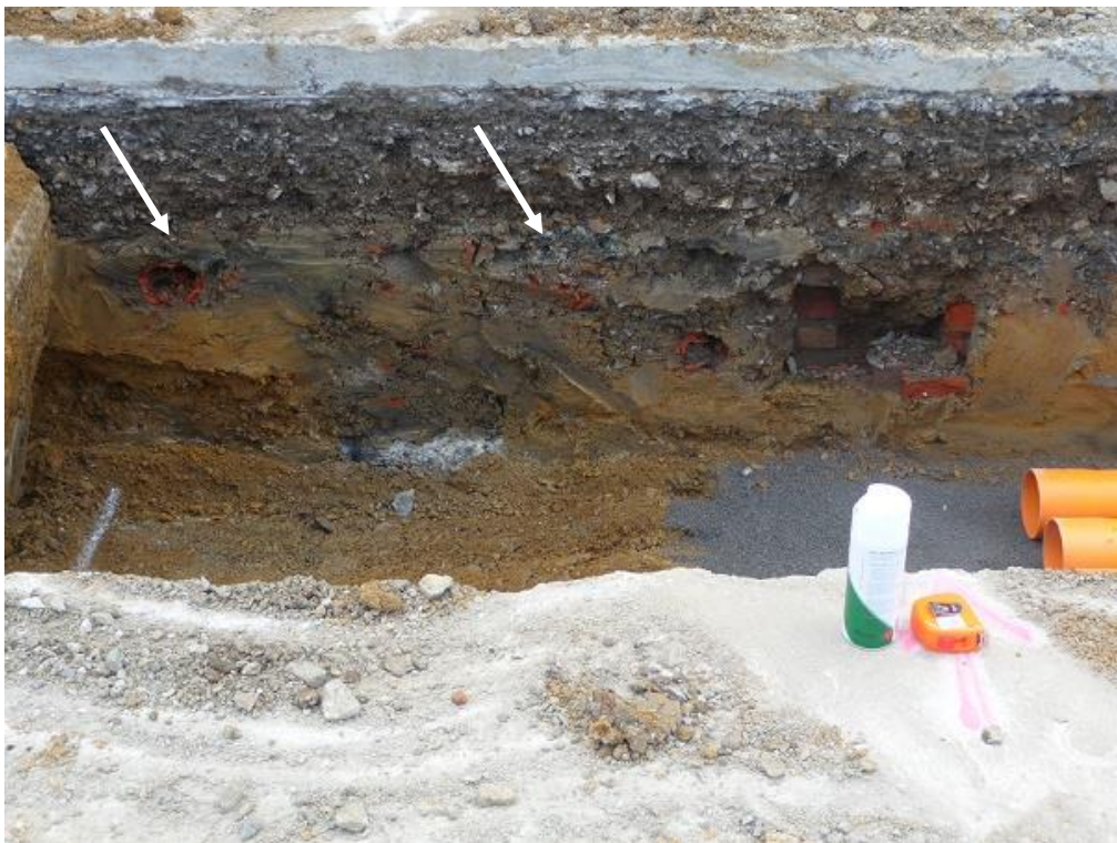
Figure 3.11 Group of four drains, with the two pipe drains indicated by the arrows
