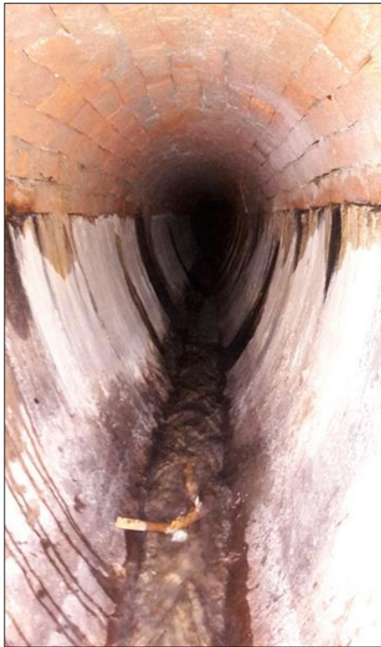
Figure 6.56 Damaged stormwater drain showing interior of stormwater culvert (left); damaged section of stormwater drain cut for repair (4 December 2015; image courtesy Emma Christie)
