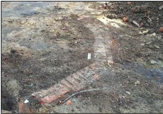
Figure 57. View of foundation wall for bay window (Fraser house)
