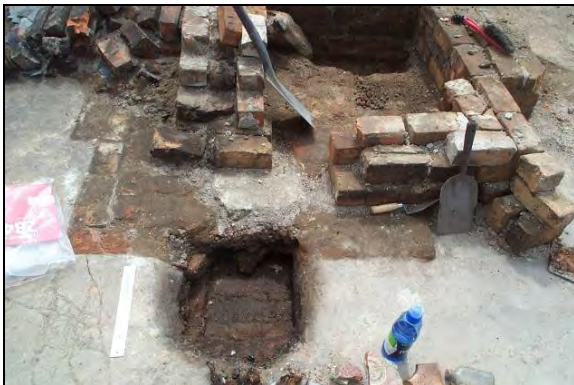
Figure 42. Brick foundation and hole in concrete
