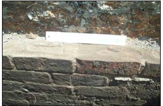
Figure 95. Close up of brick work showing different types of brick used
