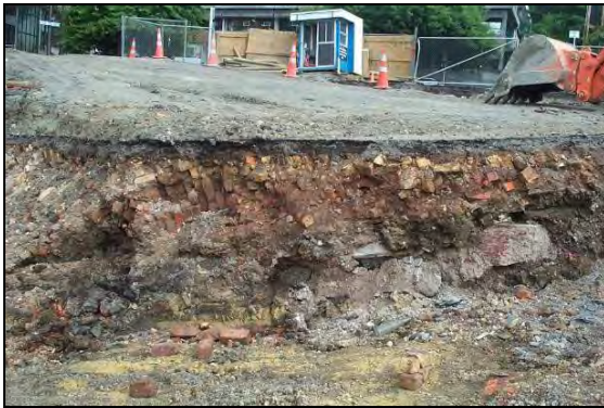
Figure 28. Brick and concrete fill under paving and asphalt at Wynyard St frontage of Allotment 16
