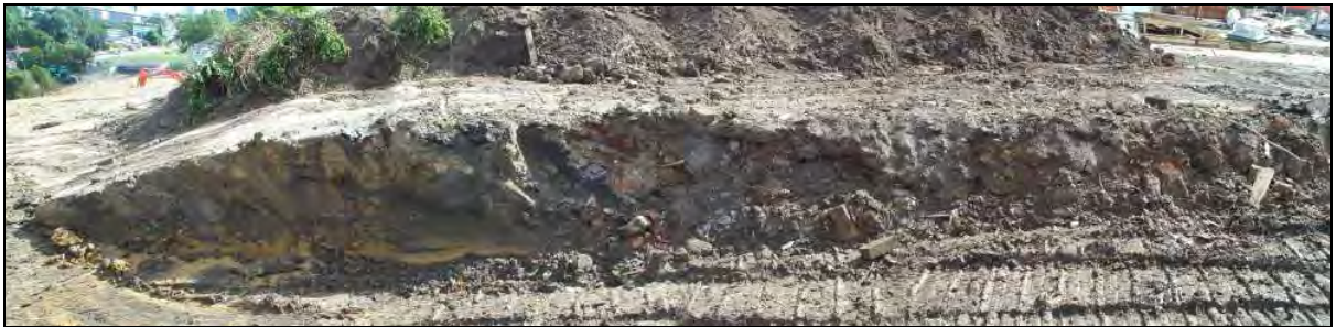
Figure 131. Cross section through fill material showing building rubble used to level the land
