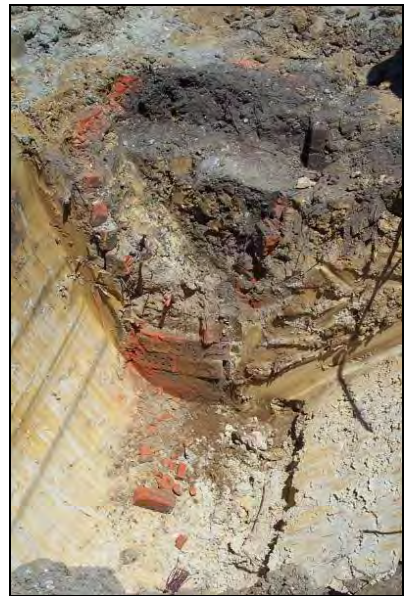
Figure 87. Sectioned view of well
