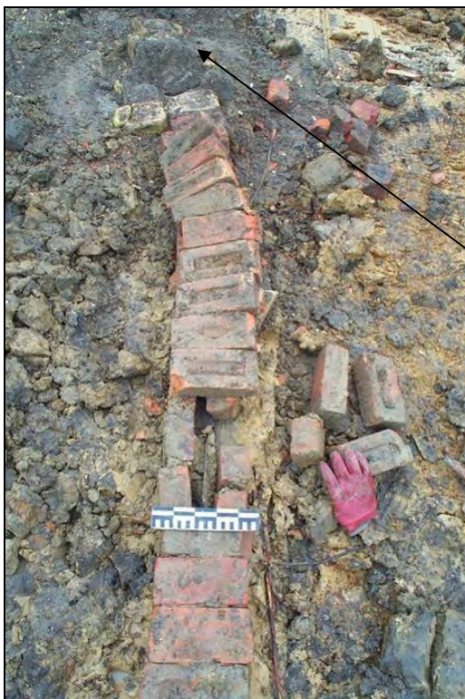
Figure 88. View of frogged brick drain at the front of Allotment 19 (looking west)
