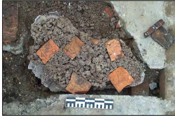
Figure 41. Brick and concrete base course under concrete floor
