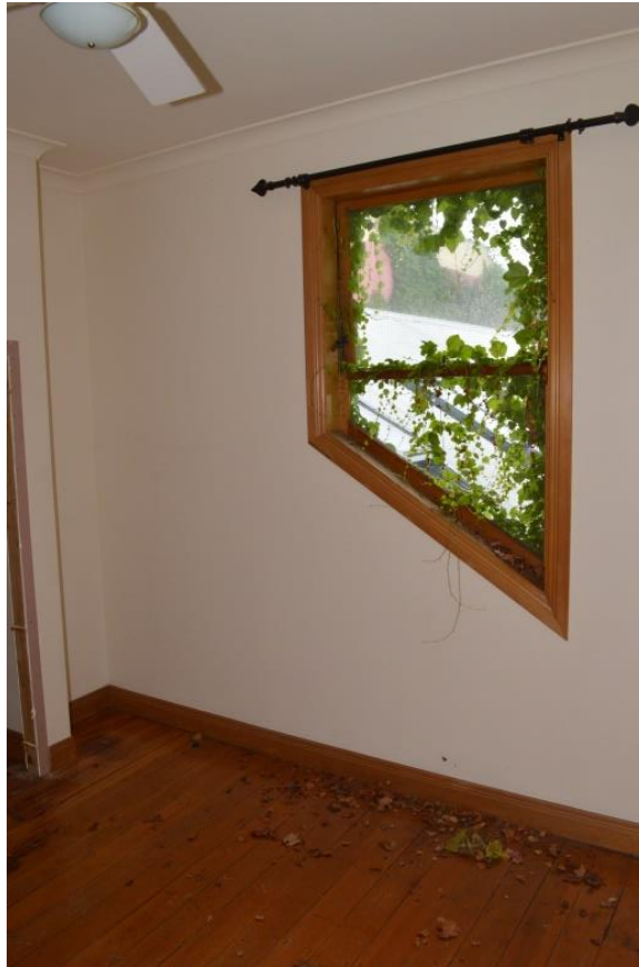
Figure 3.25. Double hung sash window with modification in F03 (source: Clough & Associates, 2015)
