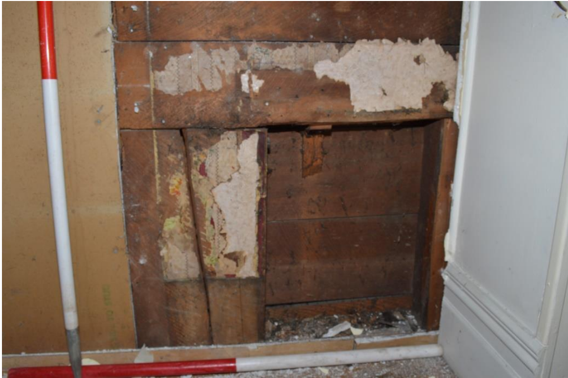
Figure 3.39. Degraded wallpaper layers in G02 and paint stain from blocked-up door architrave (source: Clough & Associates, 2015)
