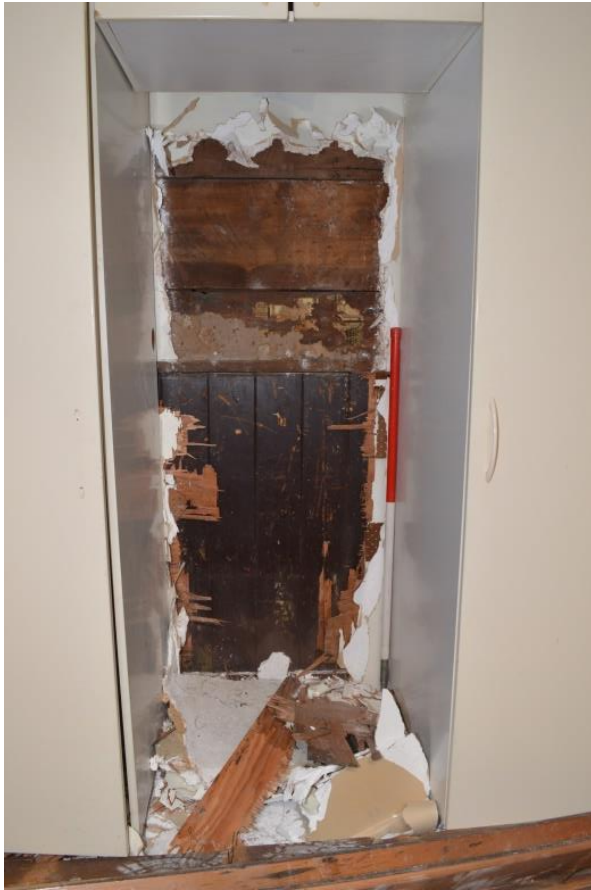
Figure 3.56. Exposed wooden wainscoting on the west wall within G05b behind the modern kitchen (Phase 6) (source: Clough & Associates, 2015)
