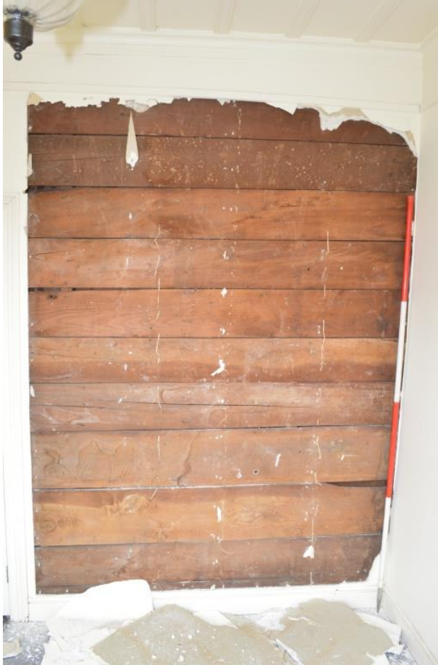
Figure 3.74. Sarking boards covered in F02 (source: Clough & Associates, 2015)
