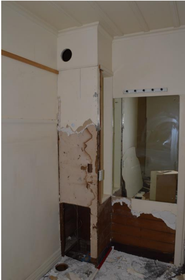
Figure 3.84. Photo showing sarking boards enclosing the removed chimneybreast from the fireplace in G04 (source: Clough & Associates, 2015)
