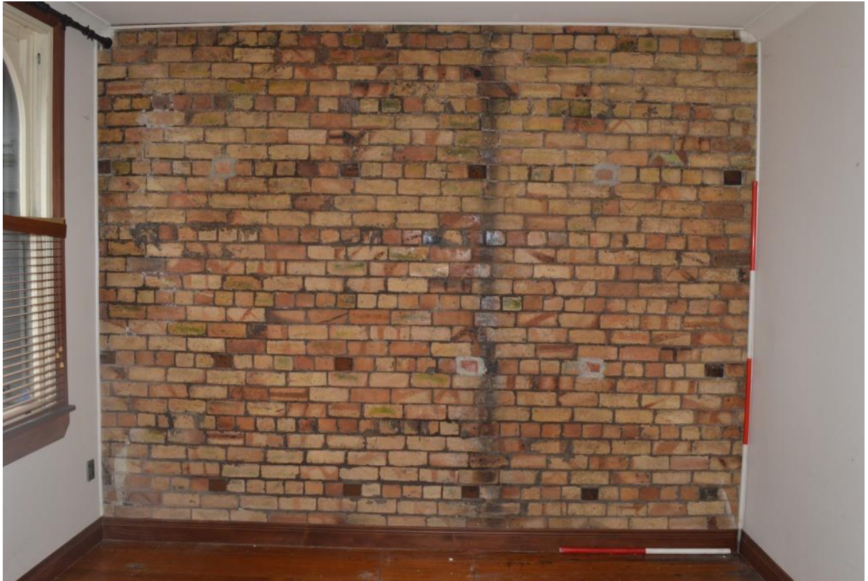
Figure 3.11. Eastern wall of G01 showing brickwork with wooden anchor blocks (source: Clough & Associates, 2015)
