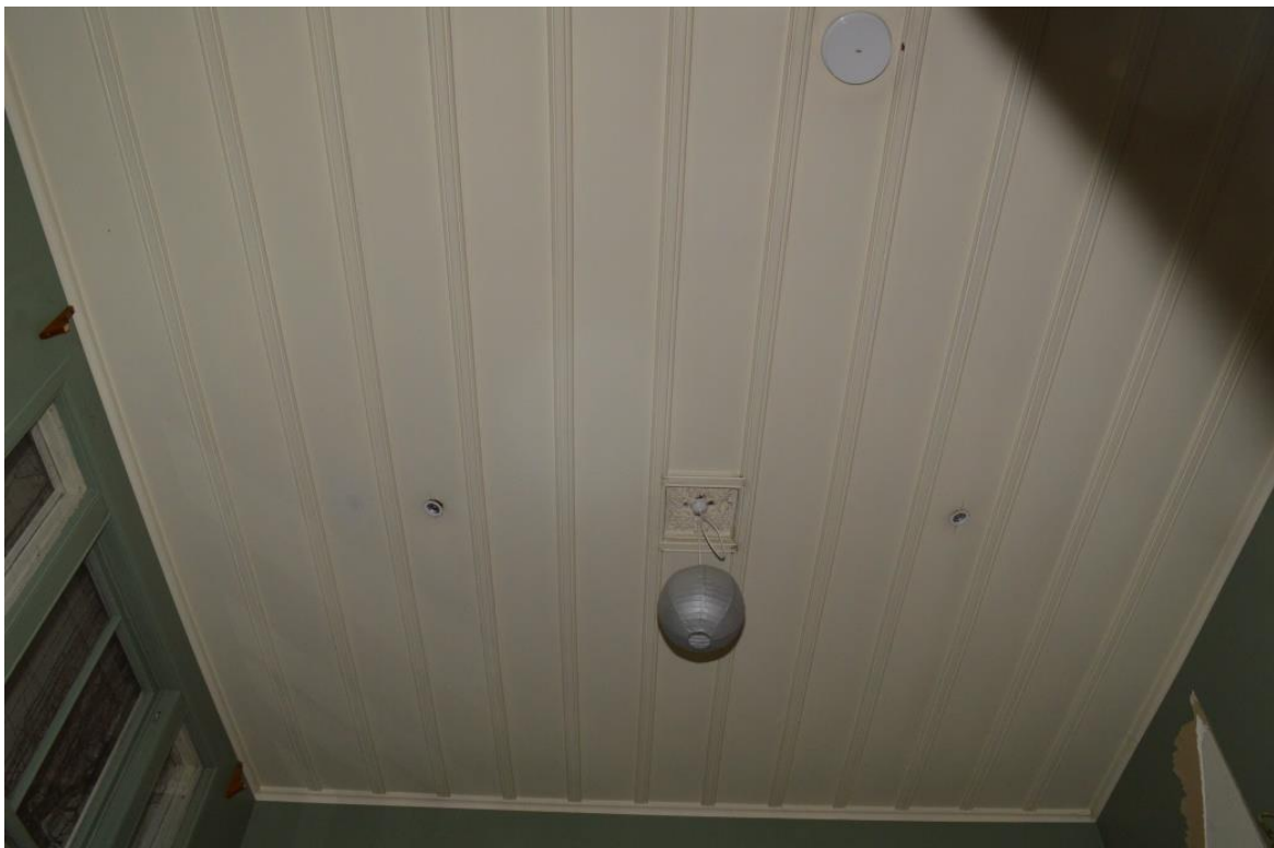
Figure 3.36. Board and batten ceiling in G04 (source: Clough & Associates, 2015)
