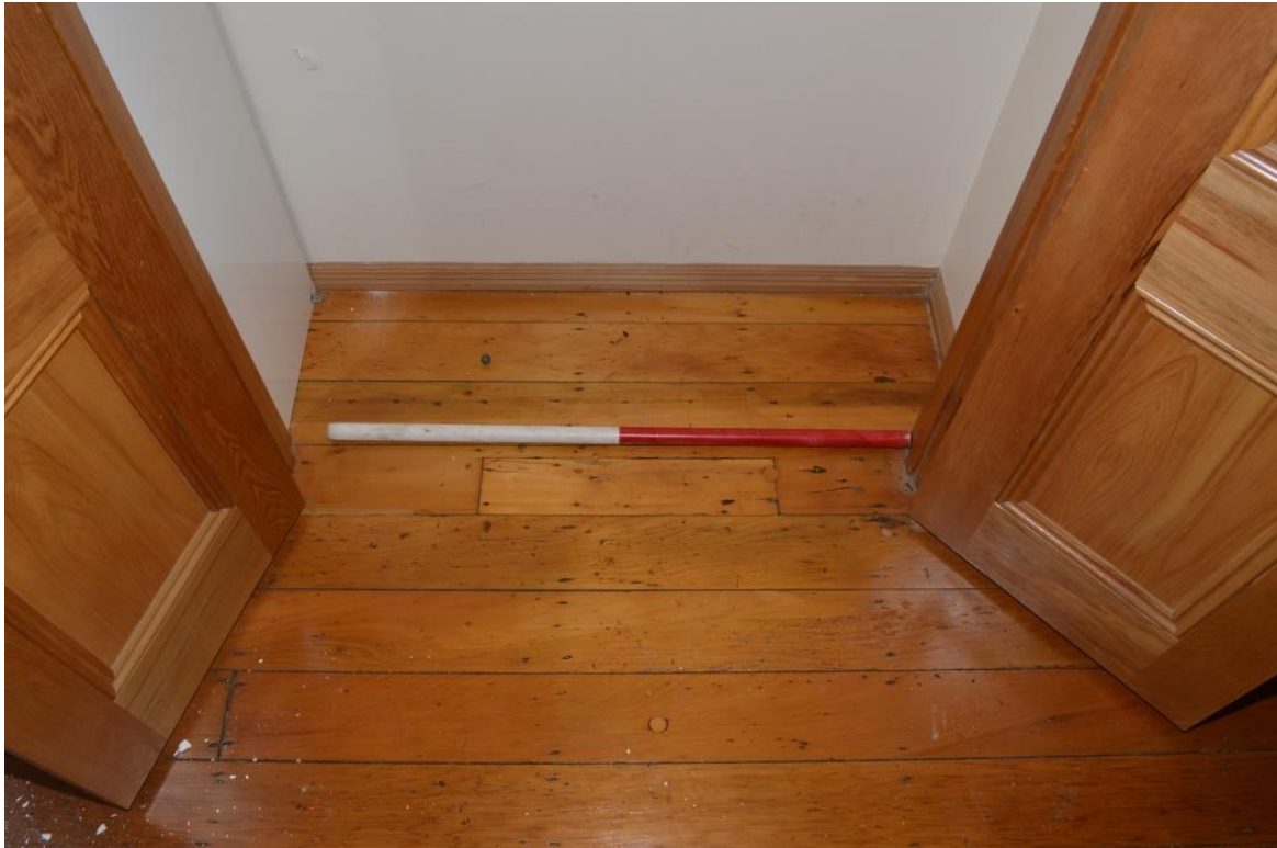
Figure 3.19 Removed north-south running internal wall with the cupboard of F03 (source: Clough & Associates, 2015)
