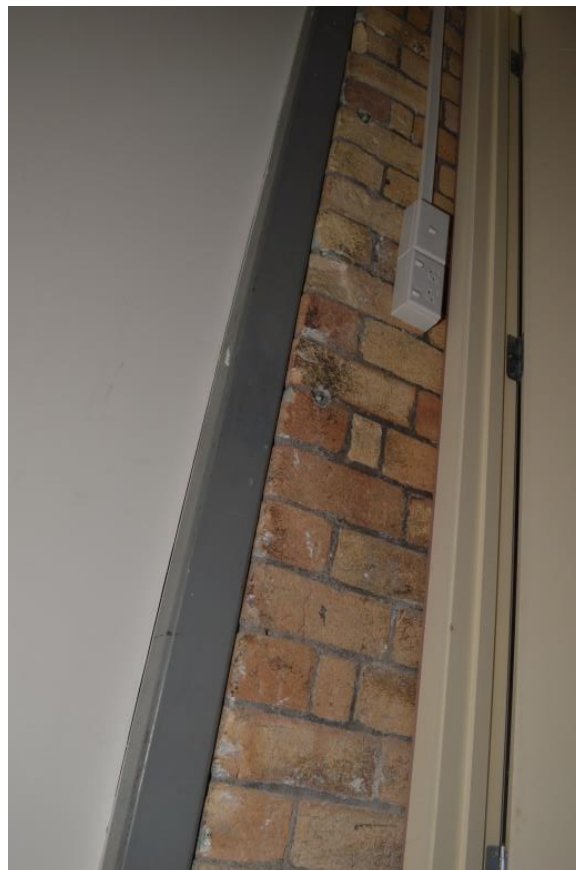
Figure 3.14. Metal support post against the modified Phase 1 brickwork (source: Clough & Associates, 2015)
