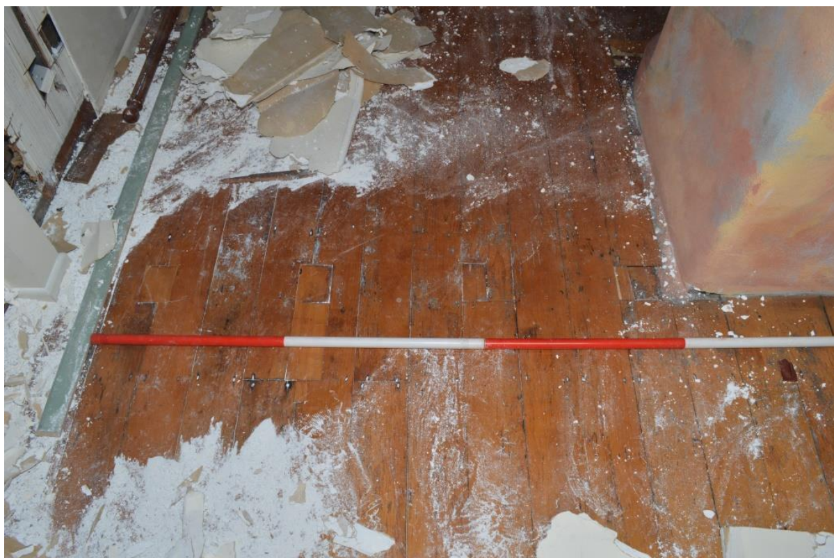
Figure 3.50. Showing edge of timber floorboards and cut-off wall studs delineating the end of G05a and the Phase 1 pre-1900 building. Photo is looking southwards into G05a (source: Clough & Associates, 2015)
