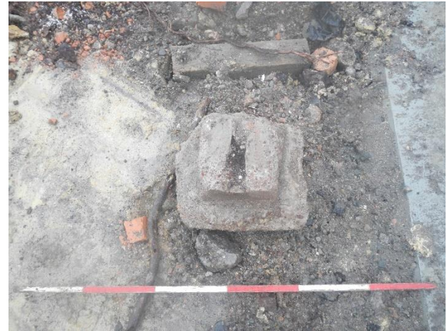
Figure 4.20. View showing concrete pile following removal from the construction cut
