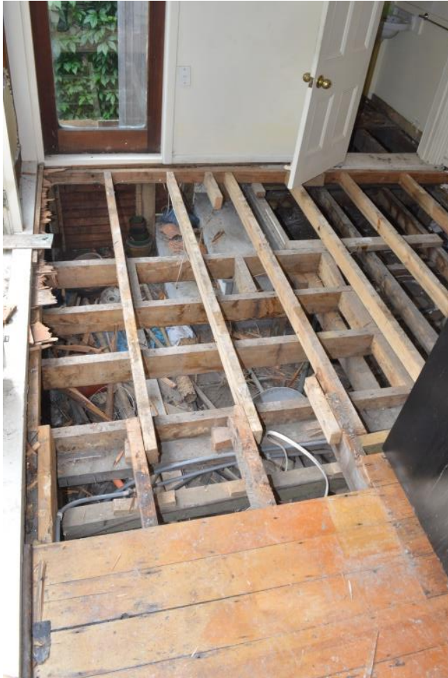
Figure 3.67. Looking north over removed floorboards and exposed subfloor in G05c from G05b (source: Clough & Associates, 2015)
