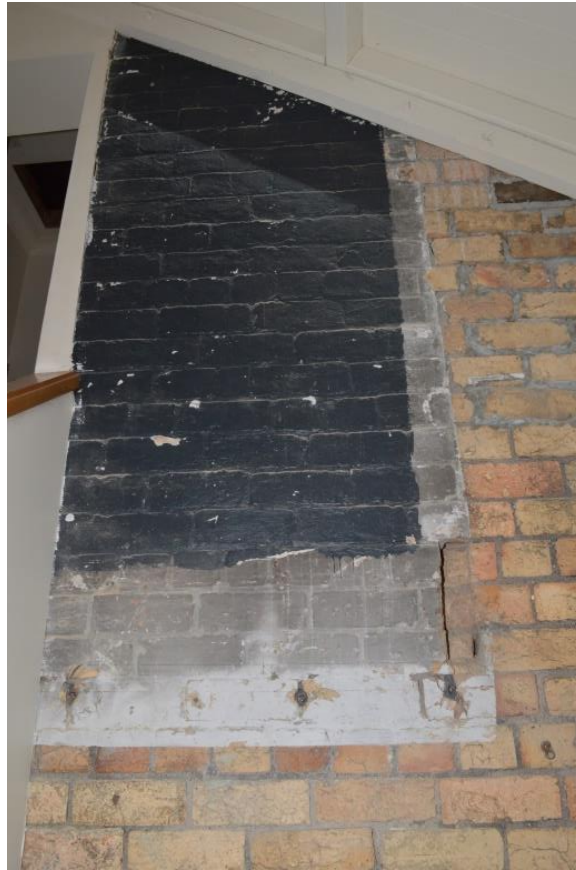
Figure 3.23 North facing elevation showing iron supports on original external wall (source: Clough & Associates, 2015)
