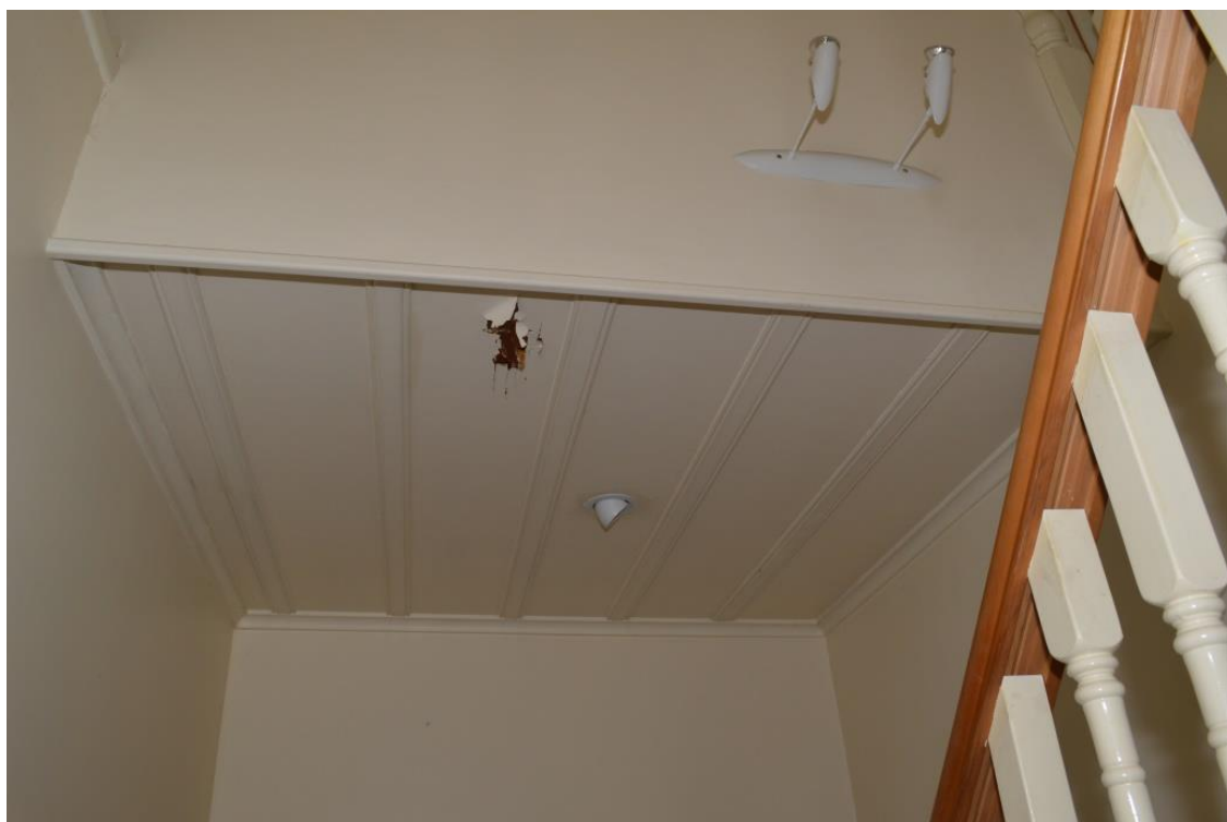
Figure 3.88. Remains of original pre-1900 board and batten ceiling within F06 above second floor staircase (source: Clough & Associates, 2015)
