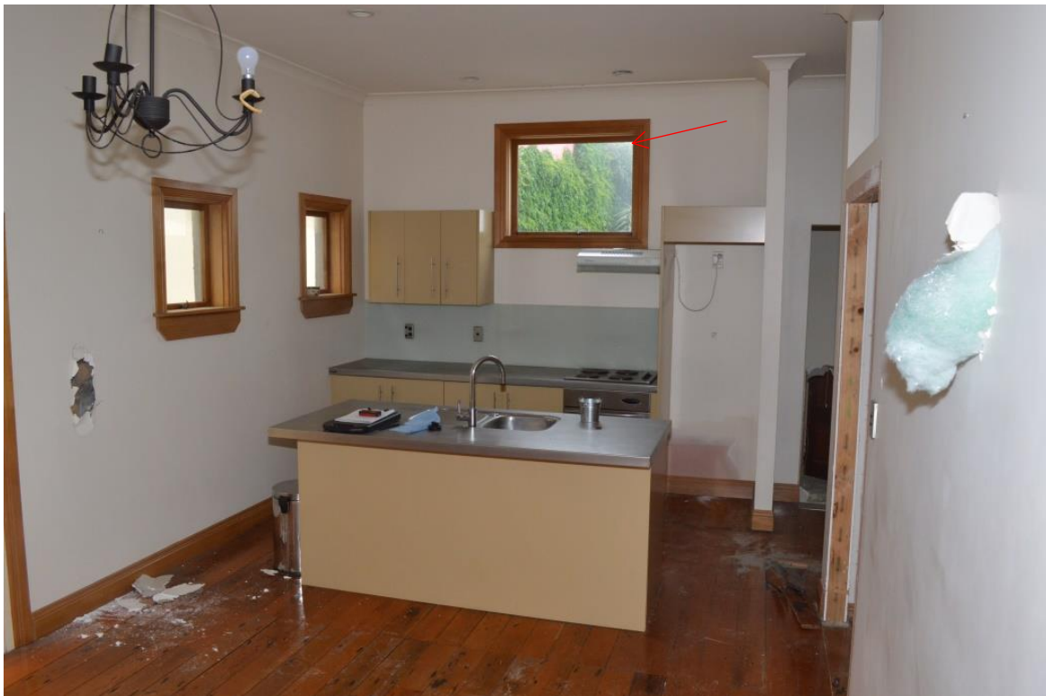
Figure 3.24. Windows within F01 kitchen. The original double hung sash window is marked with a red arrow (source: Clough & Associates, 2015)
