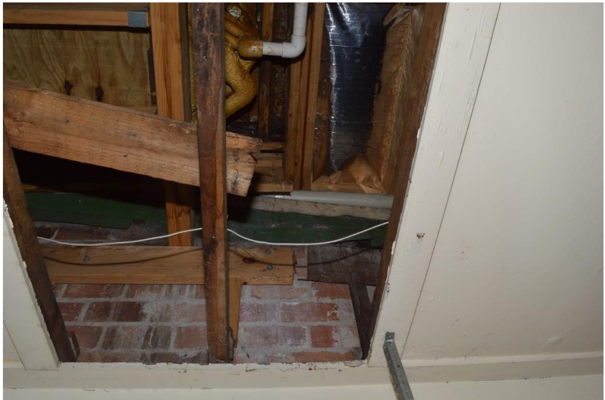
Figure 3.58. Ceiling cavity showing floor studs for Phase 6 decking and green roof flashing for the red brick garage (source: Clough & Associates, 2015)
