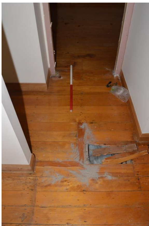
Figure 3.22. Scarring in the original floorboards at the north side of F01, showing a potential enclosed door leading to the Phase 1 fire escape (source: Clough & Associates, 2015)
