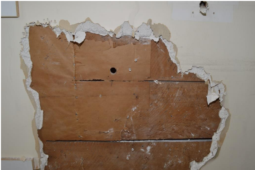
Figure 3.73.Sarking boards covered with brown paper in F01 (source: Clough & Associates, 2015)
