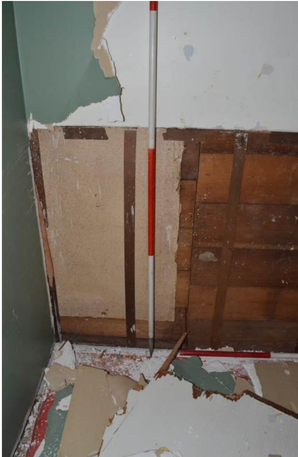
Figure 3.43. Close-up of boarded-up door opening on western wall of G04 with wallpaper (source: Clough & Associates, 2015)
