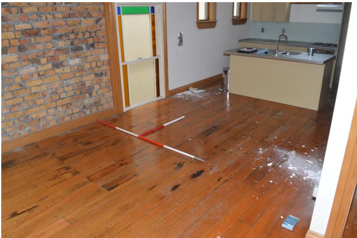
Figure 3.20. Location of infilled stairwell that would have been contemporary with the construction of the two-storey phase 1 building, within F01 (source: Clough & Associates, 2015)
