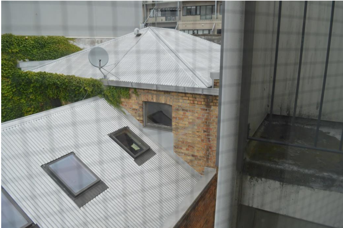
Figure 3.6. Rear (north facing) elevation of 83 Wellesley Street West, showing the blocked Phase 1 windows (source: Clough & Associates, 2015)
