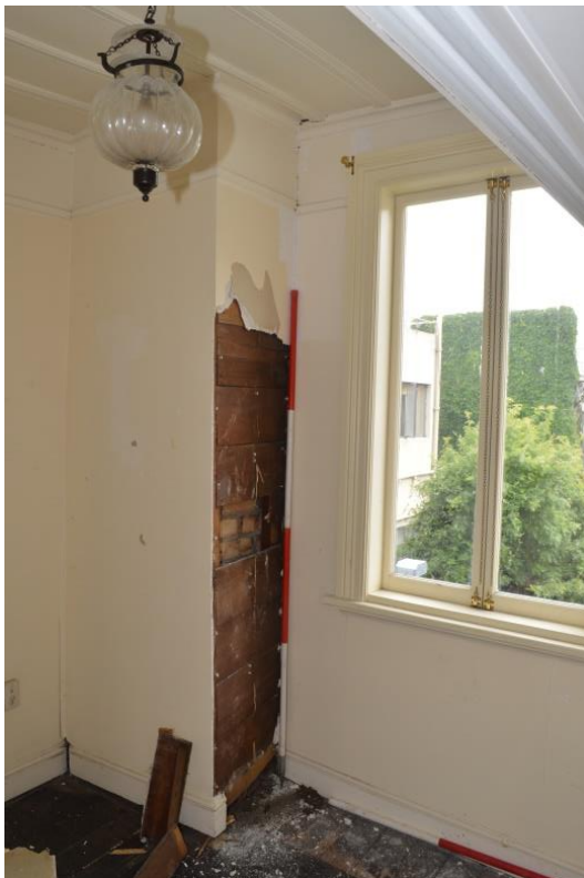
Figure 3.70. Partially exposed chimneybreast within F01 (source: Clough & Associates, 2015)
