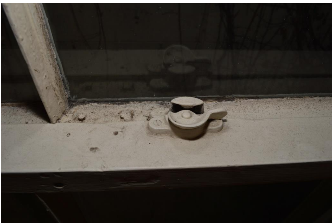
Figure 3.77. Replacement window fastener and scarring of original fastener in F03 (source: Clough & Associates, 2015)
