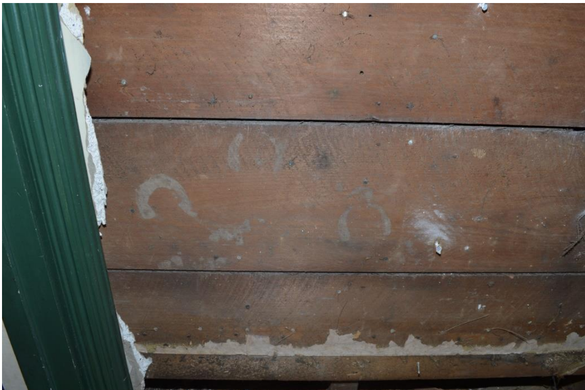
Figure 3.40. Muddy heel cap mark on sarking boards in G02 (source: Clough & Associates, 2015)
