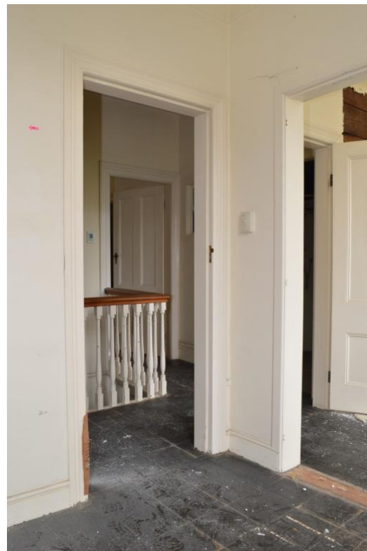
Figure 3.71. Original Phase 1 pre-1900 door architrave and skirting board within F01 (source: Clough & Associates, 2015)
