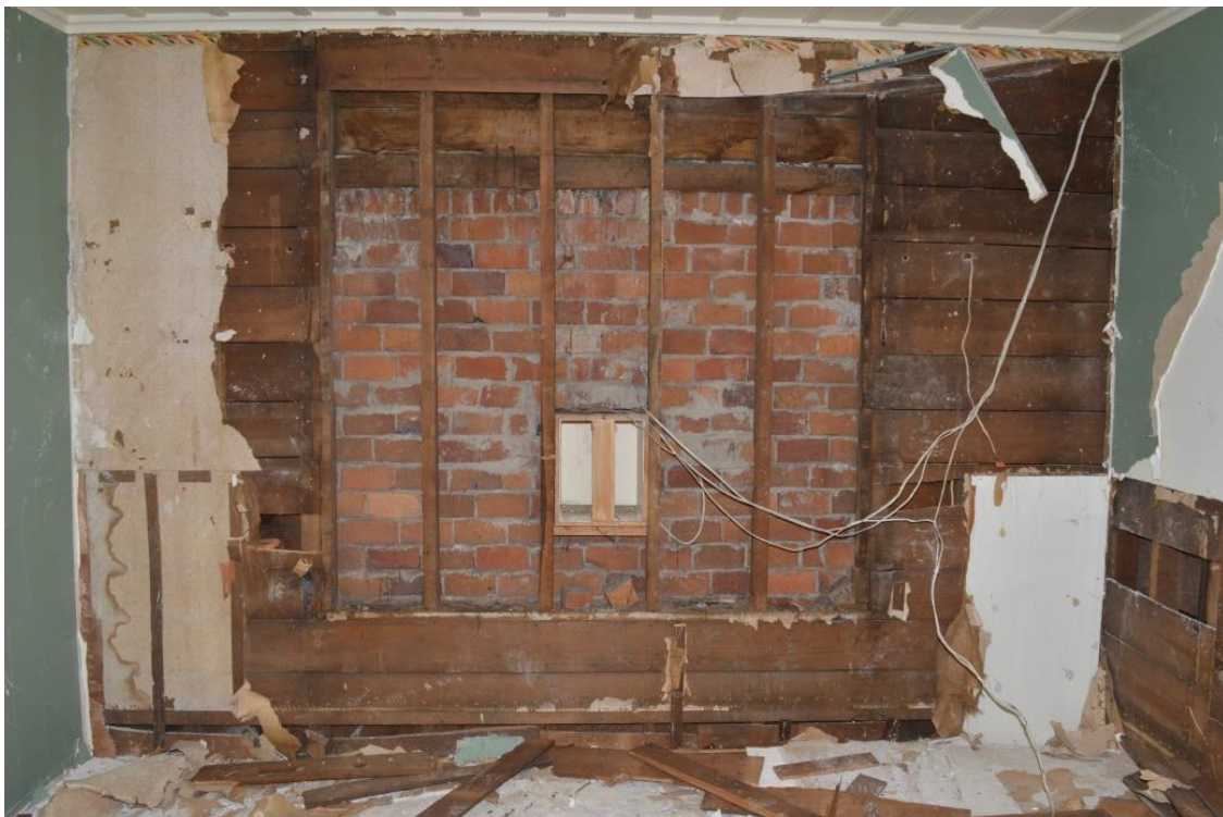
Figure 3.48. Bricked-up window on south wall of G04 from the Phase 3 brick garage extension (source: Clough & Associates, 2015)
