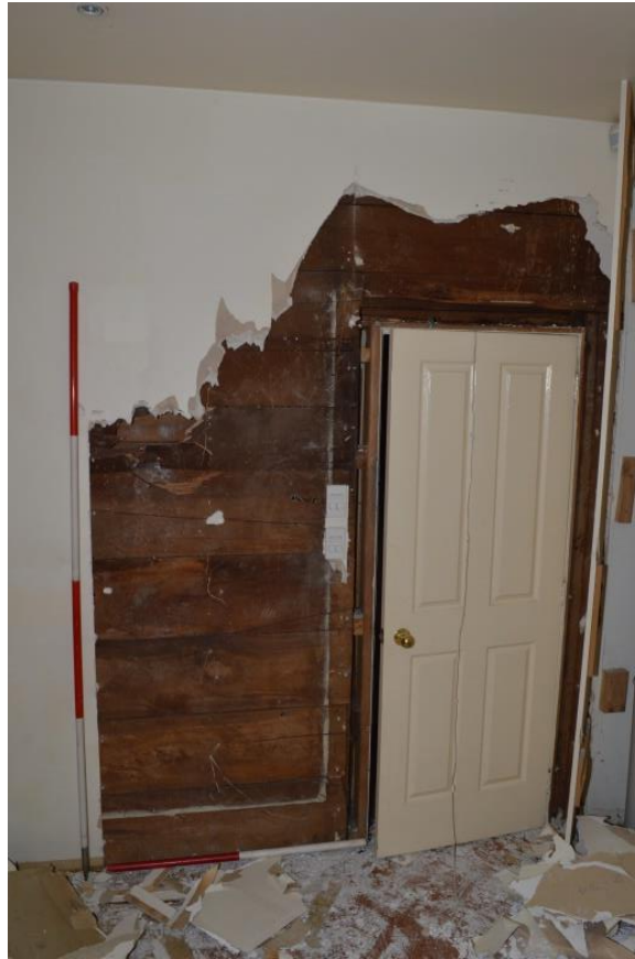
Figure 3.51. Southern wall of G05a, showing opening into G03 with paint traces of former architrave and skirtings (source: Clough & Associates, 2015)
