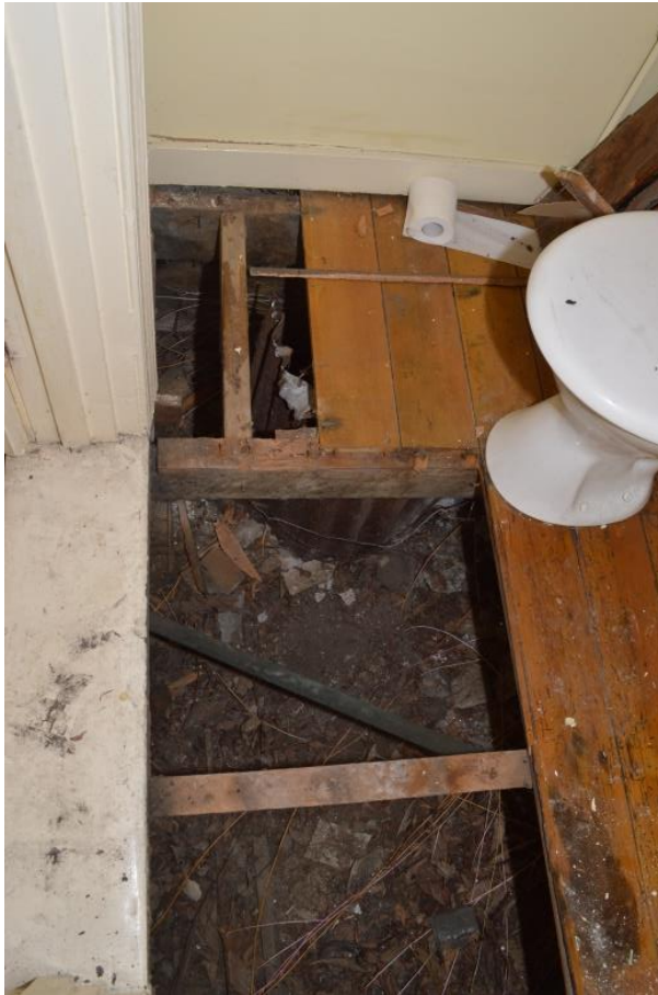
Figure 3.63. Photograph showing removed floorboards, and exposed subfloor structure within G06 (source: Clough & Associates, 2015)
