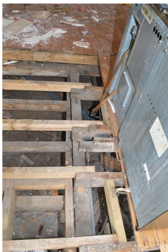
Figure 3.65. Looking south over G05c between G06 (door on left-hand side of photo) and kitchen island (on right). Note the concrete steps marked with red arrow and series of raised floor joists. The joists running north/southern (lower joists) are from Phase 5, the Phase 6 joists are aligned east/west (source: Clough & Associates, 2015)
