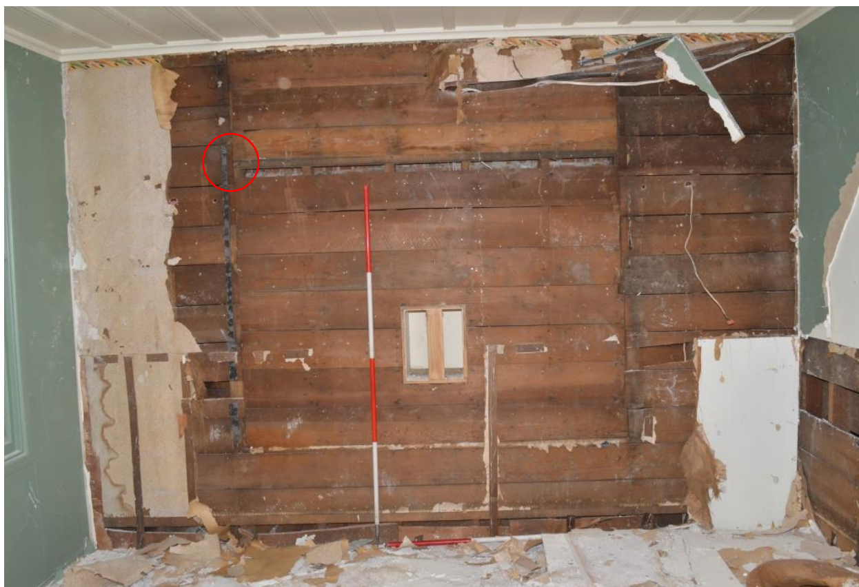
Figure 3.45. South wall of G04 showing blocked-up window, traces of wallpaper and hatch into the Phase 3 garage. Note the 1930-1950s wallpaper and frieze remains on the left-hand side of the photo (source: Clough & Associates, 2015)
