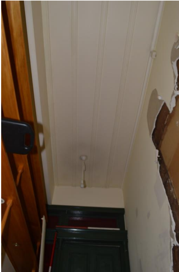
Figure 3.37. Board and batten ceiling in G02 (source: Clough & Associates, 2015)
