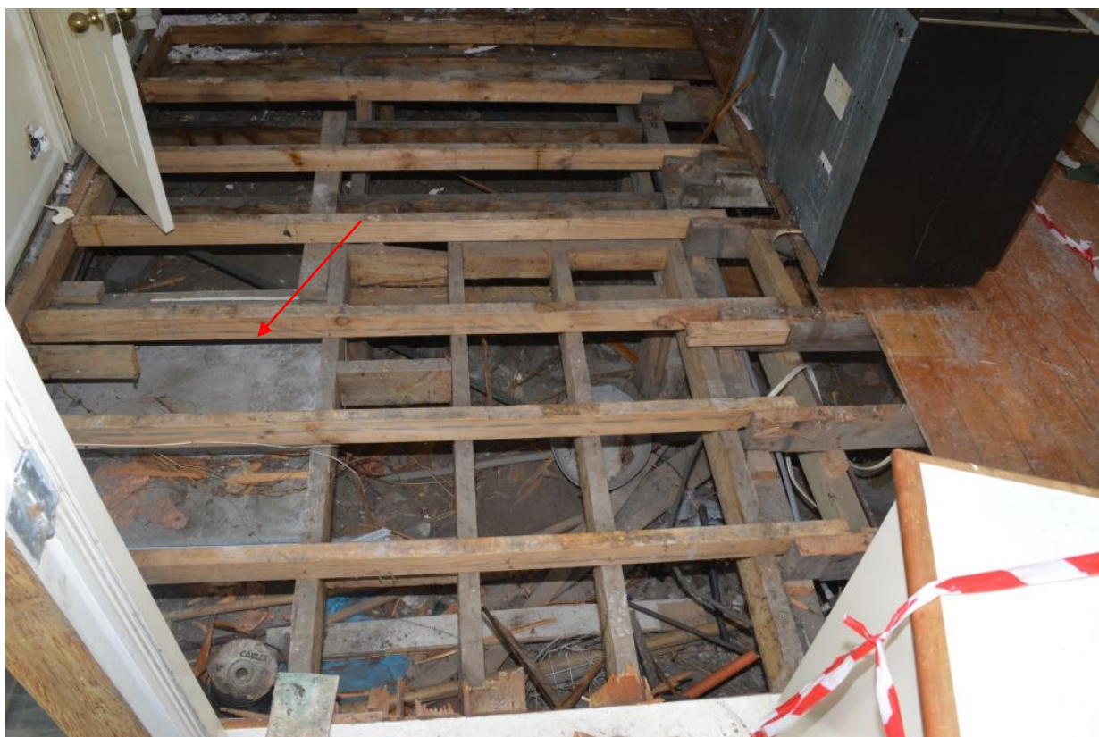
Figure 3.65. Looking south over G05c between G06 (door on left-hand side of photo) and kitchen island (on right). Note the concrete steps marked with red arrow and series of raised floor joists. The joists running north/southern (lower joists) are from Phase 5, the Phase 6 joists are aligned east/west (source: Clough & Associates, 2015)
