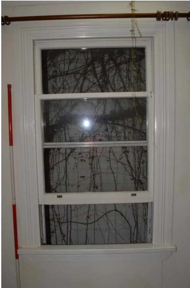
Figure 3.82. Double hung sash window with original architraves on eastern elevation of F05 (source: Clough & Associates, 2015)
