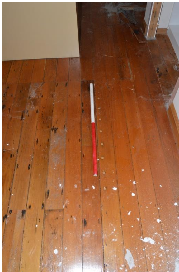
Figure 3.21. Photograph showing cut of spindles for a balustrade within original floorboards (source: Clough & Associates, 2015)
