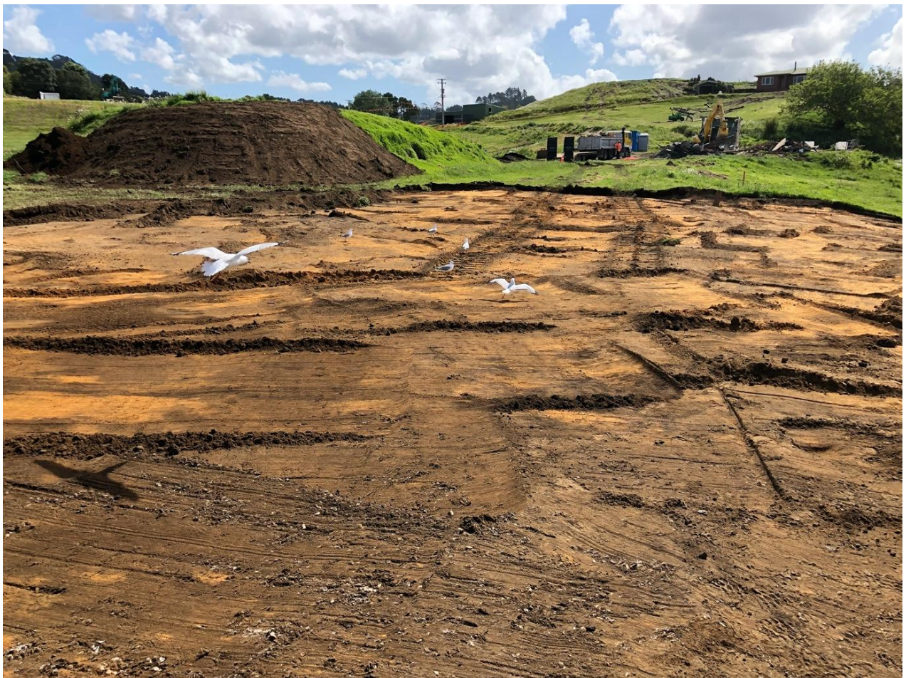
Figure 29. Overview of area stripped for the silt pond, facing west. Note redeposited shell in foreground close to site T11/1014
