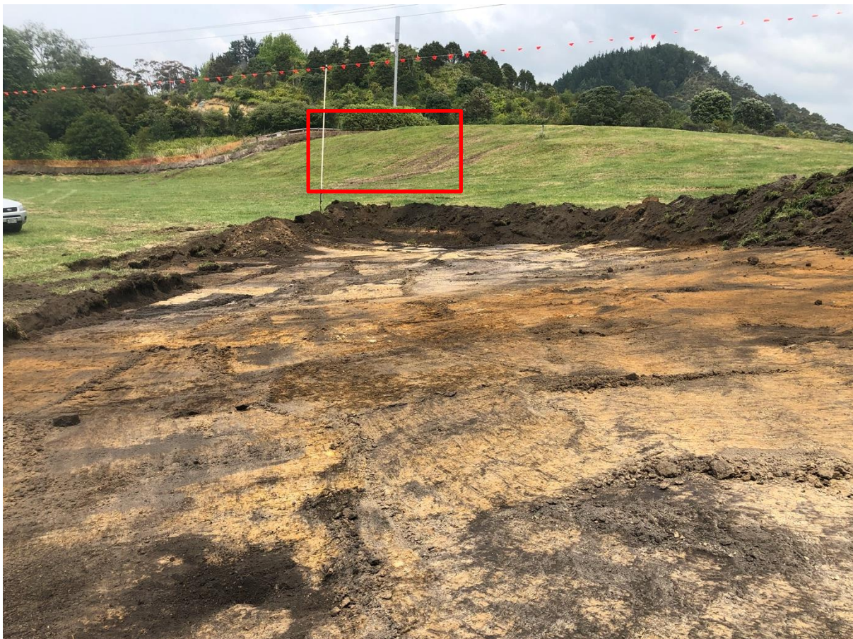
Figure 39. Topsoil strip in progress 18/11/2019 in Stage 2B area between sites T11/1014 and T11/2790, facing southeast – red rectangle shows location of midden 101
