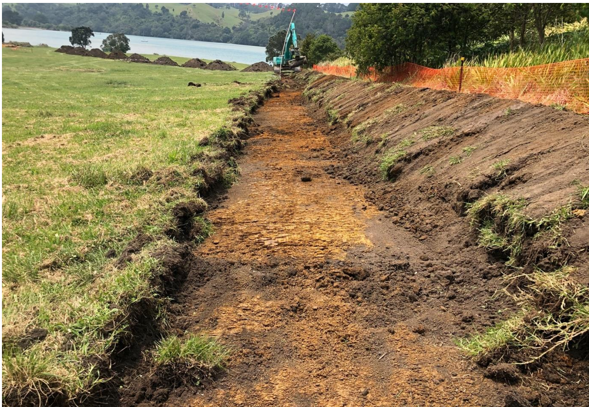
Figure 22. Topsoil strip in progress 18/11/2019 in Stage 2B area, facing northeast
