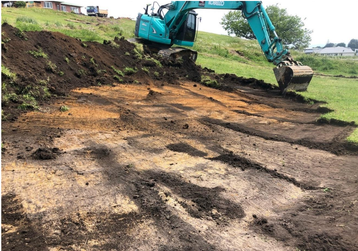
Figure 23. Topsoil strip in progress 18/11/2019 in Stage 2B area, facing north
