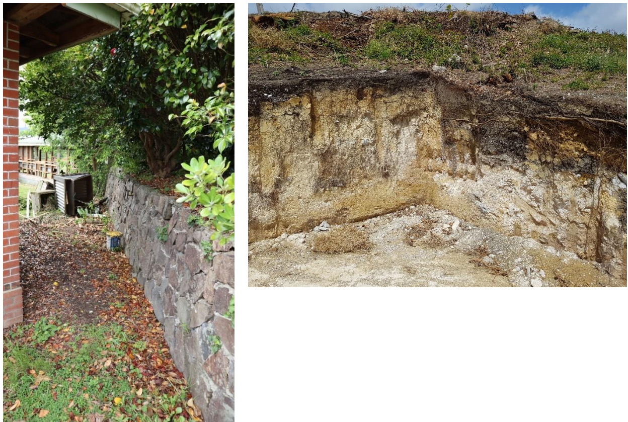
Figure 41. Retaining wall prior to house removal (left - November 2019) and subsequent removal (right – January 2020)
