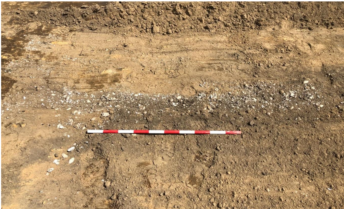
Figure 20. Shell backfilling irrigation pipe trench in Stage 2B area (scale interval 0.10m)
