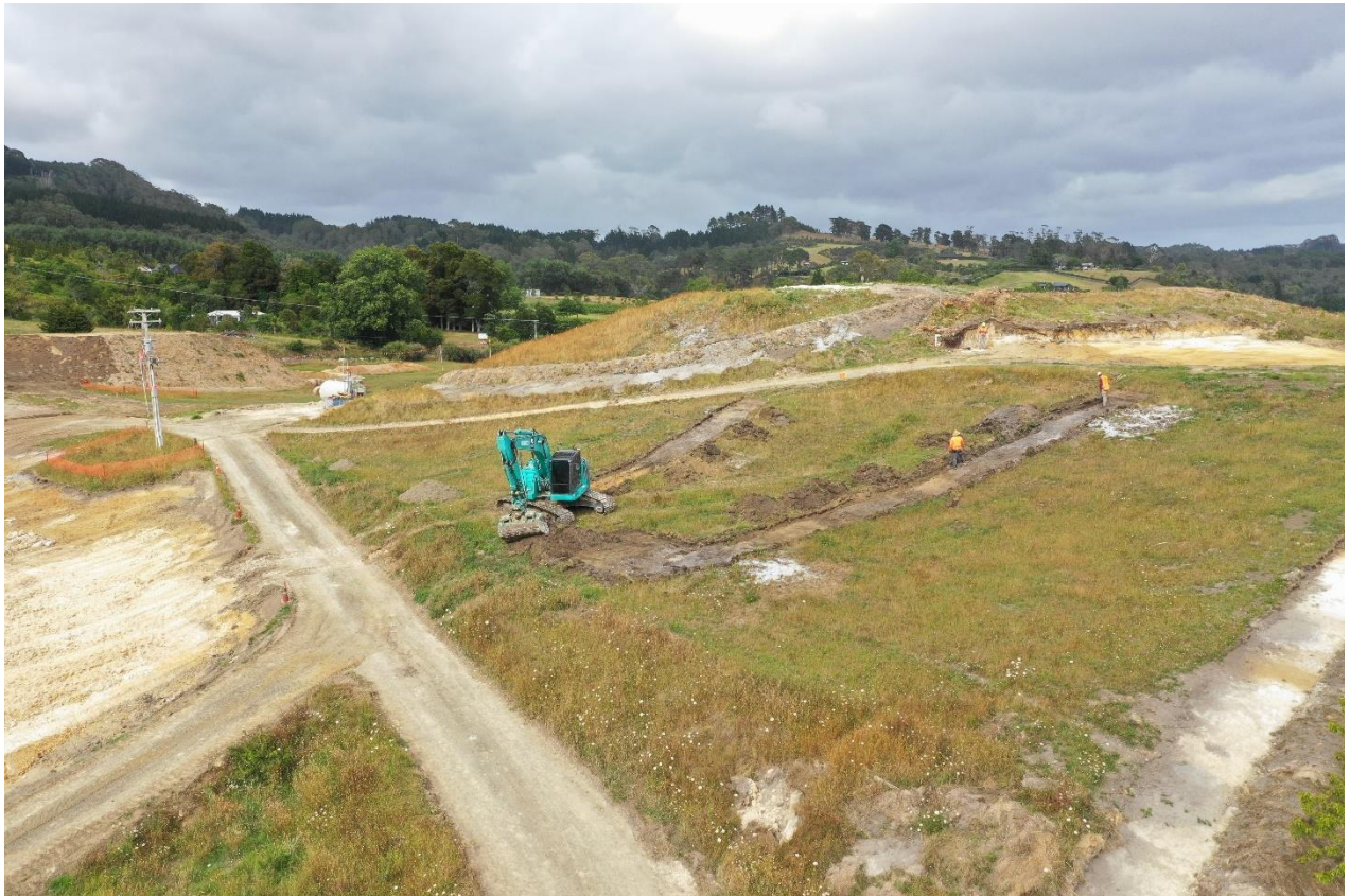
Figure 46. Drone photo showing initial test trenches (1 and 2) for site T11/1050, facing south
