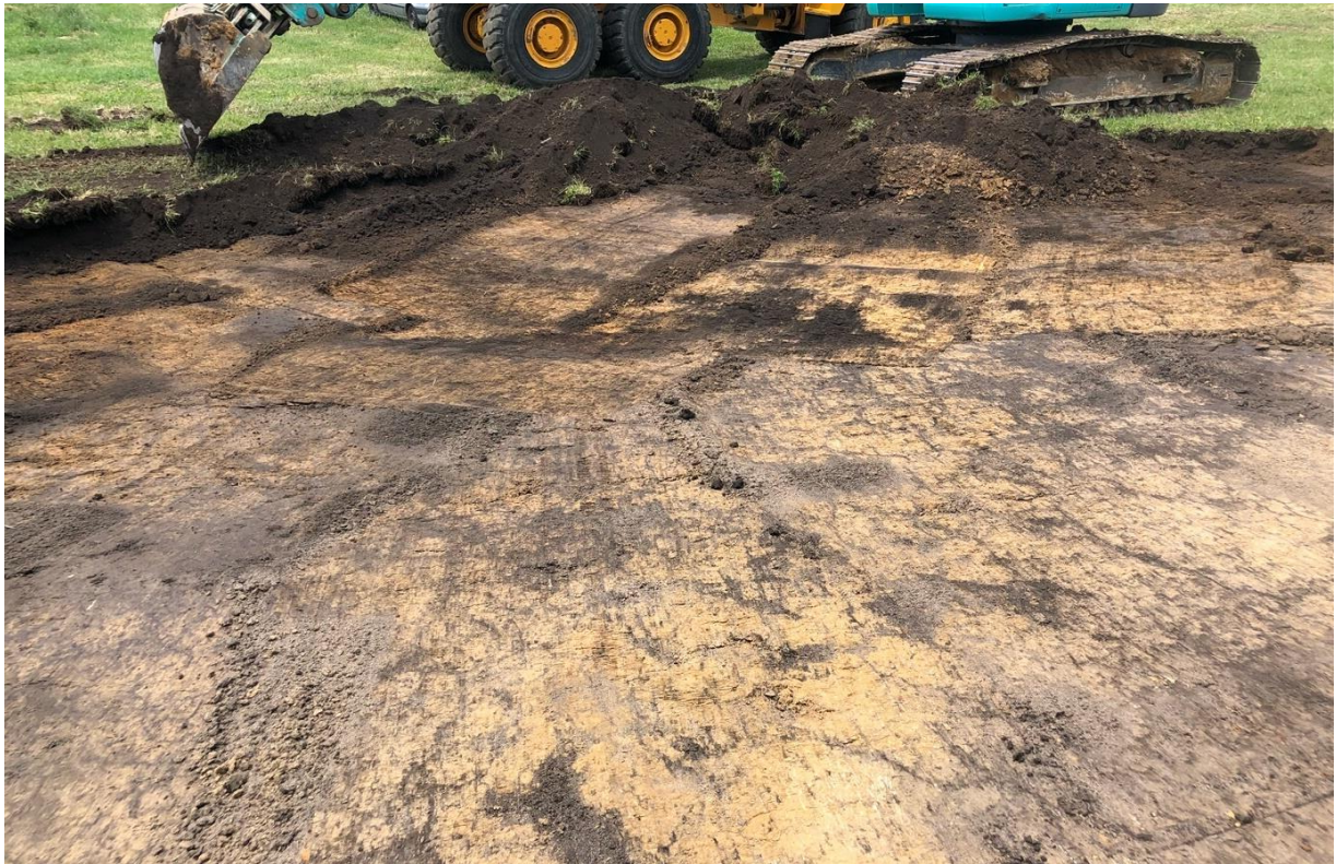
Figure 21. Topsoil strip in progress 18/11/2019 close to site T11/2790, facing north
