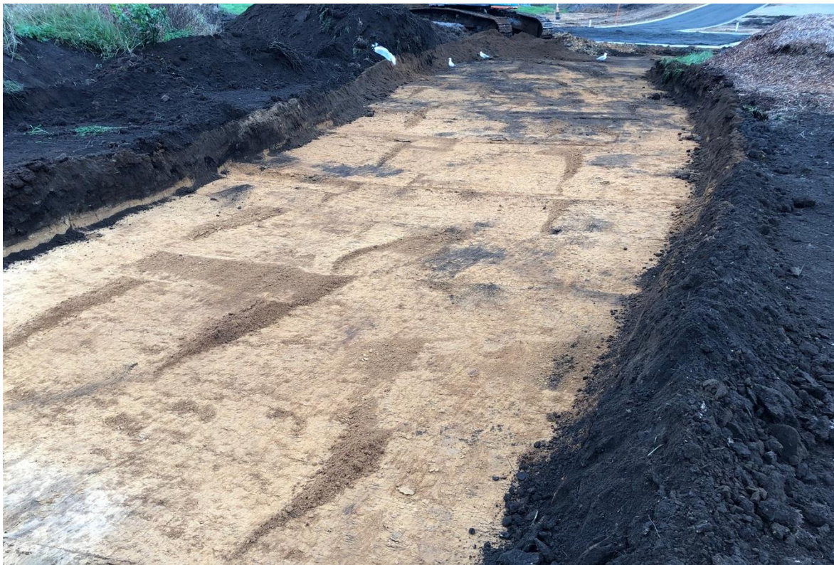
Figure 31. The two photos show the stripped overflow channel in the reserve area close to T11/1014
