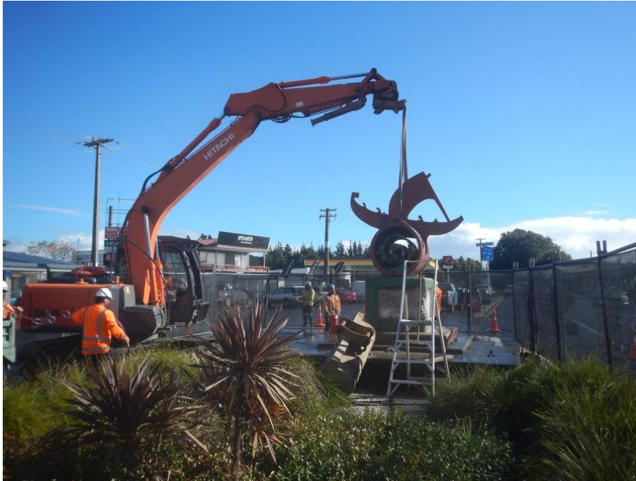
Figure 29. Slings holding the sculpture during removal from plaque plinth base
