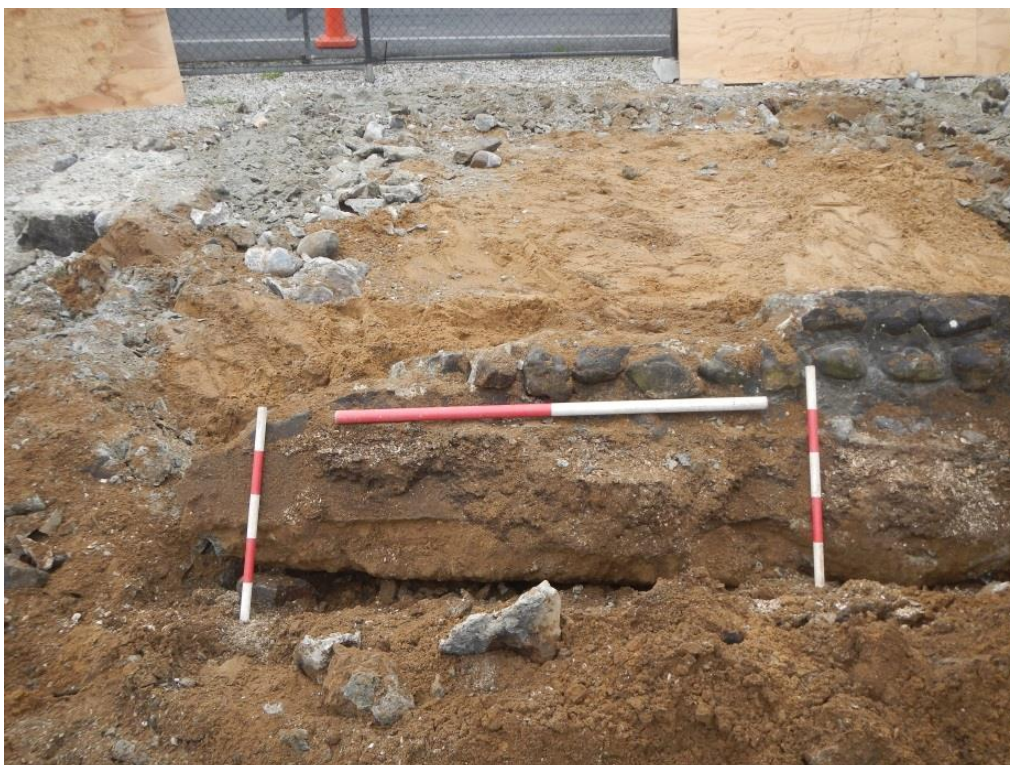
Figure 36. Removed section of concrete ring foundation showing timber shuttering pours. Scale intervals 0.5m and 0.1m
