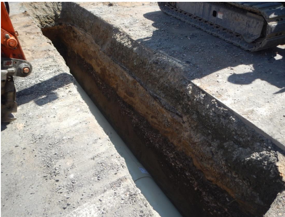
Figure 62. Insertion of sewerage pipe across SH10 showing east-facing section of stratigraphy and midden (056)
