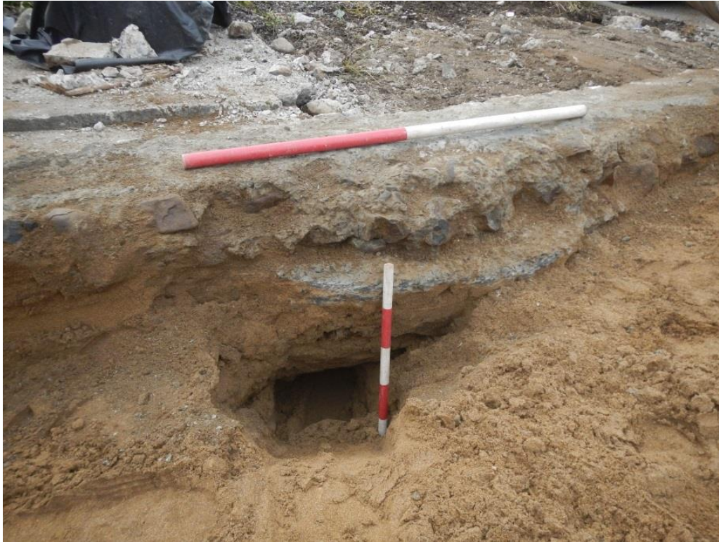
Figure 35. Exposed internal elevation face inside the concrete ring foundation of the monument. Scale intervals 0.5m and 0.1m
