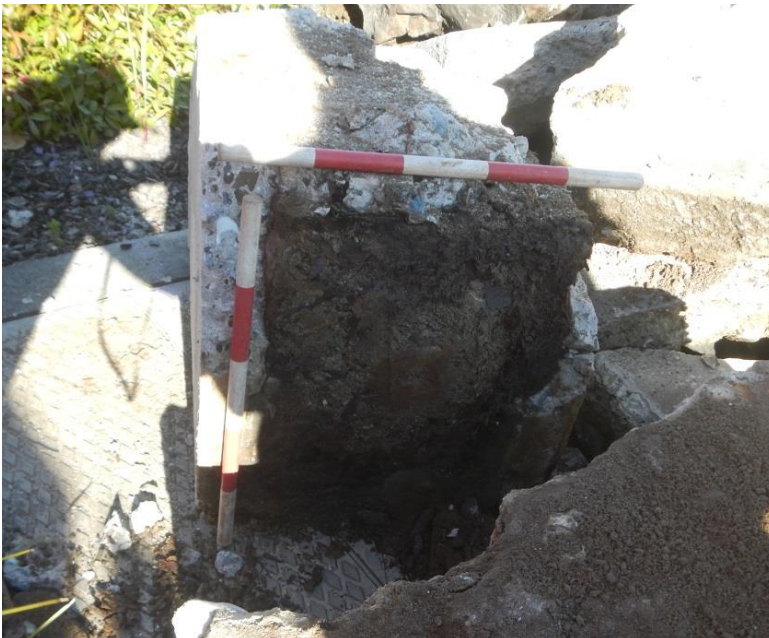
Figure 32. Exposed centre of the upper plaque plinth with the exposed rotten timber of the pou. Scale intervals 0.1m
