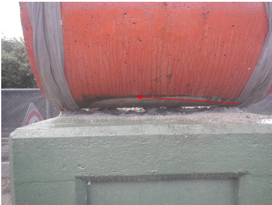
Figure 30. Sculpture after removal of concrete with exposed metal pipe arrowed in red
