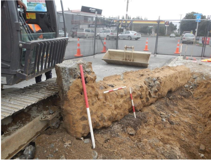
Figure 37. Removed section of ring foundation showing underside base and pour methods. Scale intervals 0.5 and 0.1m
