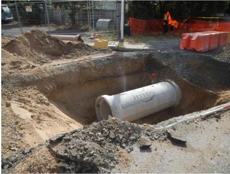
Figure 66. Looking northwards over stormwater trench (Trench 4) at Mamarua Road showing modern services running beneath road. The pipe is 750mm in diameter
