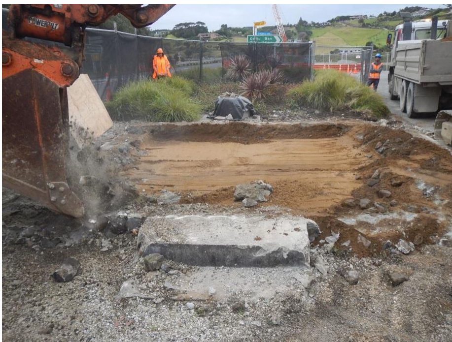
Figure 34. Looking eastward after basal plinth had been removed showing internal natural sand infill and concrete ring foundation
