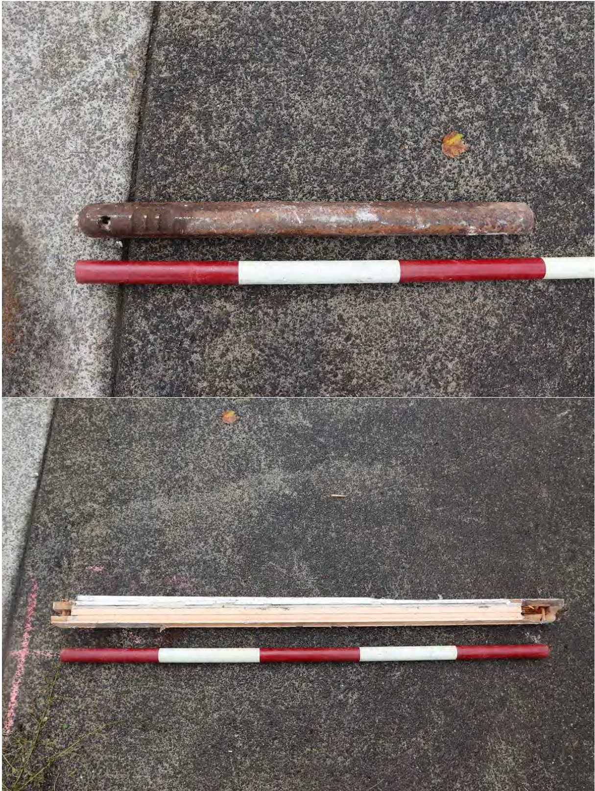
Figure 62. Top: sash window weight. Bottom: Section of window frame. Scale interval 20cm
