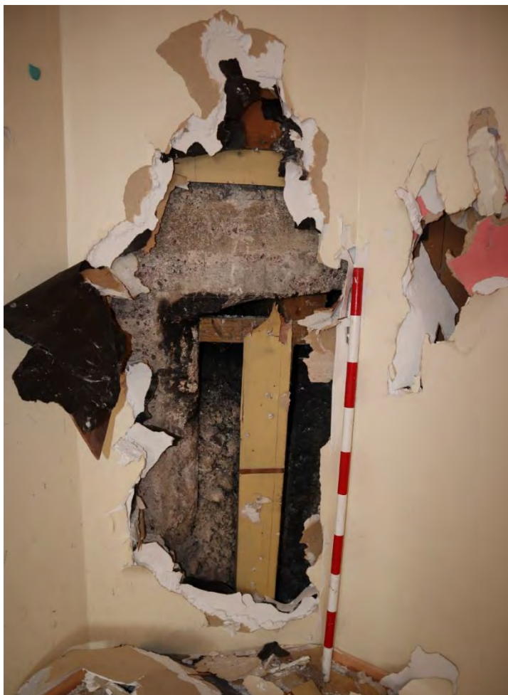
Figure 25. View of interior wood frame and concrete at back of main room (west)
