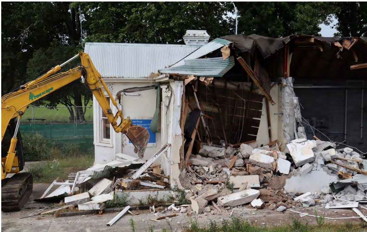
Figure 54. Demolition of the front facing portion of the structure beginning with the veranda and adjoining wall. Facing south
