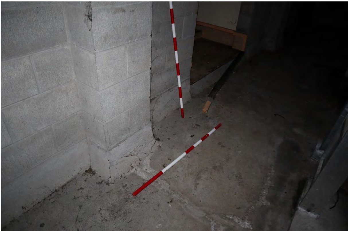
Figure 41. Moulded concrete fluted base on pillar
