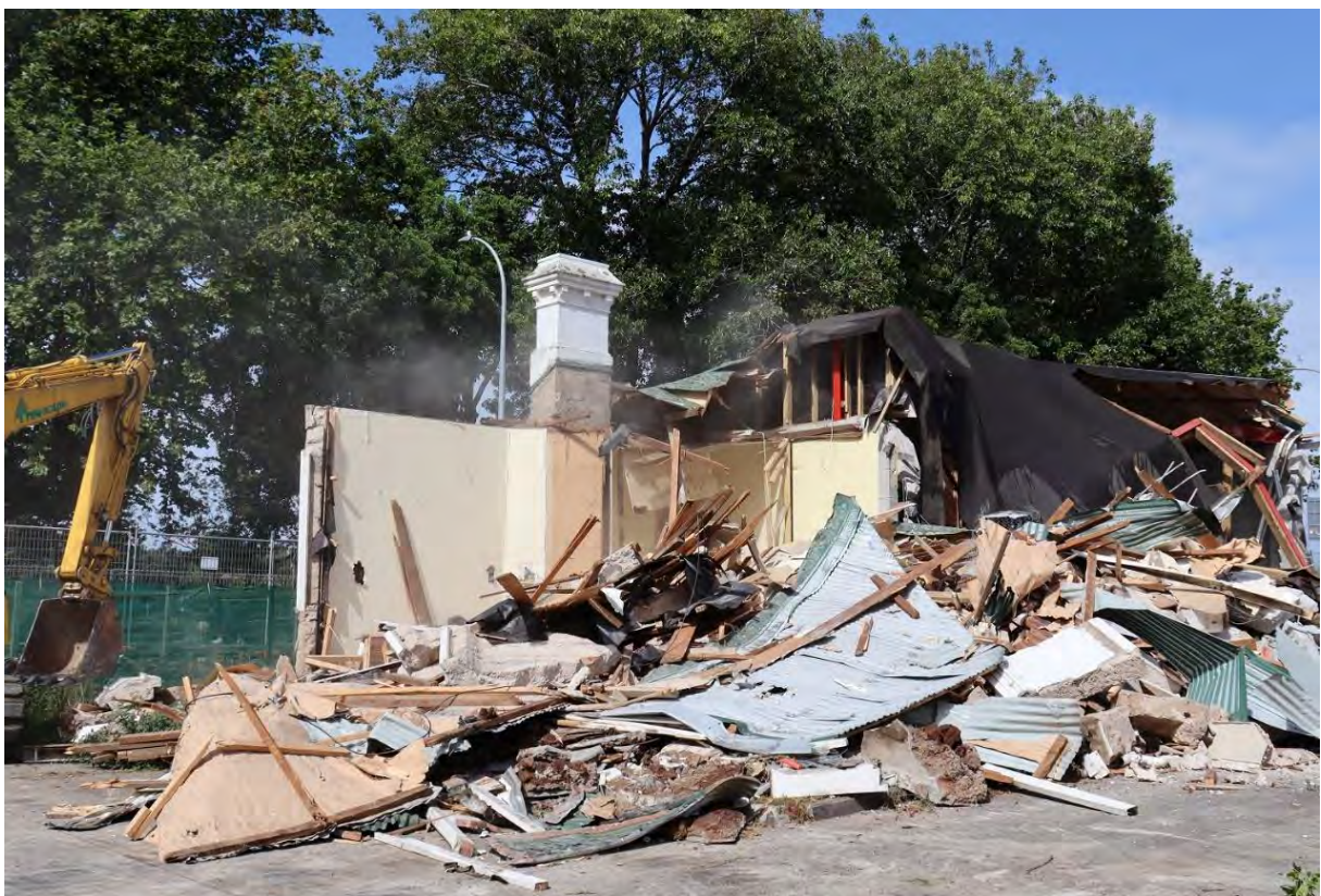
Figure 56. Demolition taking out the southeast portion of the structure (front facing portion). Note concrete chimney left standing, showing what it looked like from below the roof. Facing southwest
