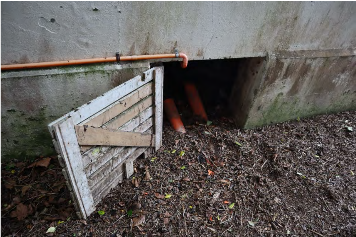
Figure 17. Access to underfloor beneath main room of building
