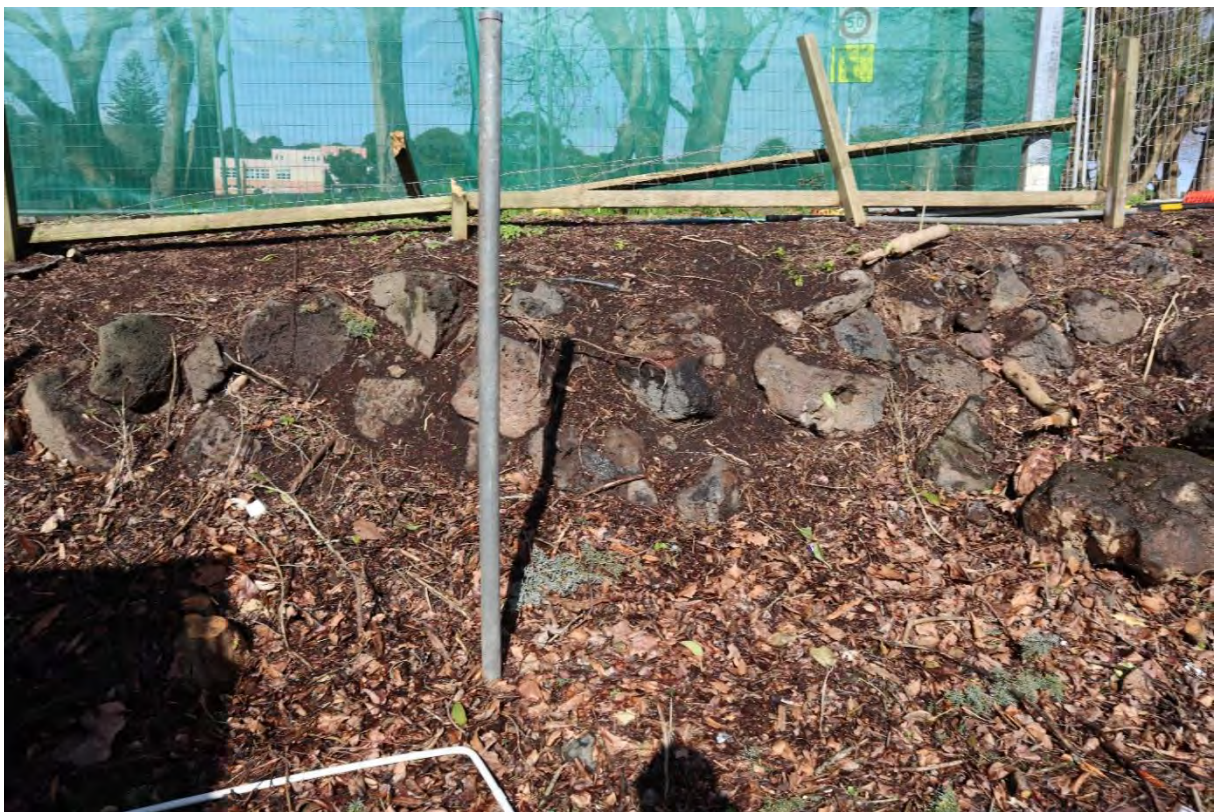
Figure 44. Exposed basalt retaining along the southern side of the property
