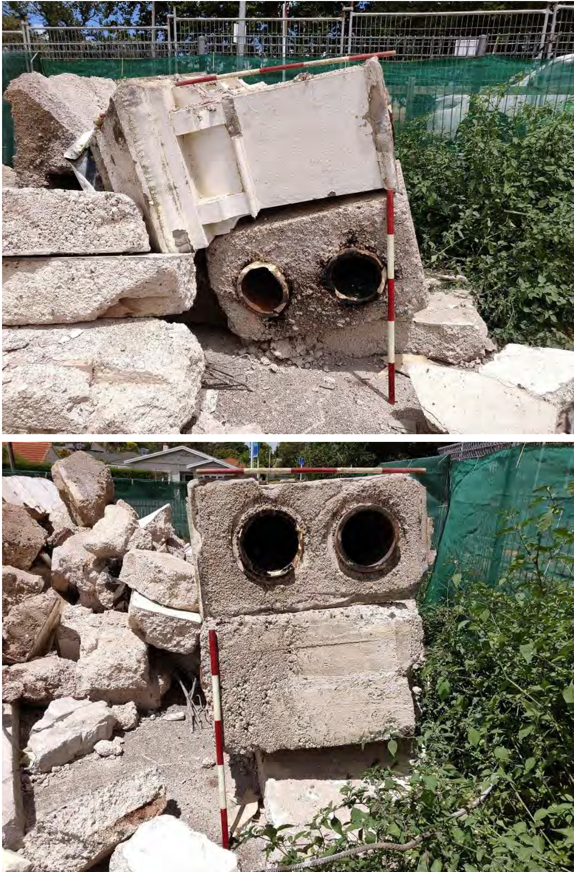
Figure 63. Sections of chimney showing ceramic flues encased in concrete. Scale interval 20cm
