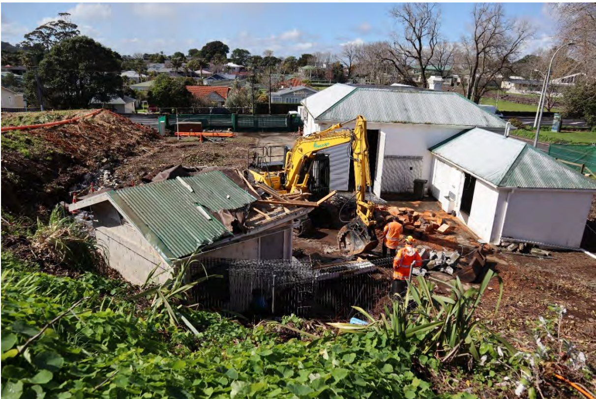
Figure 48. Demolition of the NW pump building showing roof removal (looking east)
