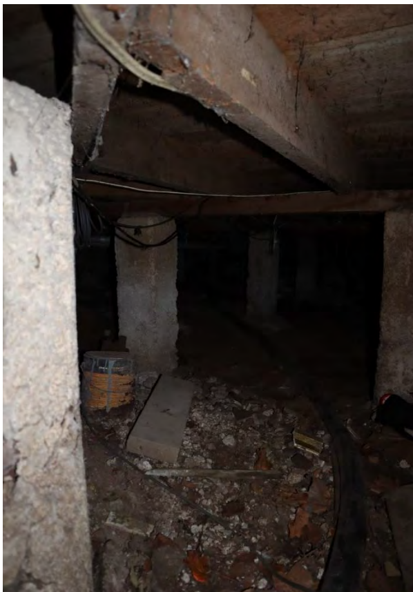
Figure 19. Photograph taken under the building showing concrete piles and floor joists
