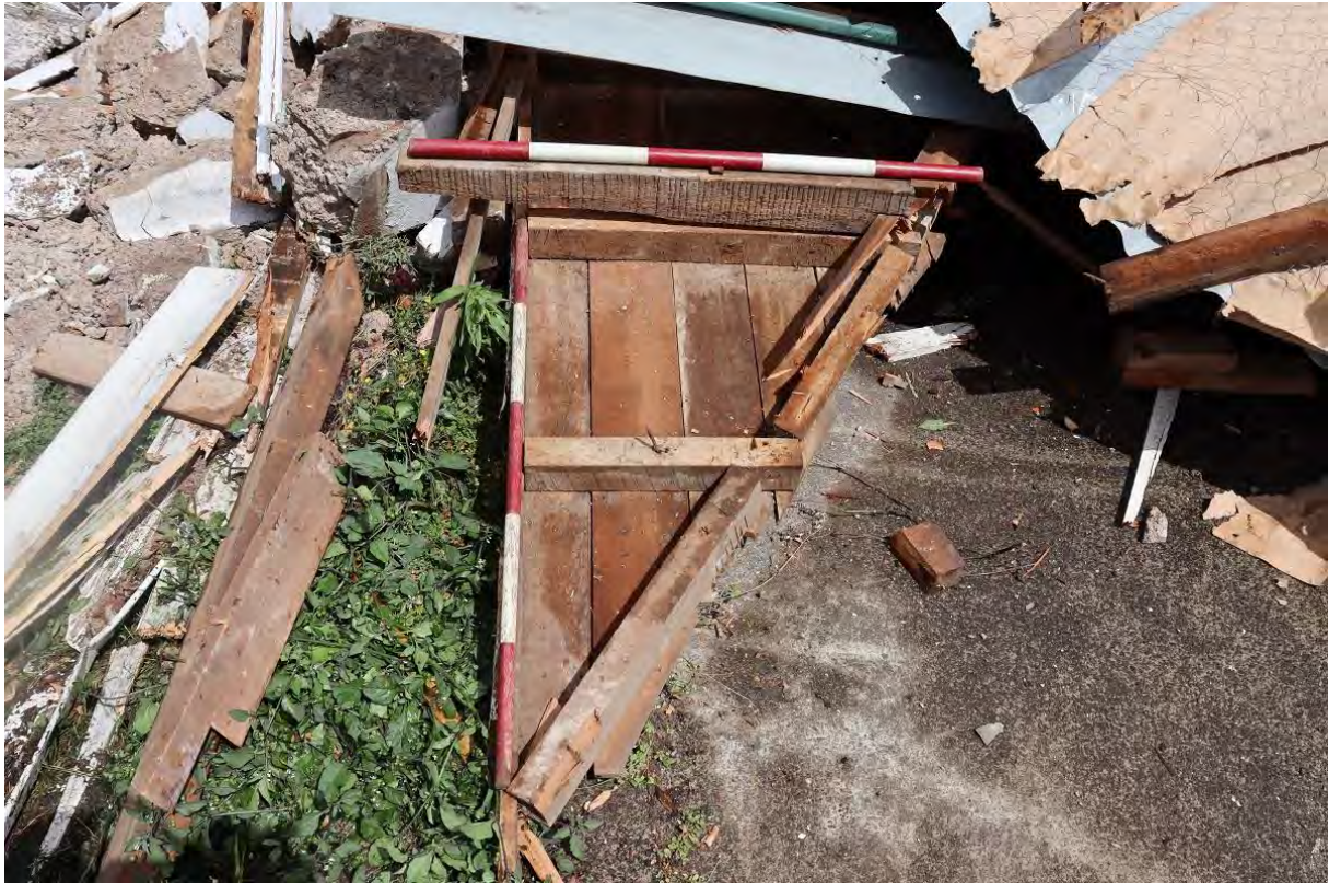
Figure 60. Section of timber gable from the front of the house. Scale interval 20cm
