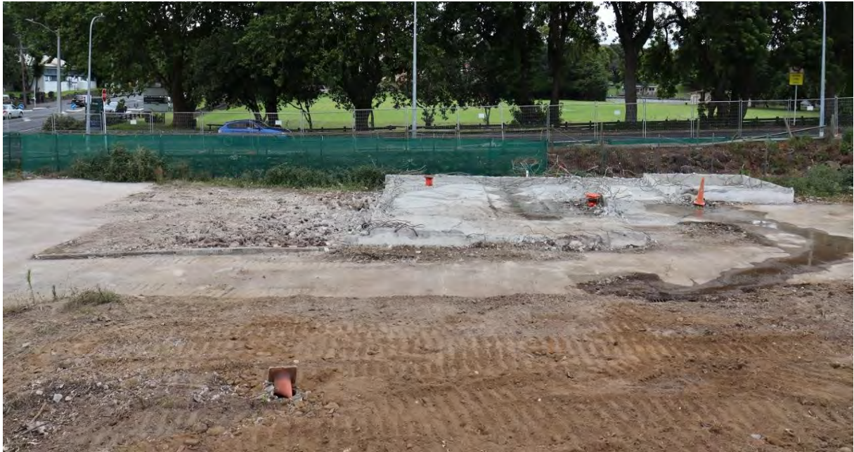
Figure 66. Demolition complete and material removed revealing concrete base. Note the pumphouse area is raised, with different concrete. Facing south
