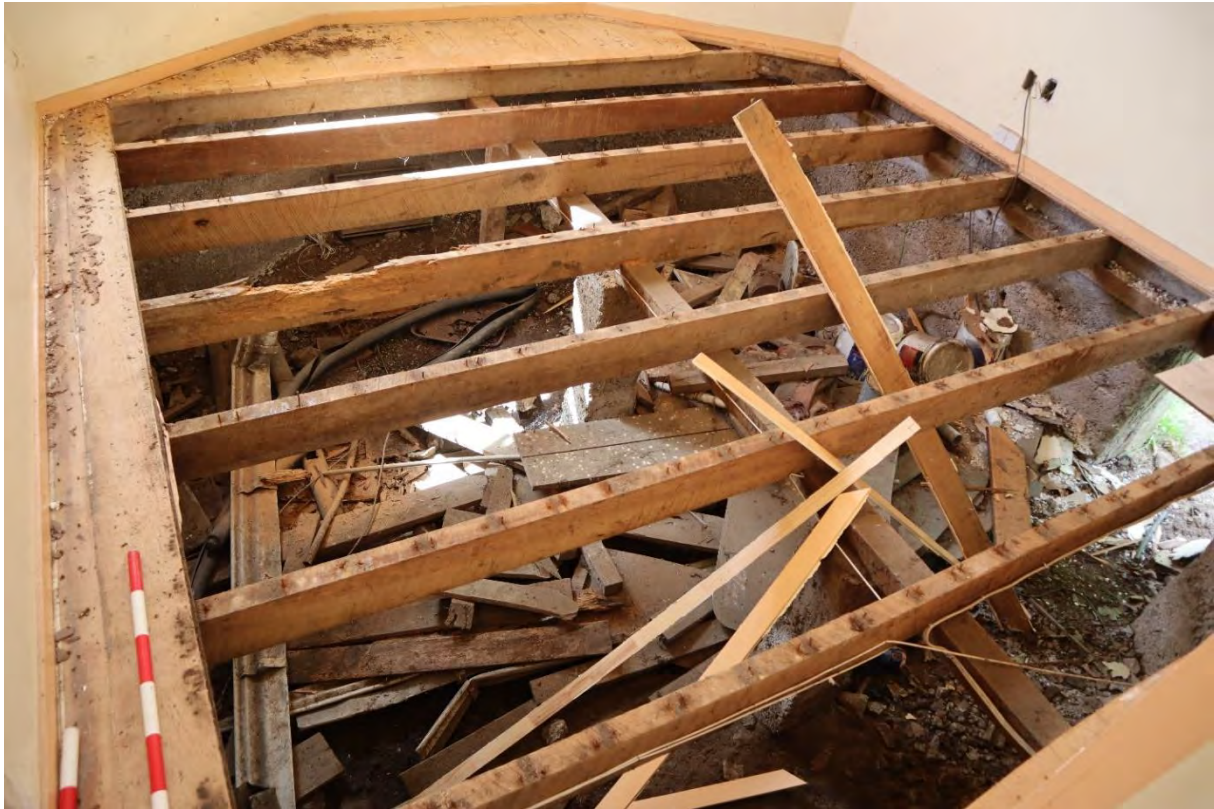
Figure 26. Floor joists and bearers exposed in main room
