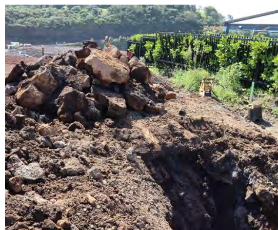
Figure 8-32. Pipe trench towards quarry showing basalt blocks from trench
