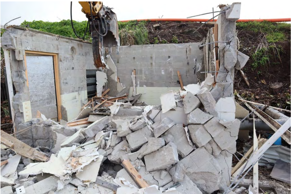
Figure 50. Concrete block exterior structure during demolition
