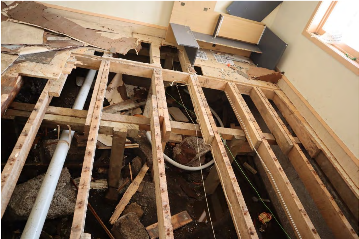
Figure 34. Exposed bearers and joists in north room with plywood flooring
