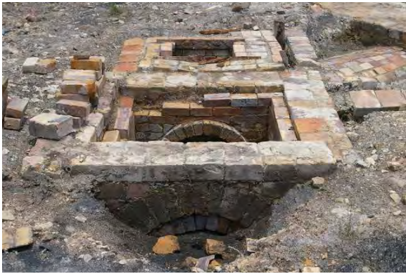
Figure 99. S7 showing blocked arch in front, open arch behind leading to S7b; flue to K5 on right. Looking south
