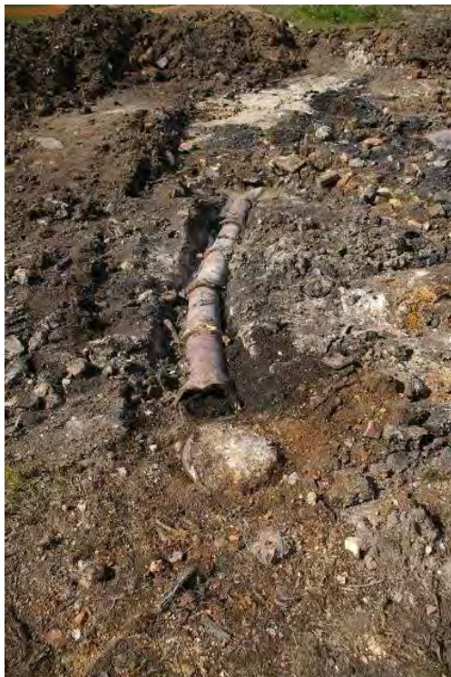
Figure 75. Drain 1 terminating at foundation pile in service floor for K3
