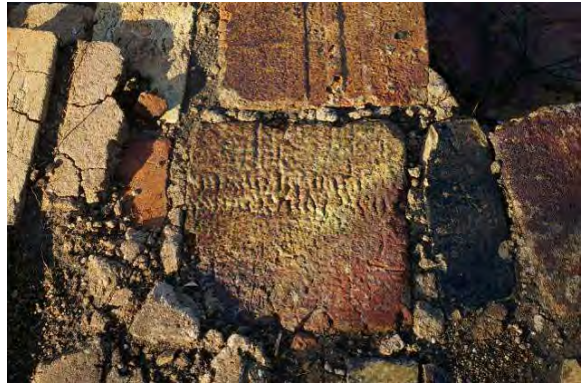
Figure 59. Example of fire damaged square brick reused in kiln wall, and soft buff coloured mortar
