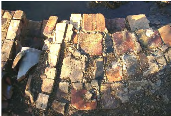
Figure 55. Use of mixed bricks including extruded squares and narrow bricks near firebox, K1
