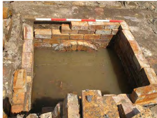
Figure 100. Showing the arch through the inner skin and main wall of S7a to S7b
