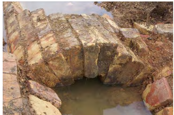
Figure 115. Double arched bricks of K9 flue
