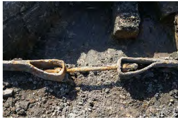
Figure 90. Adjustor bolt for iron strapping, S5
