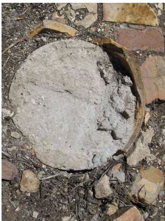
Figure 122. Foundation pile, ceramic pipe filled with concrete and small amounts of shell
