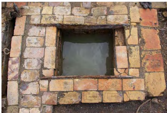
Figure 97. S7 close up of flue control box with recycled DRURY bricks in firebox – steel gate with lifting hook on left
