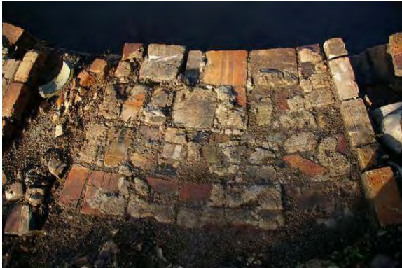
Figure 58. K1, mixed wall bricks and mortar between two fireboxes
