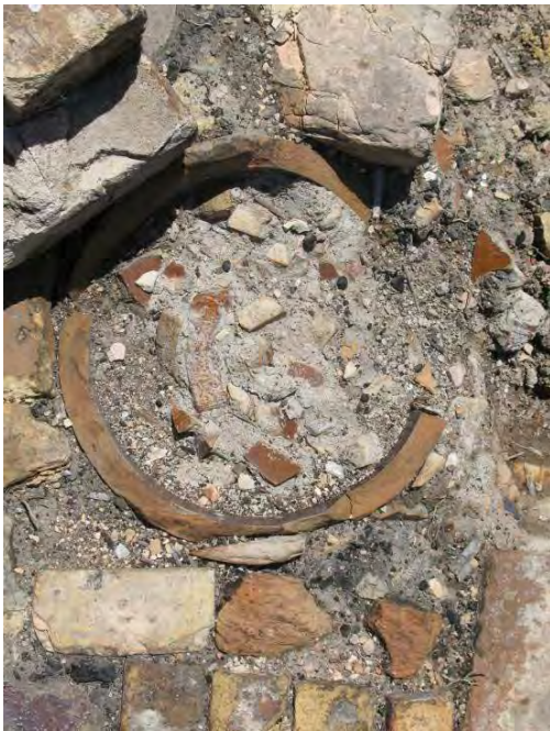
Figure 120. Foundation pile with ceramic aggregate
