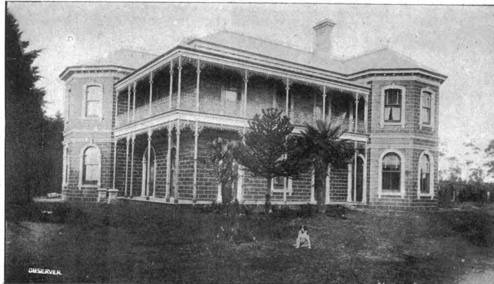
R. O. Clark's Private Residence, Hobsonville.—Foundations, walls, and partitions built entirely of squares (No. 134)
