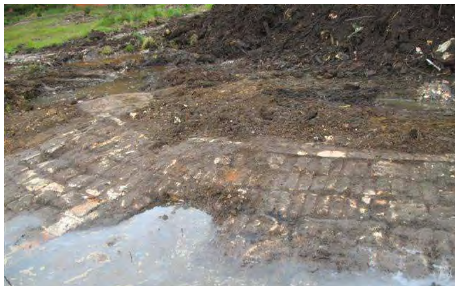
Figure 102. Loose inner 'skin' of S7, machine pressed bricks with one KAMO brick in stack wall
