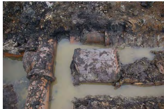
Figure 76. Junction of drains D2 and D3
