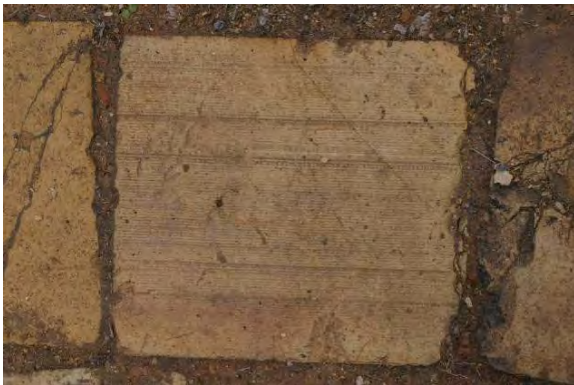
Figure 126. Extrusion dye marks from tooling
