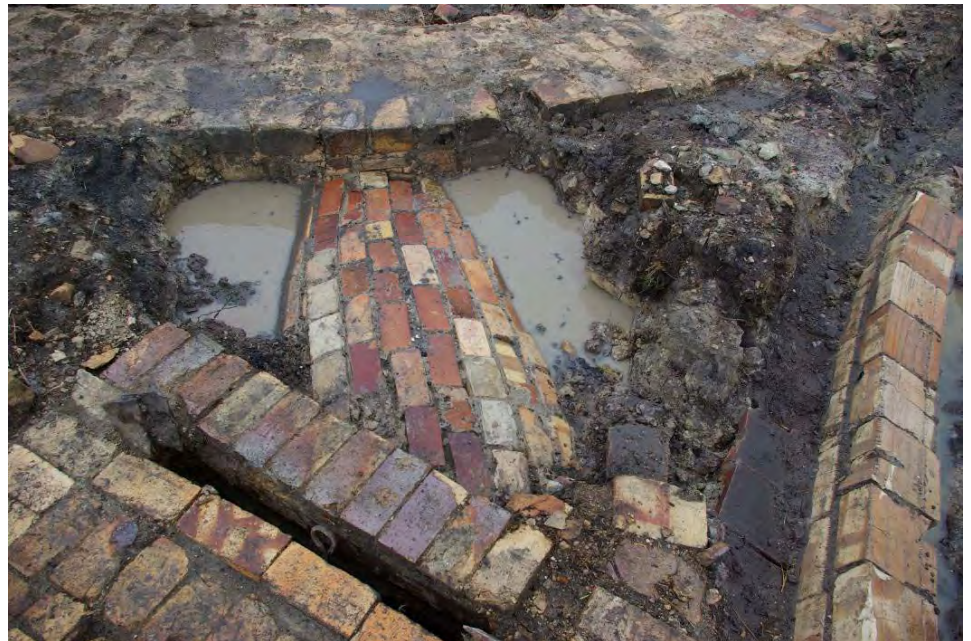
Figure 95. Juxtaposition of S7b gate controlling flue, flue and K5 at top. F1 on right (square bricks on long hollow glazed ceramic blocks). Looking west
