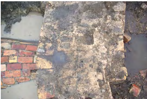
Figure 73. Soft buff sandy mortar wall of K5, junction of flue
