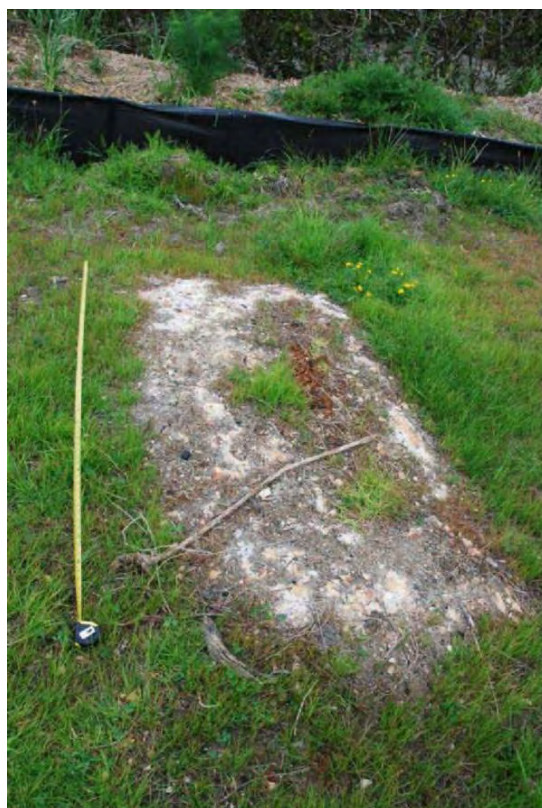
Figure 123. Concrete foundation pile near foreshore, with wooden inset (from Geometria 2007)
