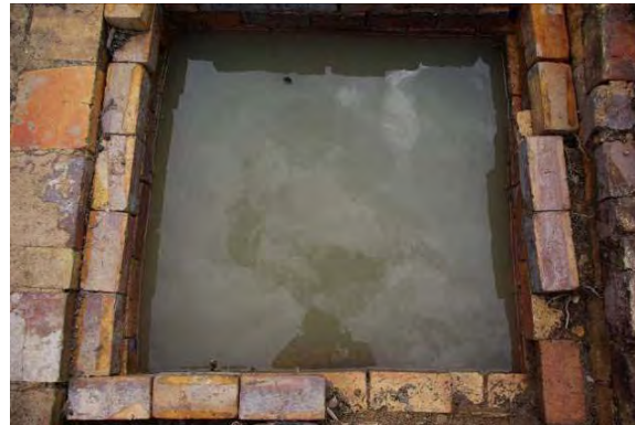
Figure 102. Loose inner 'skin' of S7, machine pressed bricks with one KAMO brick in stack wall
