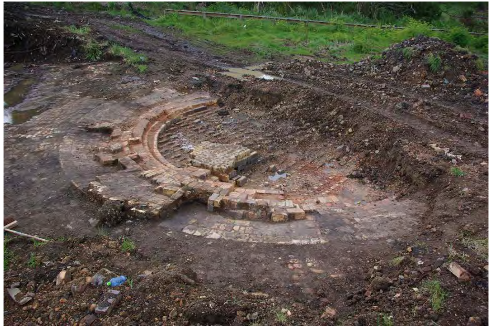
Figure 104. Kiln K7 with part of chequer floor; looking east
