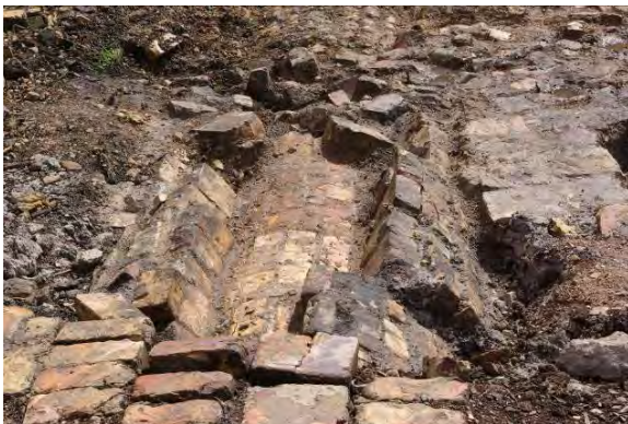
Figure 60. K1 close up of double skinned flue
