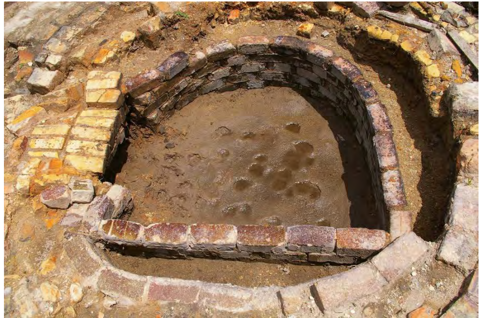
Figure 91. Stack S5 inner skin of extruded glazed bricks; arched flue on left; looking southwest
