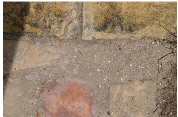
Figure 93. Mixed shell cement mortar of foundation, S5
