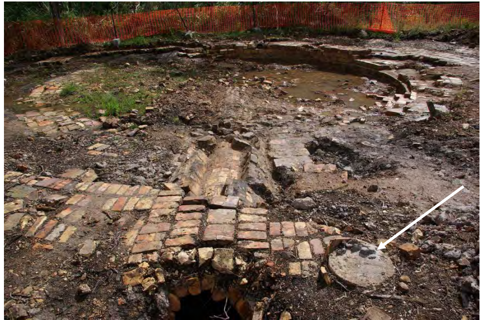
Figure 54. Kiln K1 showing kiln and flue; concrete filled ceramic pipe foundation pile (arrowed); looking north
