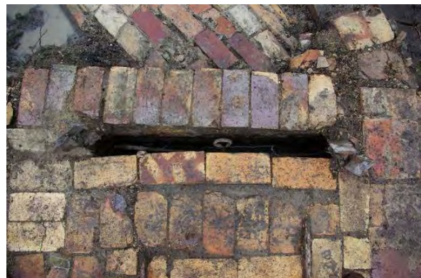
Figure 98. Close up of gate controlling air flow from K5. Iron guides for the gate once extended above the present level but have been cut off
