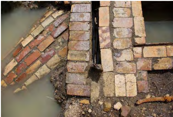
Figure 101. Junction of flue from K5 and gate to S7
