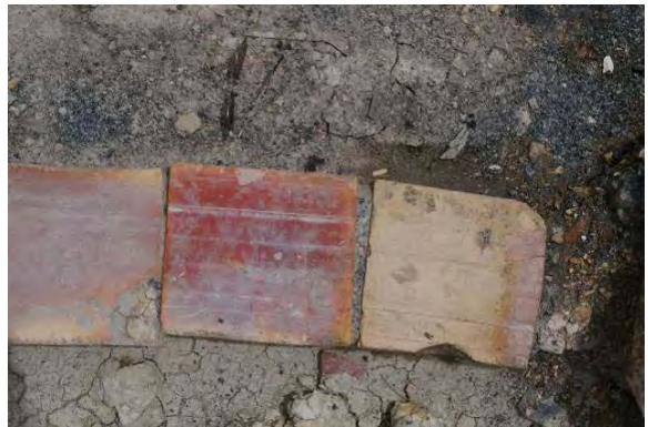
Figure 127. Square bricks with dye tooling marks
