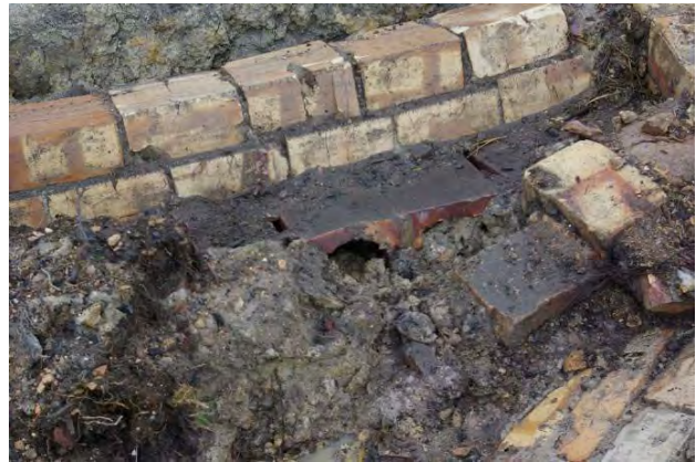
Figure 86. Section view of F1 showing layer of hollow ceramic blocks overlaid by double course of square double sized bricks
