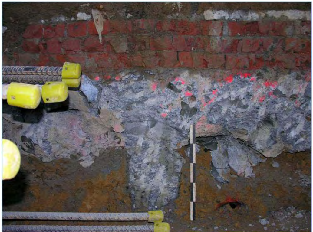
Figure A9.14. Concrete footing with piles beneath along the front of the four story building fronting Victoria Street (C', Figure A9.5)
