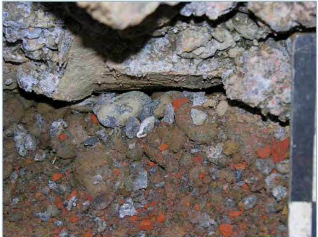
Figure A9.11. Round gravel and pebbles with sea shell from poorly cemented aggregate forming part of the concrete foundation footing (C, Figure A9.5)
