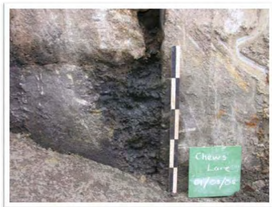
Figure 25. Concrete blocks showing the marine deposits of muddy sand and round gravel sandwiched between the blocks and the foundation wall of an existing building. The bottom of the trench is recently-poured concrete
