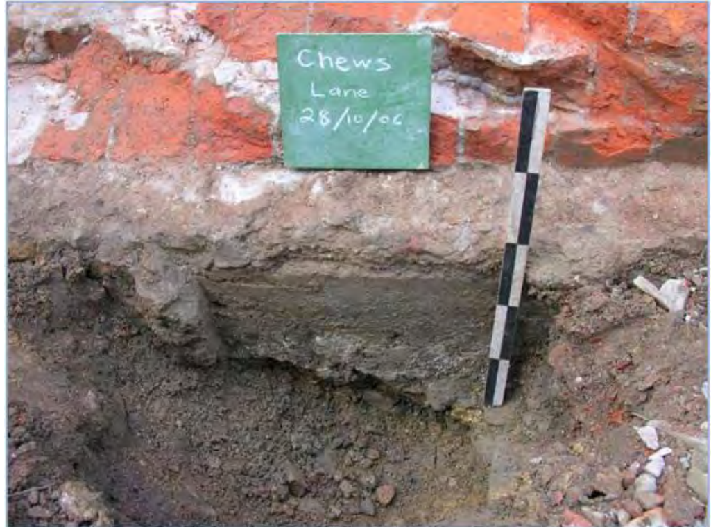
Figure A9.16. Concrete footing of the foundation shown in Figure A9.15 showing a flat surface that is probably the result of wooden formwork. Whether the formwork was part of the original foundation construction or dates from when the foundation was strengthened is not known
