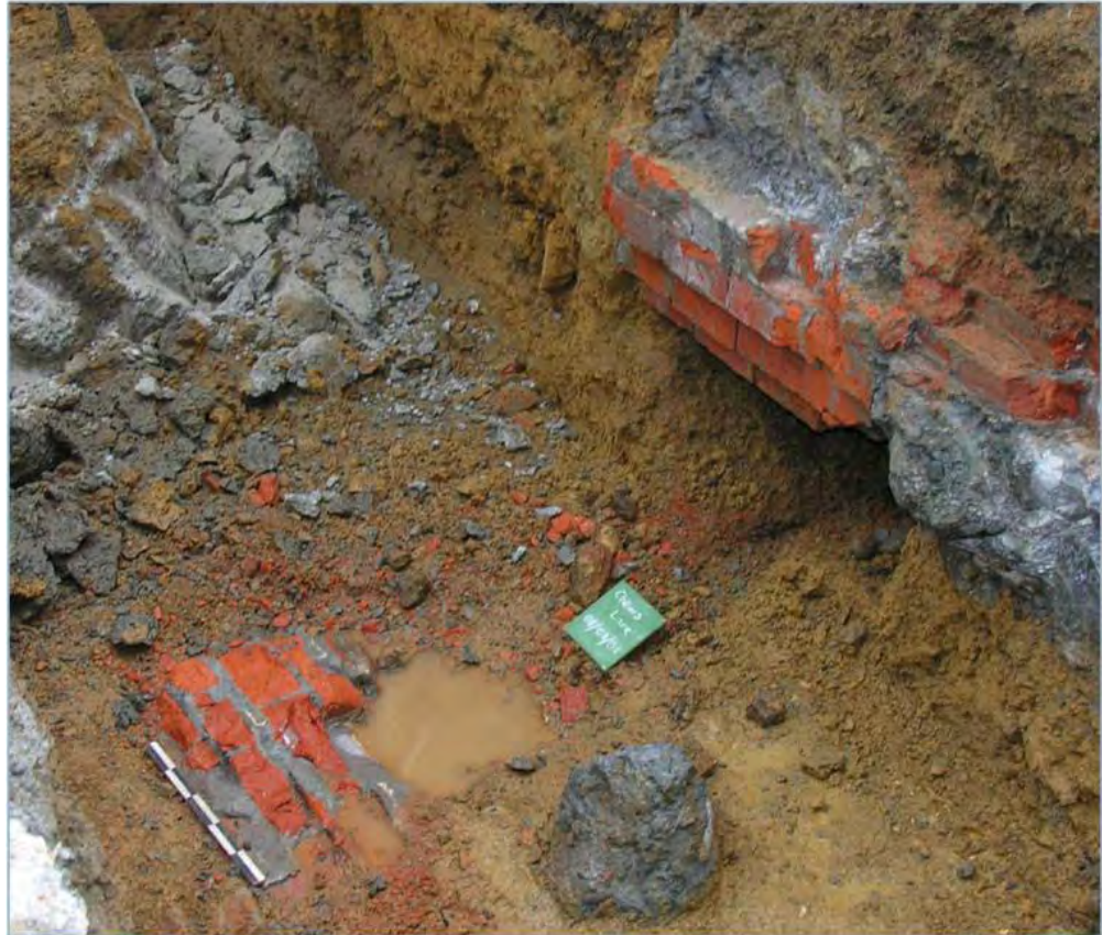
Figure A9.9. Brick arch (at right) after removal of the left hand section of curve, and the arch support pile (bottom left)
