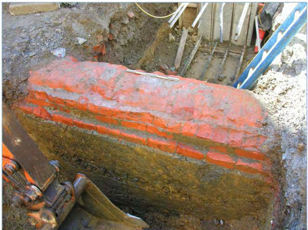
Figure A9.12. Foundation with a massive concrete footing and bricks above (B, Figure A9.5). Note the rounding of the brick upper surface, probably a result of demolition of the wall in preparation for a new building
