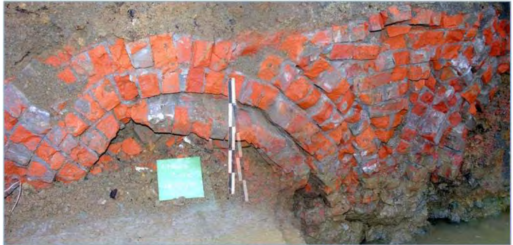
Figure A9.7. Brick arch foundation along the south end of the Victoria Street road frontage (A, Figure A9.5) (image compiled from two overlapping photographs). Note the infill of brick between the complete arch and the next arch at the right hand side of the photograph. Scale = 50cm
