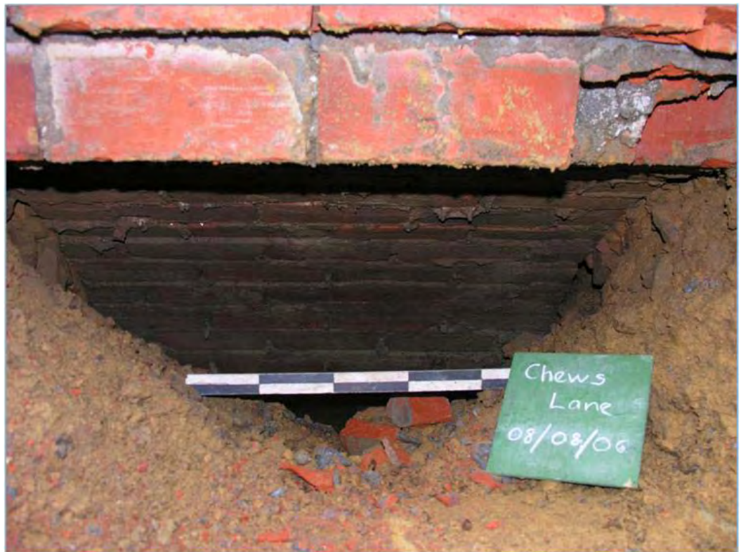
Figure A9.8. Underside of brick arch foundation, along the north side of the three story building fronting Victoria Street (A', Figure A9.5)
