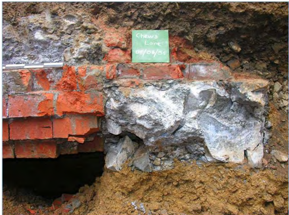
Figure A9.10. Brick arch foundation (Figure A9.8) with the younger, abutting concrete footing and bricks of the foundation of the building to the north. Concrete aggregate included angular stones more than 10cm long, and round beach gravel and pebbles (See Figure A9.11)
