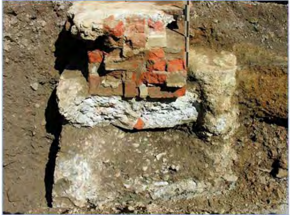
Figure A9.21. Concrete footing and brick work of external wall of building at D, Figure A9.6, on the Willis Street road frontage. The original footing is the lighter-coloured concrete immediately below the bricks. The slightly darker concrete below the light coloured concrete, and to the left and right of the bricks, is later and probably to strengthen the foundation below the building frontage when Willis Street was widened
