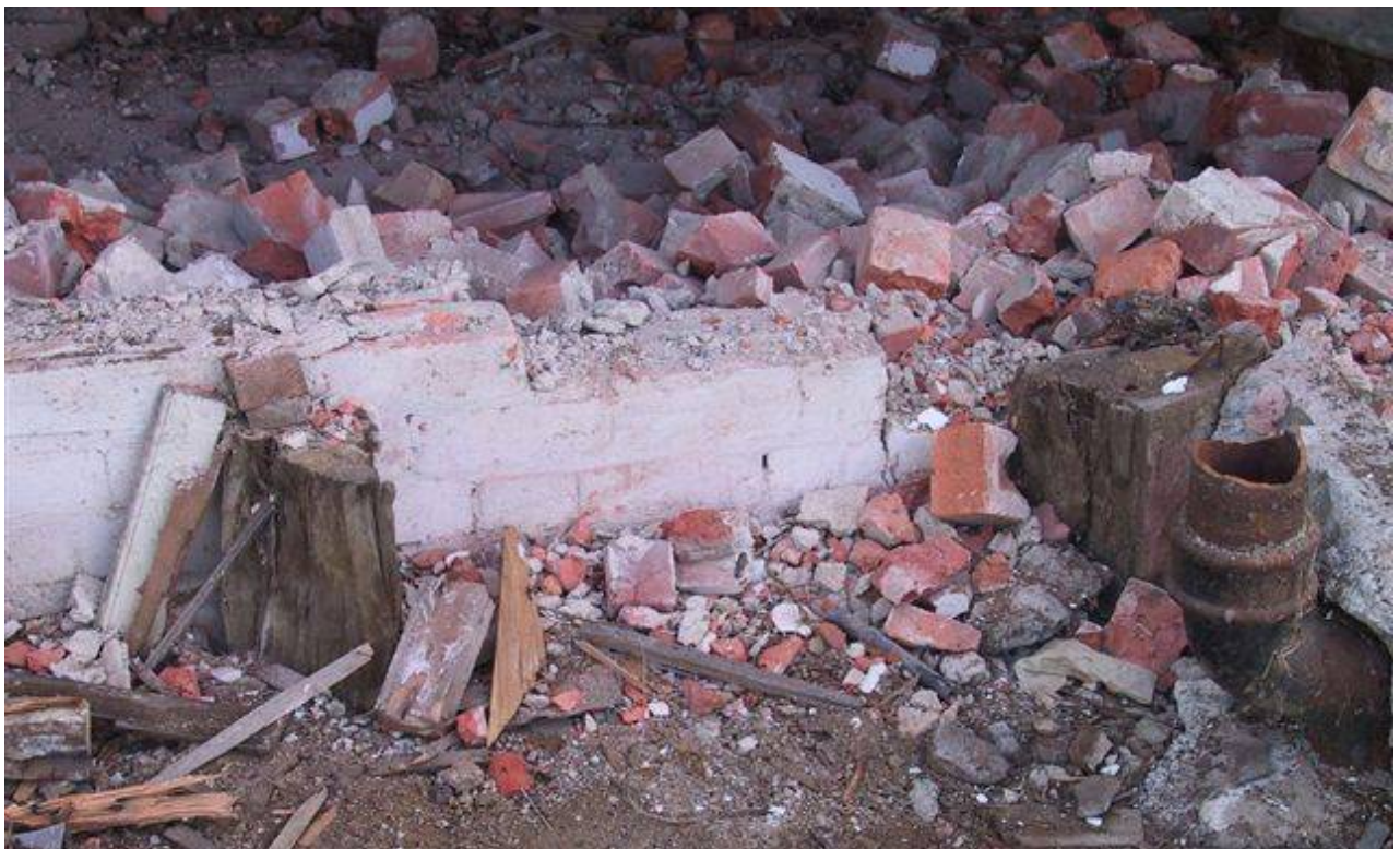
Figure 60. Wooden piles in southeast corner of the house outside later brick foundations
