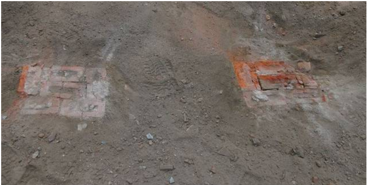
Figure 58. View of remnant brick piles under the main part of the house
