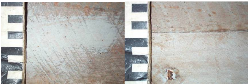
Figure 30. Circular (left) and banded (right) saw marks on kauri floorboards
