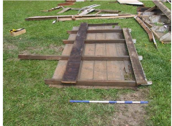
Figure 36. Ceiling of original cottage (topside)
