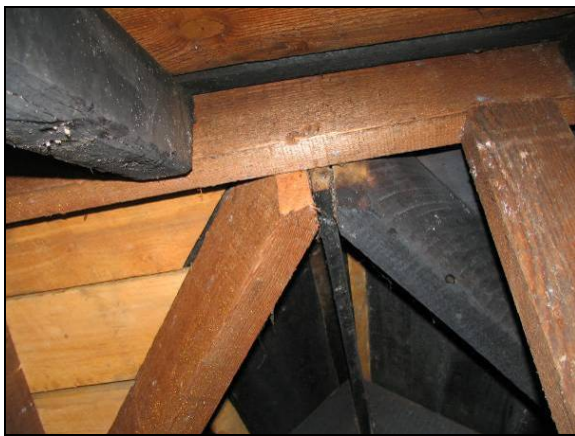
Figure 22. Inside the roof showing use of burnt beams that survived the fire and reconstruction
