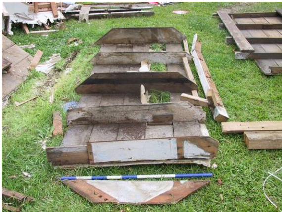
Figure 37. Reconstruction of ceiling elements and support of original cottage
