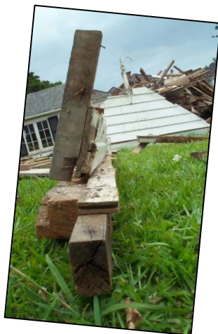
Figure 39. Connection of roof to wall studs in cottage
