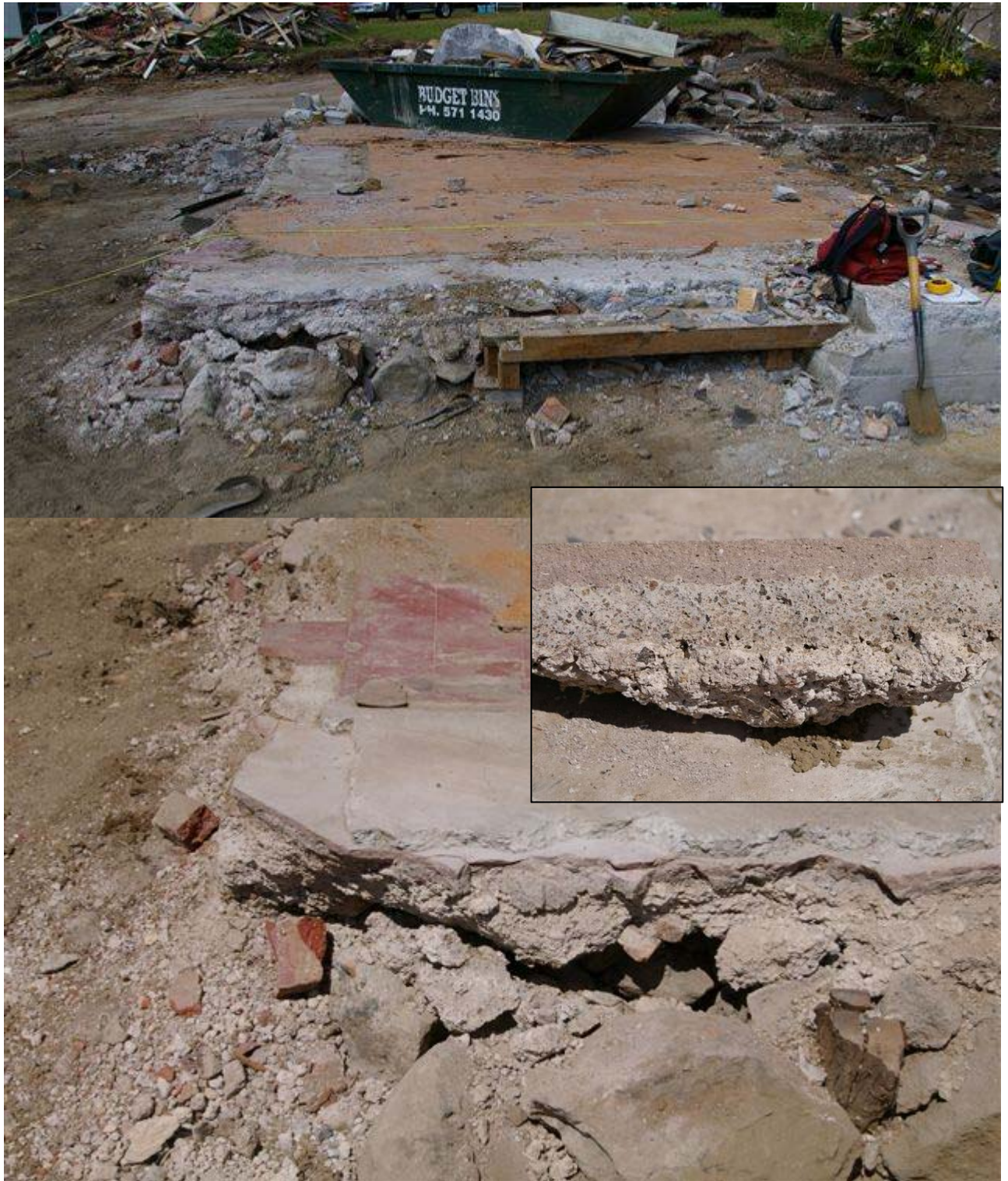
Figure 61. View of concrete pad from the kitchen area showing layers of early concrete and later tiling.
