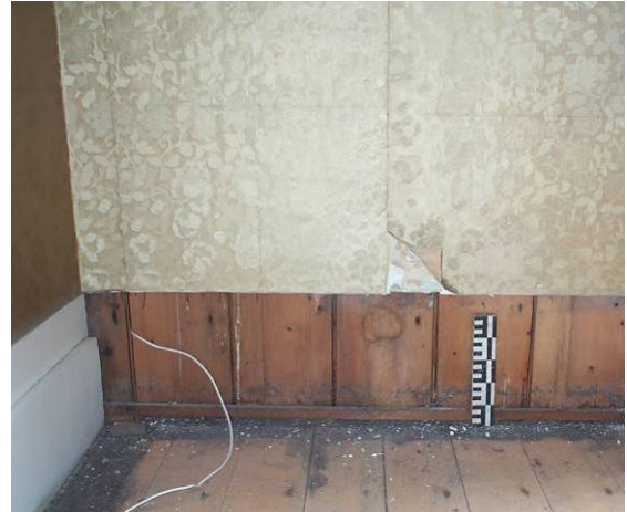
Figure 26. Wallpaper over vertical kauri sarking in dining room (G14)
