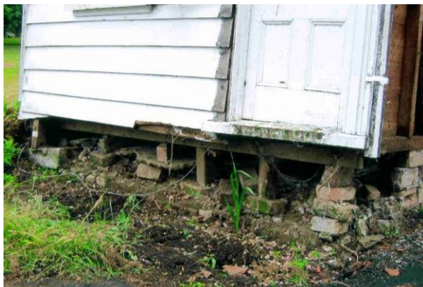
Figure 34. Base of cottage showing foundations (left: eastern end; right: north-east side)
