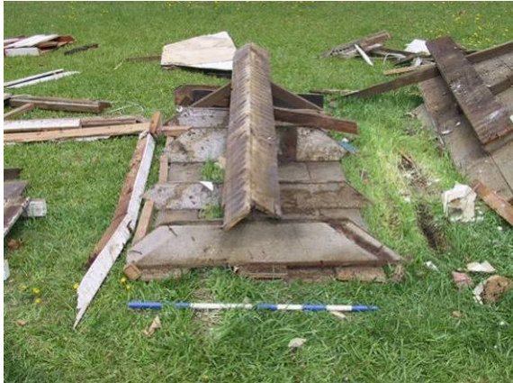
Figure 35. View of main ridge line of eastern end of cottage after demolition
