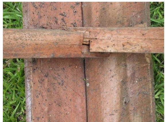
Figure 40. Ceiling bracing joint in cottage
