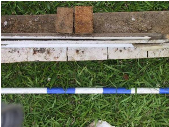
Figure 41. Join between wall and panelling in cottage
