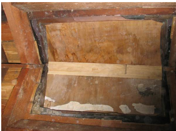
Figure 23. View of boarded up chimney hole in roof above kitchen
