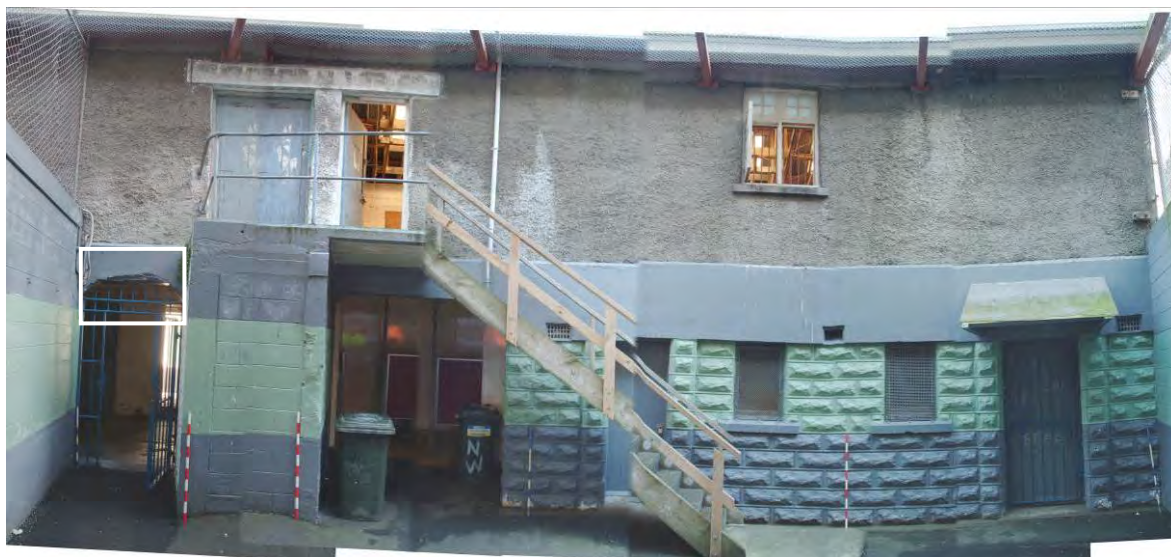
East, showing damage to concrete to allow for metal door frame
