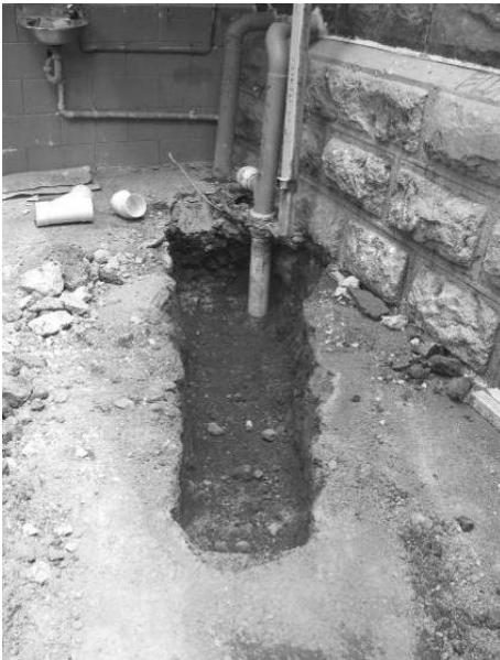
Figure 181. Drainage trench in south-west corner of exercise yard (left). Showing the exposed courses of stone in western side of trench (right)
