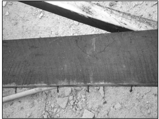
Figure 112. Circular saw marks on kauri floor beam
