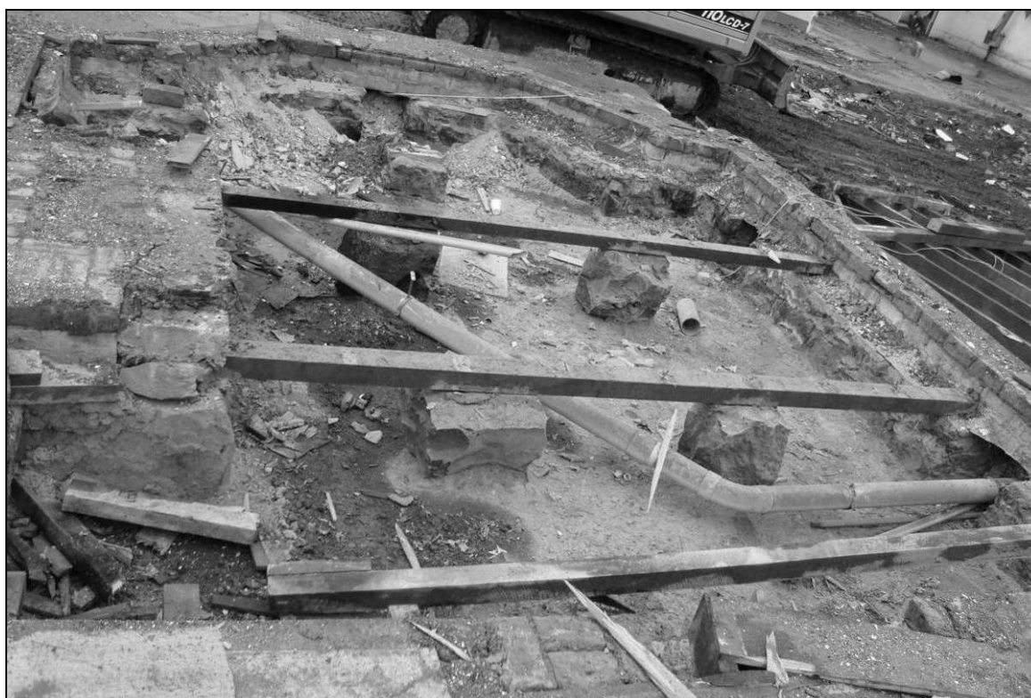
Figure 105. Basalt piles underpinning floor joists of Superintendent's House
