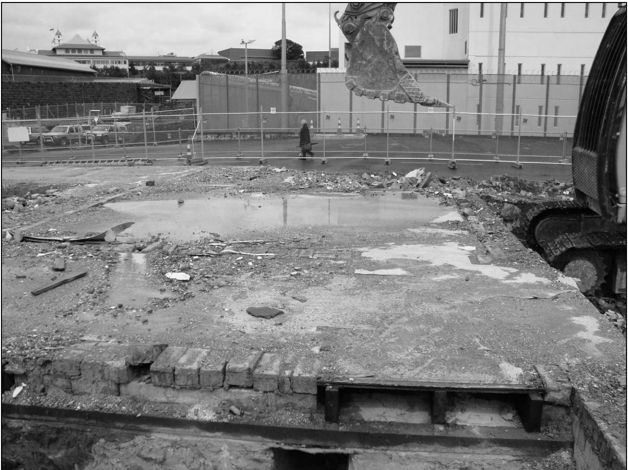
Figure 108. Metal beams in foundations of the Superintendent's House
