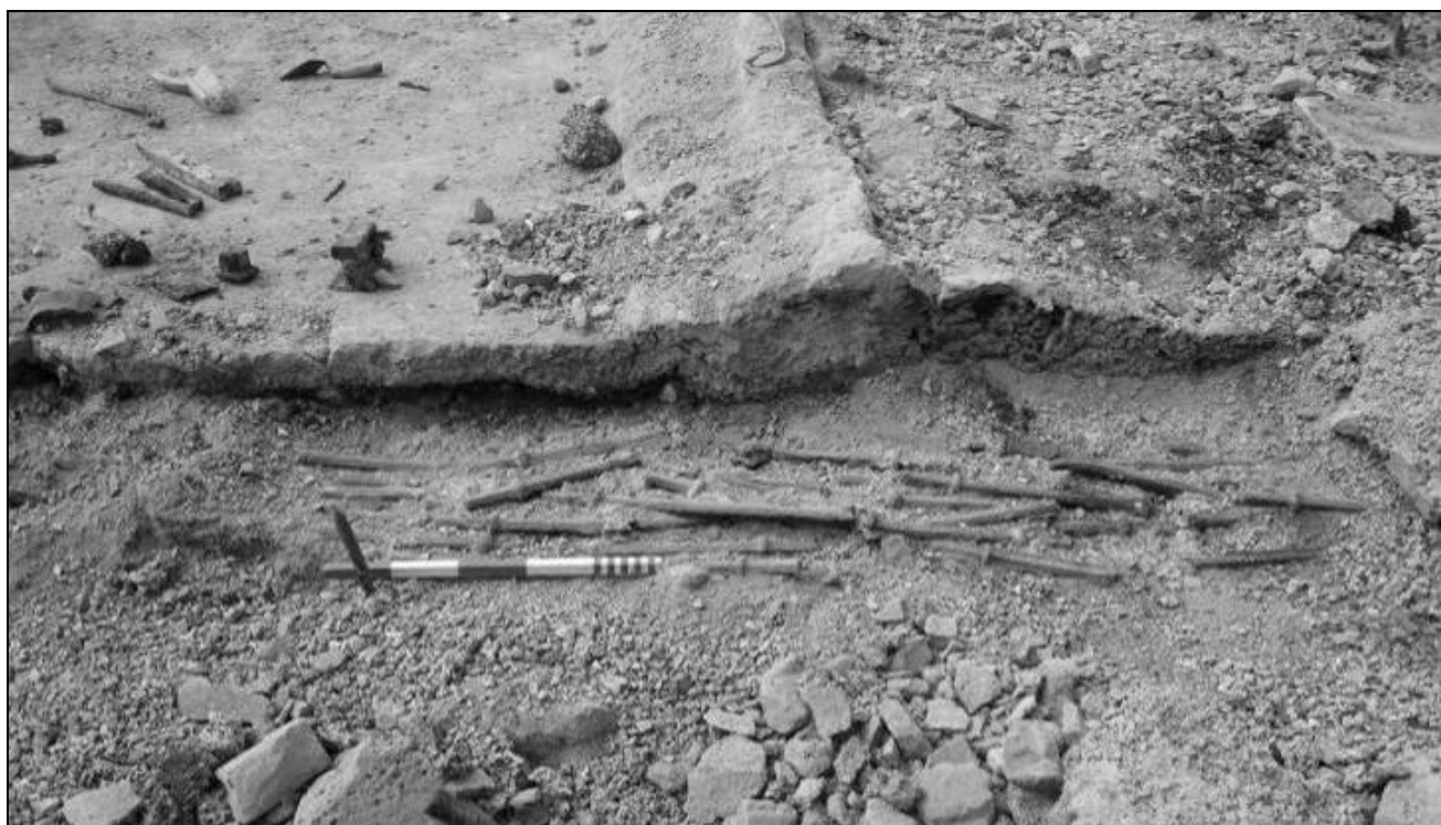
Figure 206. Drill bits laid out as steel reinforcing within the foundations of the building
