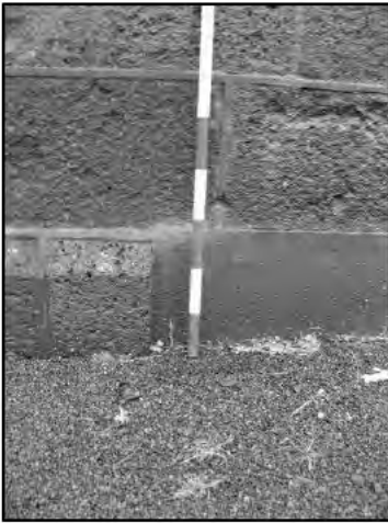
Figure 75. Basalt and concrete edging
