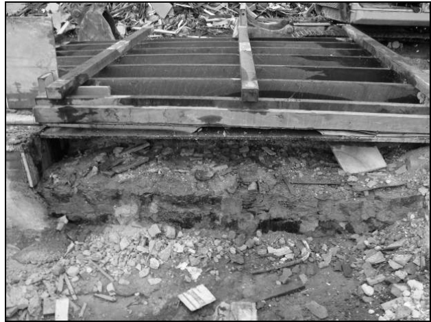
Figure 110. Wooden framing used for concrete floor below room G04 (see Figure 102)
