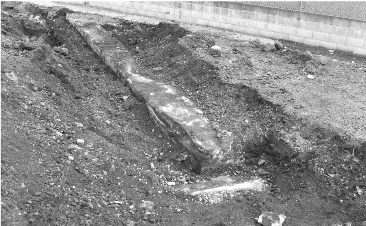
Figure 203. Old concrete wall foundation along western end of the project area
