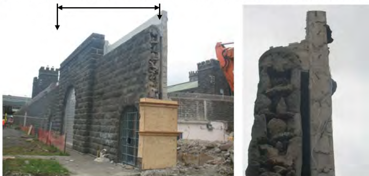
Figure 124. North Wall extension before demolition, showing thicker and narrower wall sections (left), with the wall of the Womens' Prison building behind. Close up of the internal structure of the narrow North Wall extension and Women's Prison wall (right)
