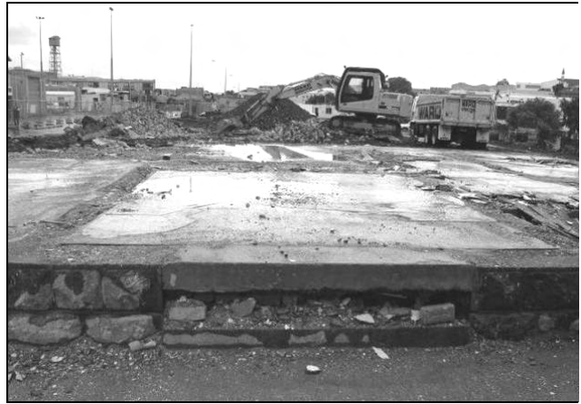
Figure 107. View of floor and foundations showing basalt and concrete
