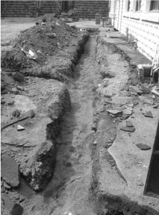
Figure 179. Looking east along the main drainage trench with branches running to the north and to the south-west (bottom right)
