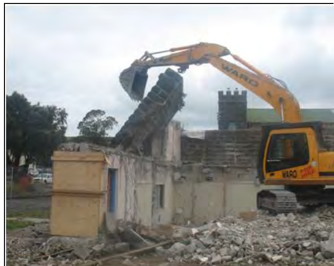
Junction on left, with demolition of the thicker wall extension in one piece on right
