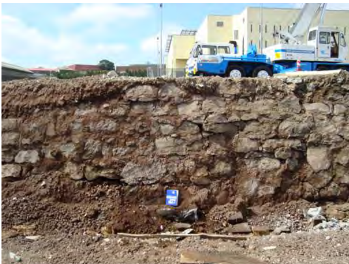
Figure 135. Close up showing irregular sized cut stone, and concrete kerb surround
