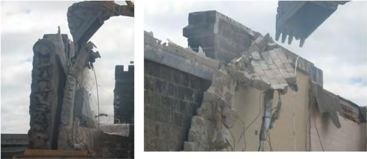
Figure 125. First stages of demolition of the concrete block Women's Prison wall
