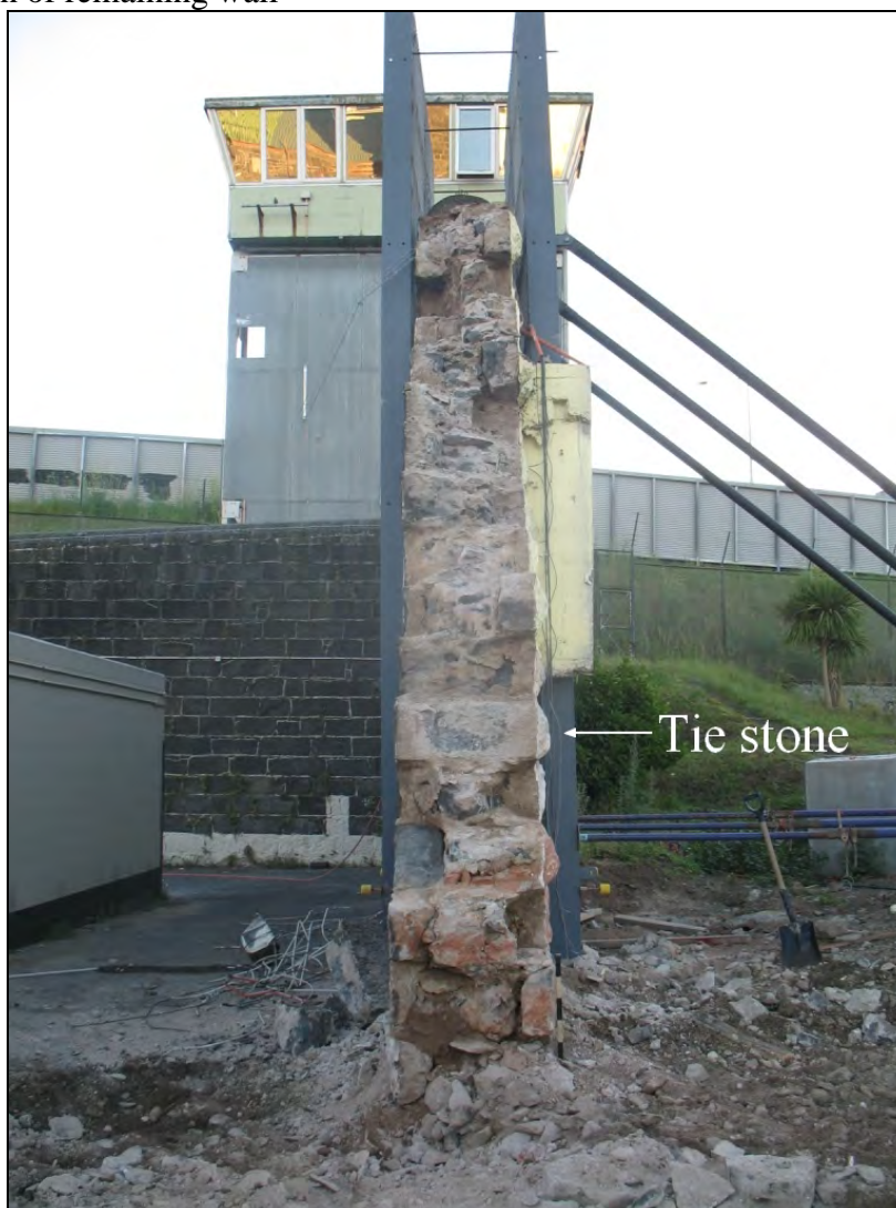
Figure 144. Cross-section of the South (heritage) Wall. Note the tapering on the exterior face of the wall (to right)
