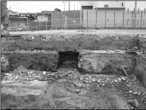
Figure 106. Close-up of wall on the basalt foundation on north side of Superintendent's House
