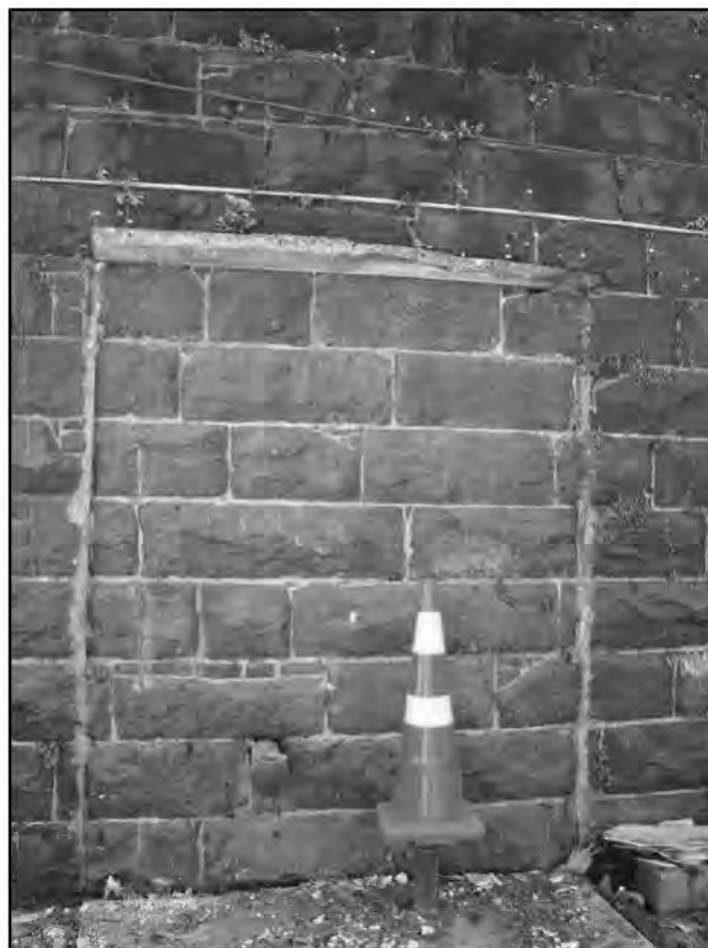
Figure 149. In-filled old entrance in eastern end of South Wall
