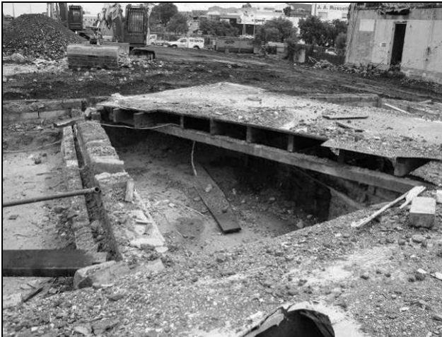
Figure 111. View of framed joists on floor beams (part intact)
