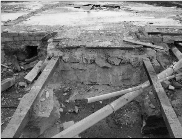
Figure 109. Wooden floor beams on basalt piles with concrete and basalt
