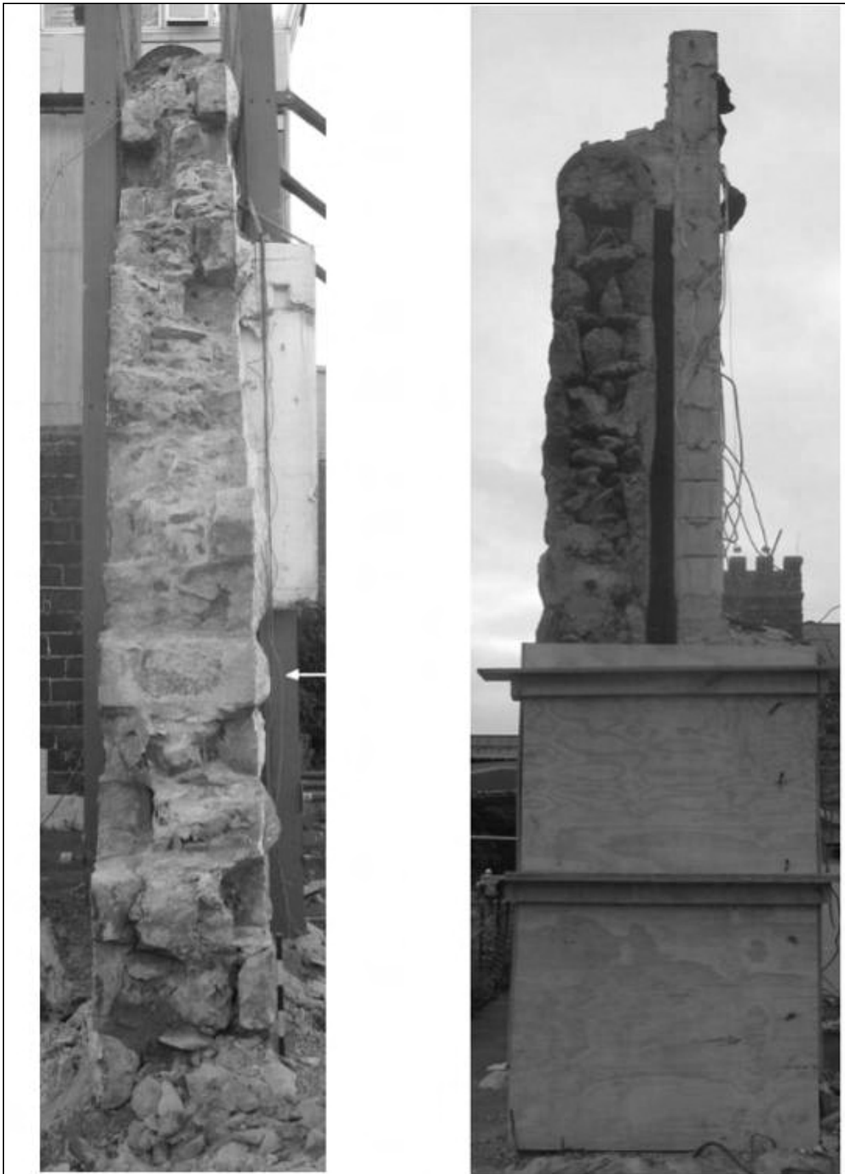
Figure 151. Comparative cross-sections of South Wall (left) and North Wall extension (right)
