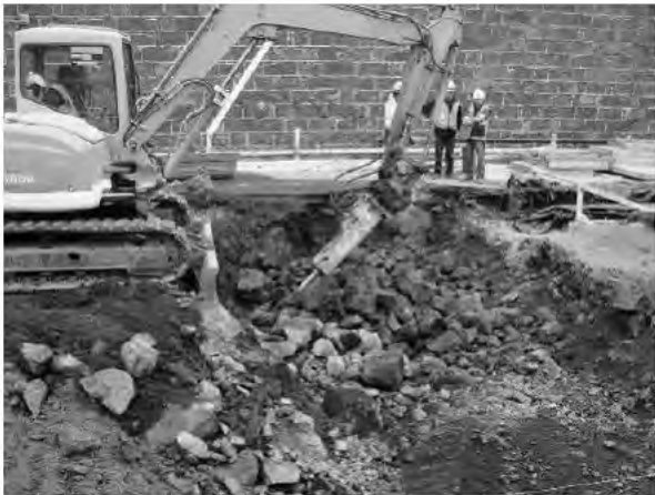
Figure 186. Rock breaking while digging out main utility trench
