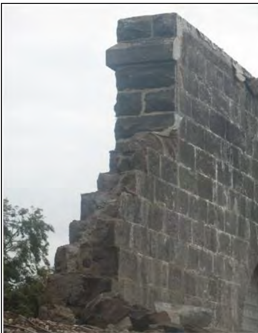
Figure 127. Junction between the thicker and narrower sections of the North Wall extension
