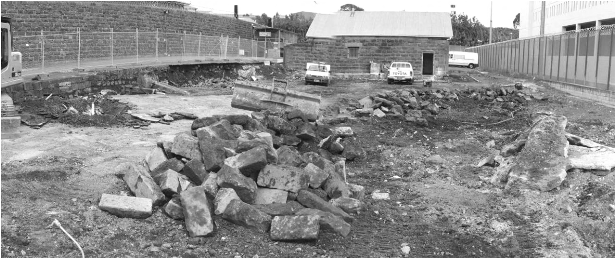
Figure 202. View of area north of Generator Shed showing removal of basalt paving
