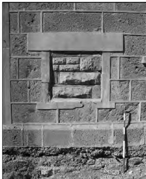
Figure 78. View of filled aperture in Generator Shed
