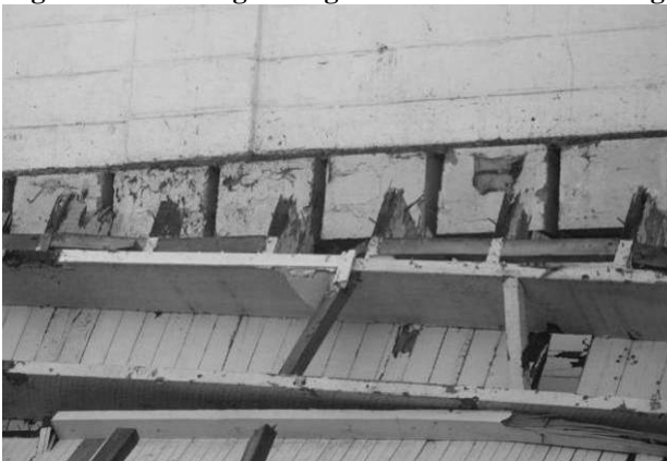
Figure 47. Detail of the construction methods used in securing the first floor to the wall of the building
