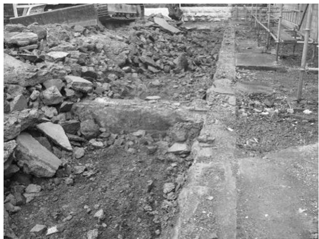
Figure 50. Hard fill beneath the concrete floor and wall located halfway along the length of the building
