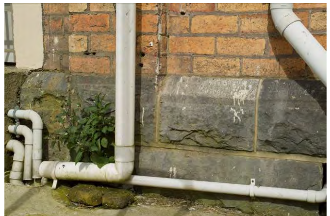
Figure 100. Basalt blocks at base of walls
