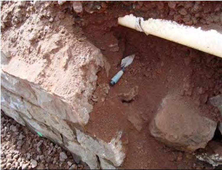
Figure 136. Showing thickness of stone blocks of wall near Superintendent's House
