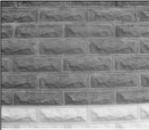
Figure 34. Moulded concrete blocks from the Bag Shop
