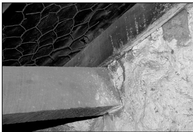
Figure 82. Roof beam mounted into basalt wall
